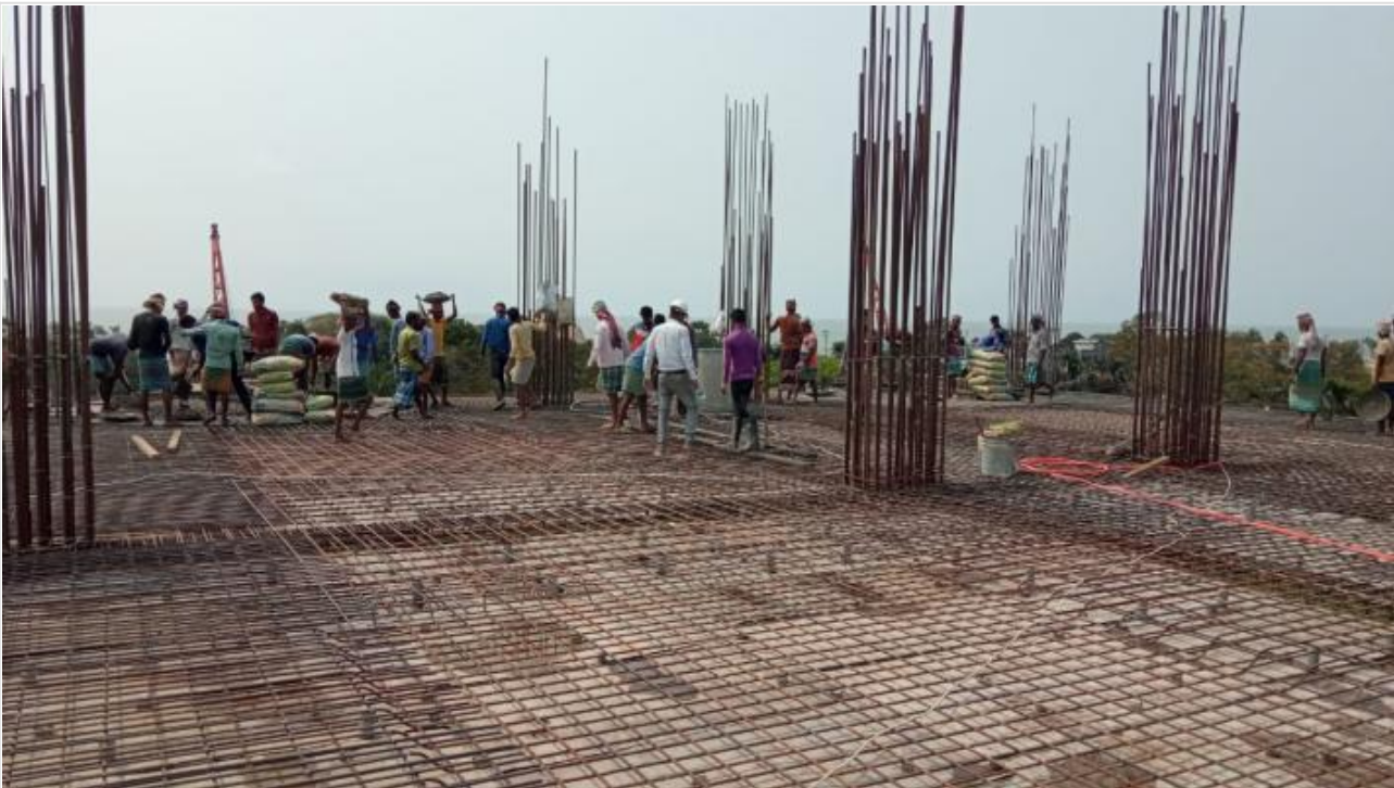
Tower-1-3rd Floor Roof Slab Concreting on 11-03-21
