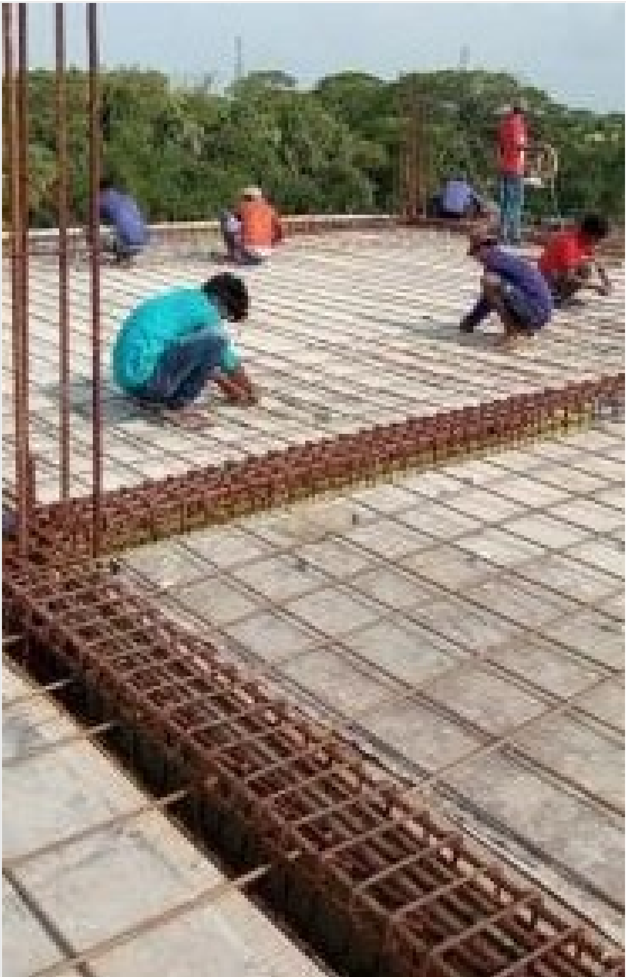
Slab Re-bar Work on 05-06-21
