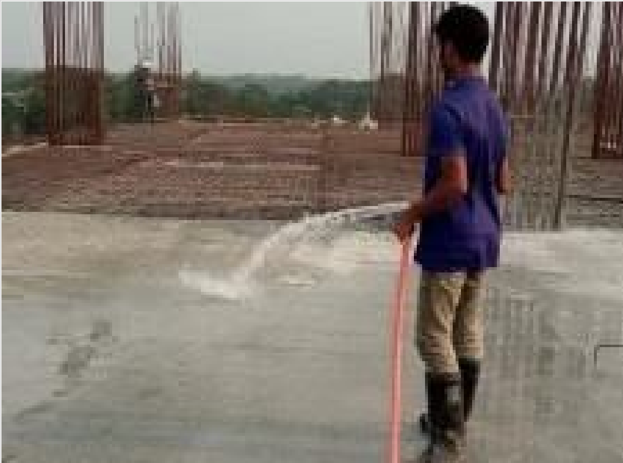
Tower-1-3rd Floor Roof Slab Curing on 31-03-21
