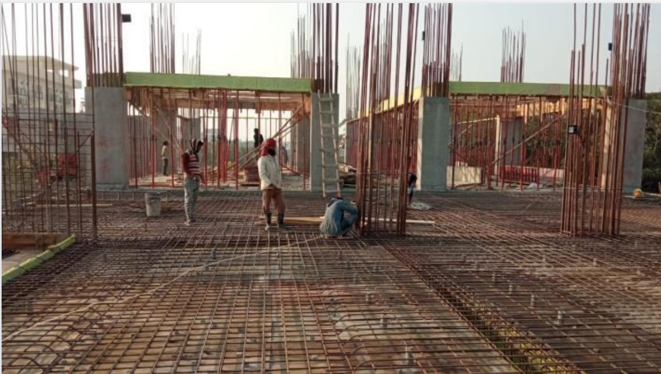
Tower-1-1st Floor Roof Slab 3600 sft Con on 05-02-21
