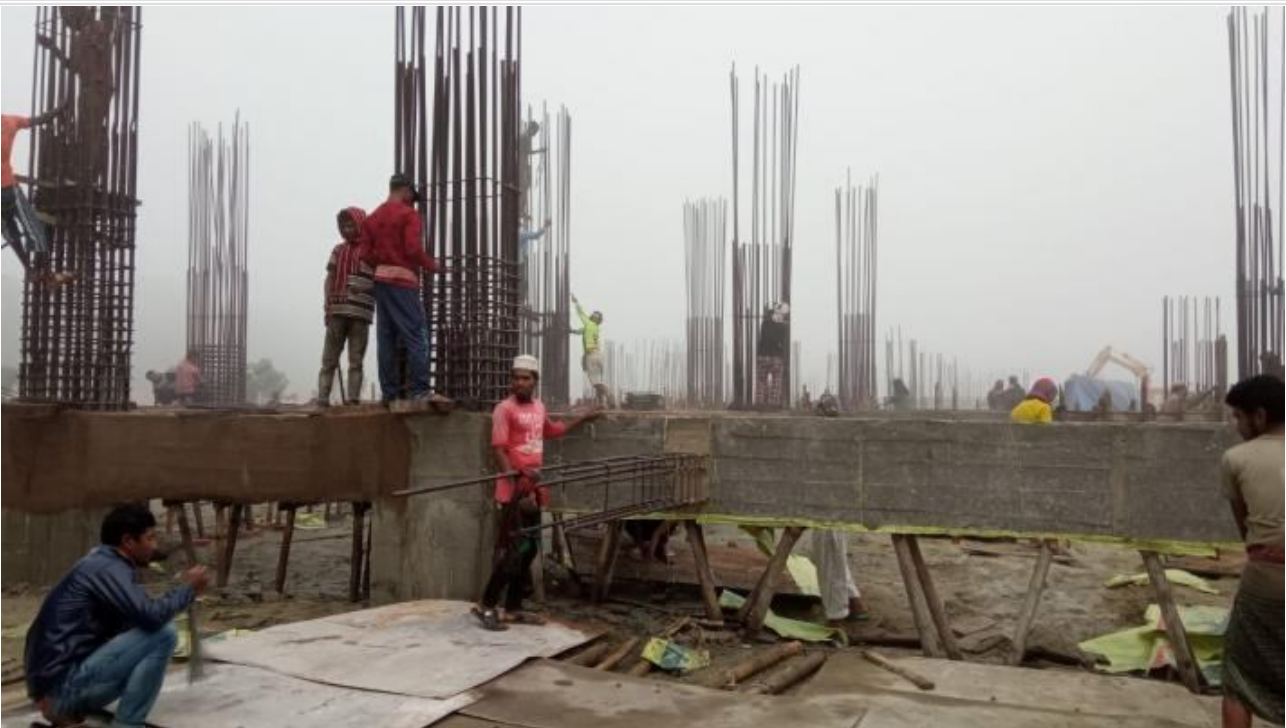
Column Work on 07-12-20
