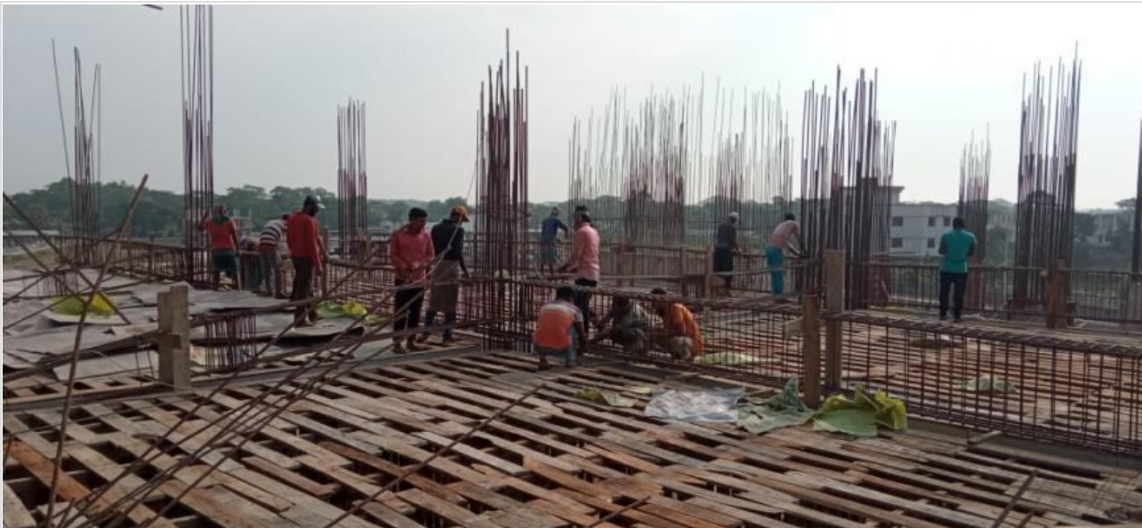
Roof Slab Shuttering on 04-05-21
