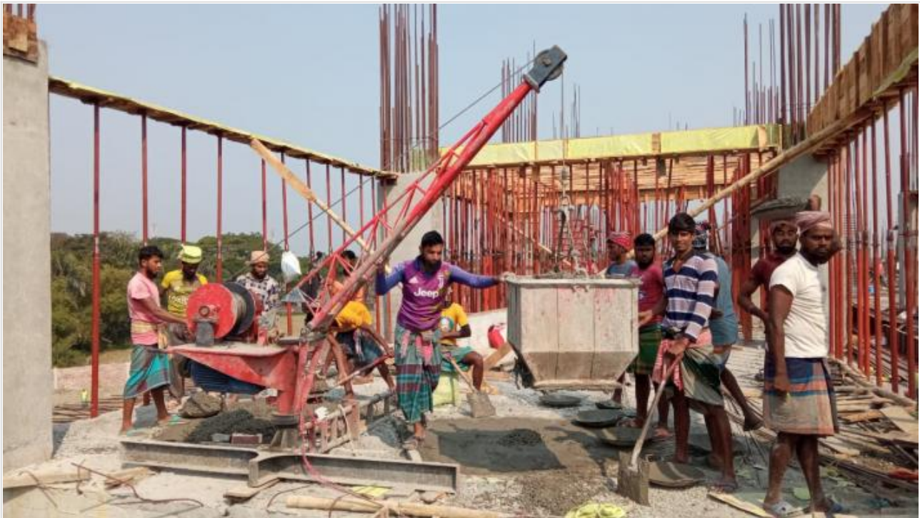
Tower-1-1st Floor Roof Slab 3600 sft Con on 07-02-21
