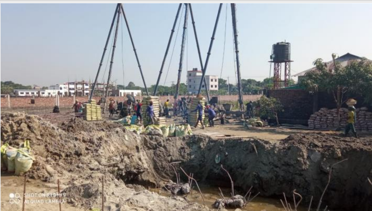
Tower-2-Piling Work on 28-11-20
