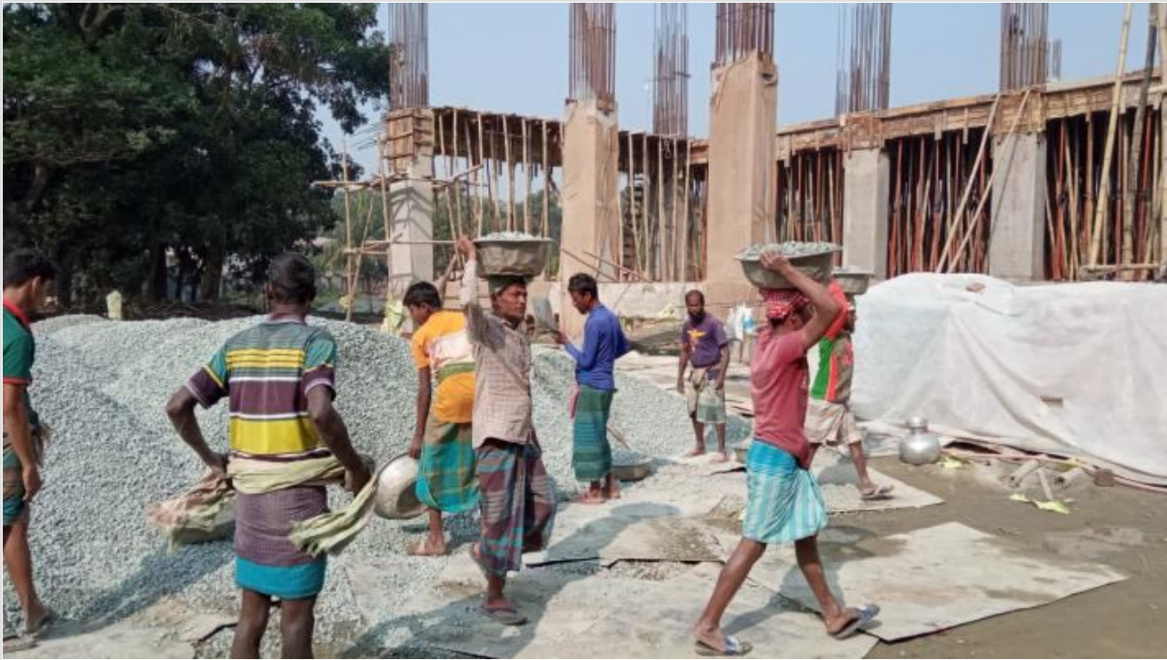
Tower-1-GF Roof Slab Concreting on 21-12-20
