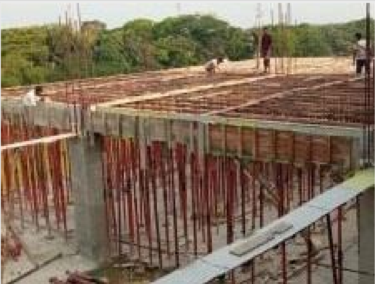
Beam Shuttering Work on 29-04-21
