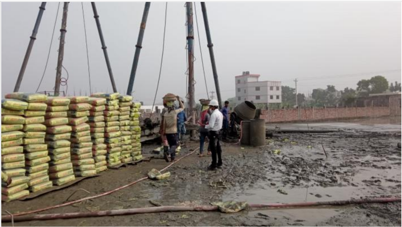
Tower-2-Pile Work on 09-12-20
