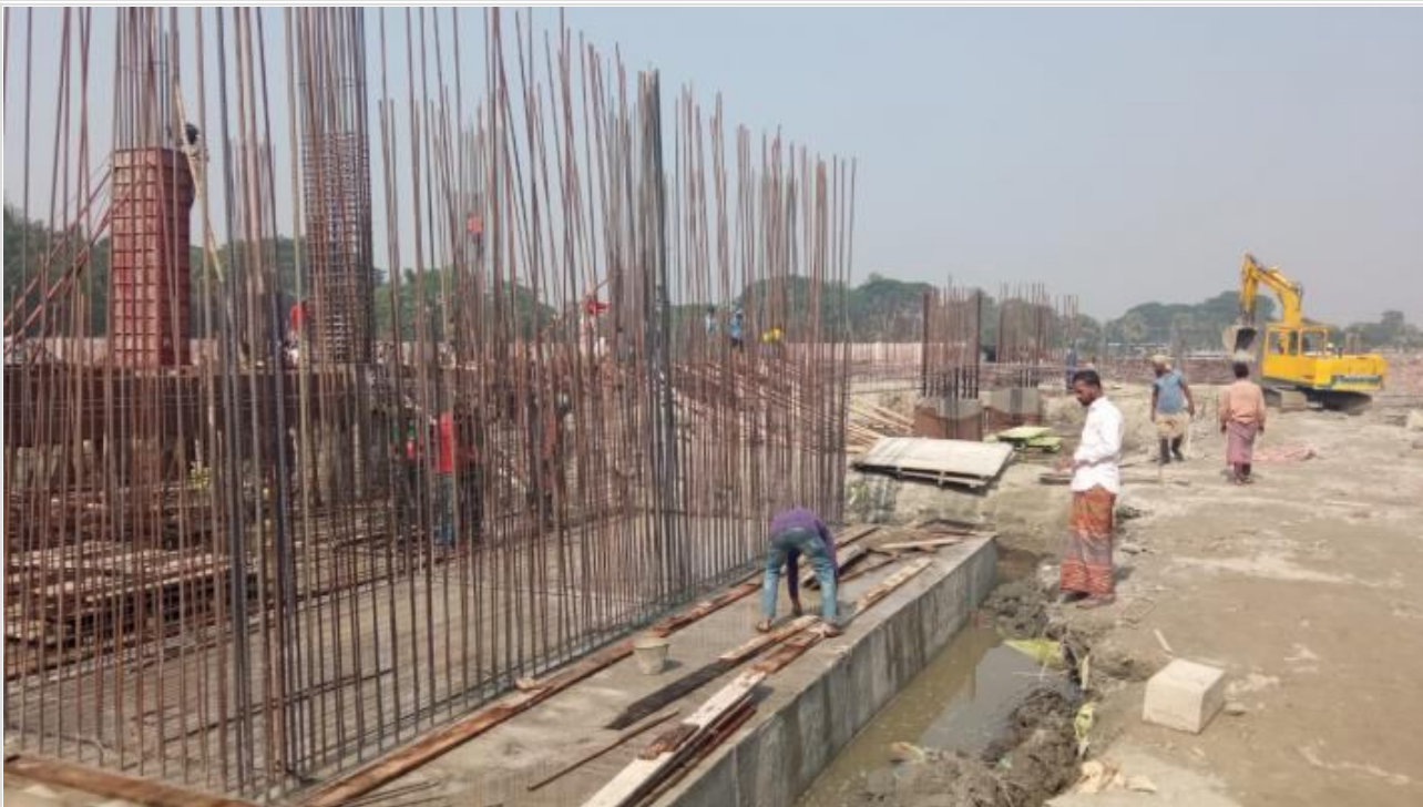
Tower-1-Lift Core Re-bar Work on 20-12-20
