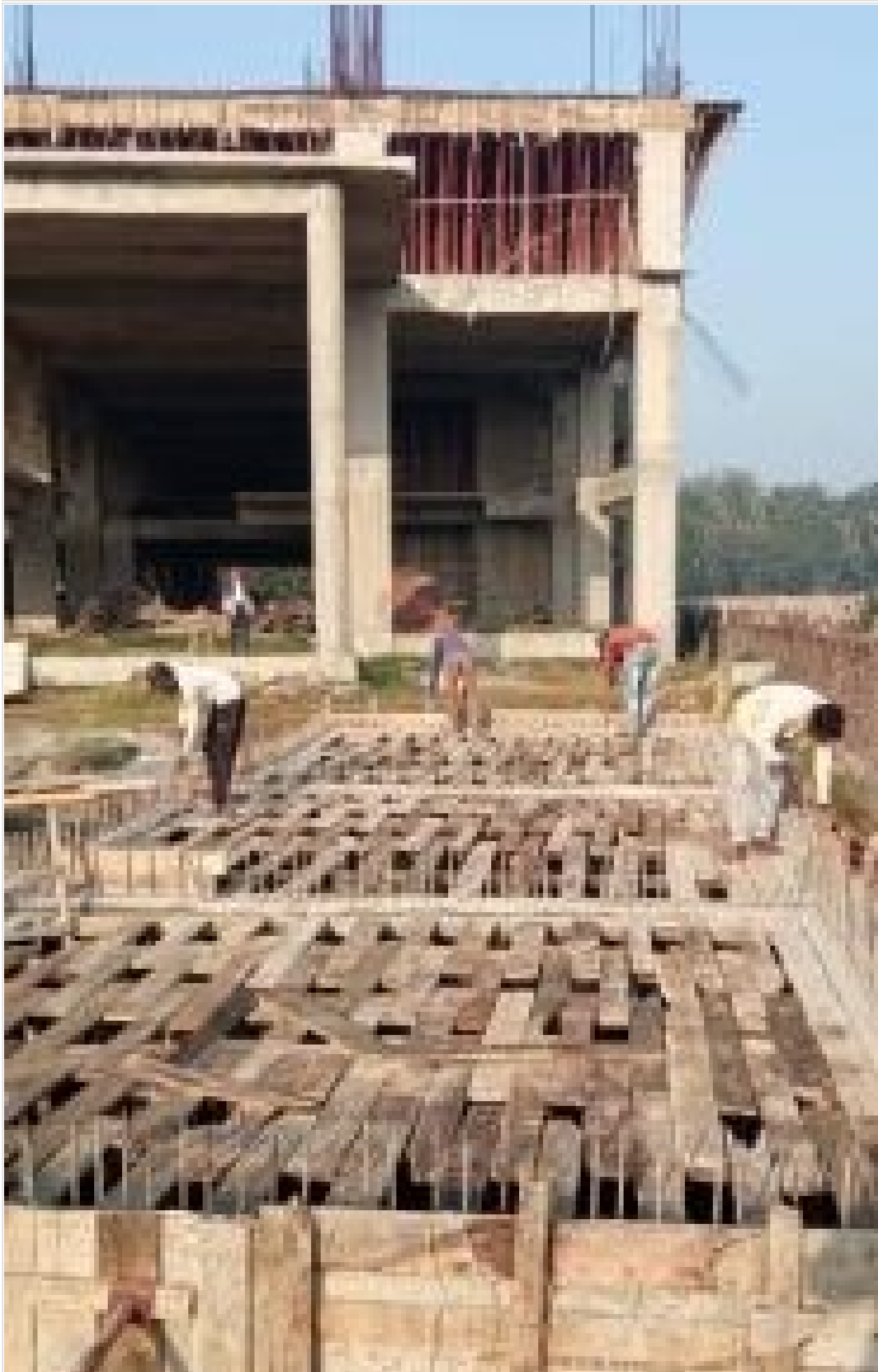
East Septic Tank Slab Shuttering on 10-02-22
