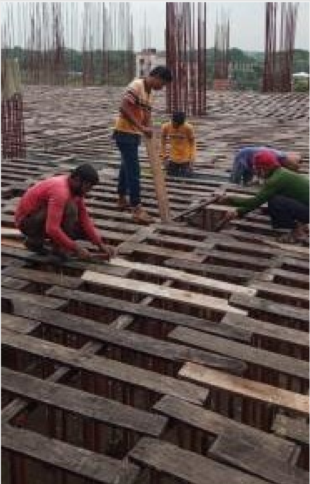
Tower-2-3rd Floor Slab Shutter Repairing on 28-10-21
