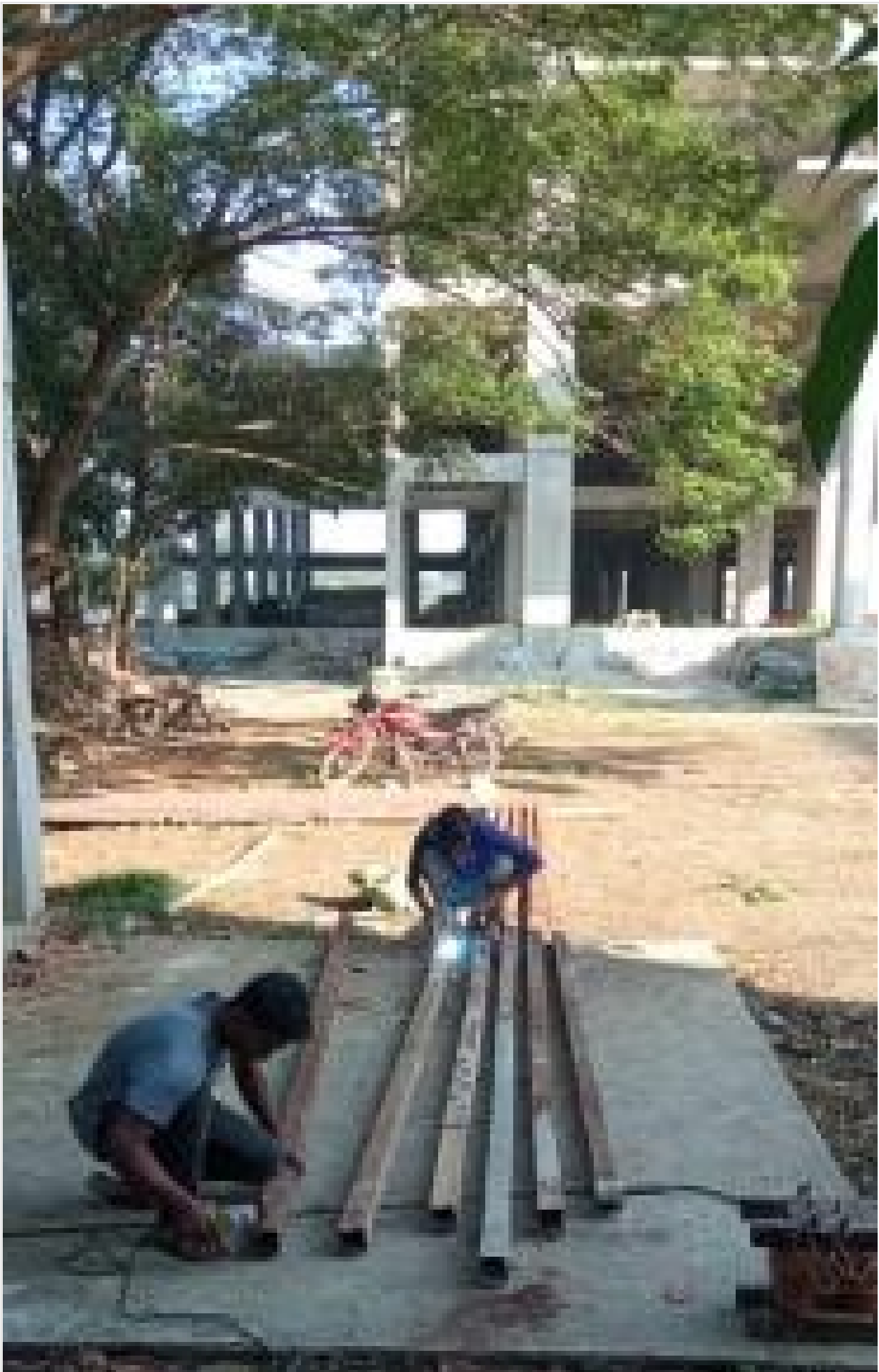
Hollow box jointing for slab shuttering on 30-11-21
