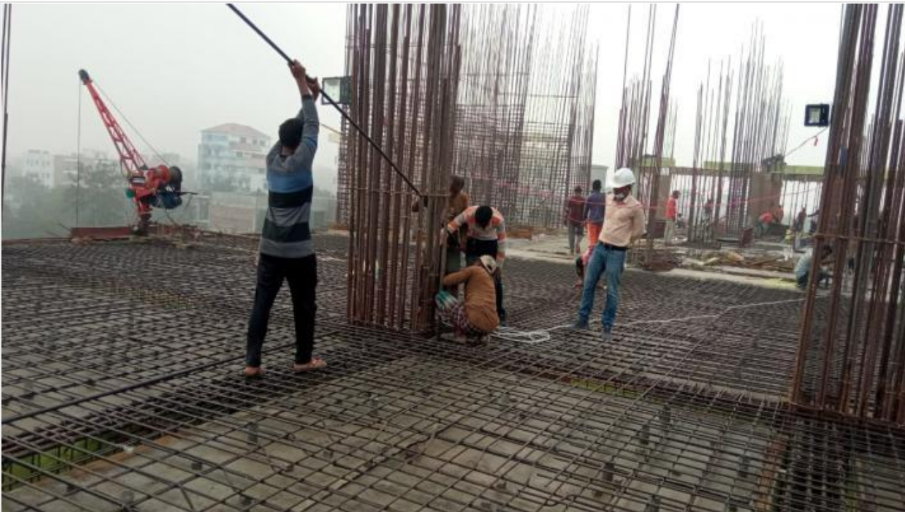
Tower-1-2nd Floor Roof Inspection on 25-02-21
