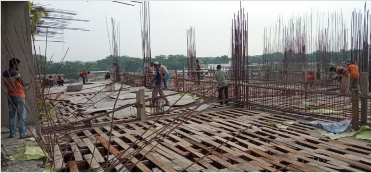
Roof Slab Shuttering on 04-05-21
