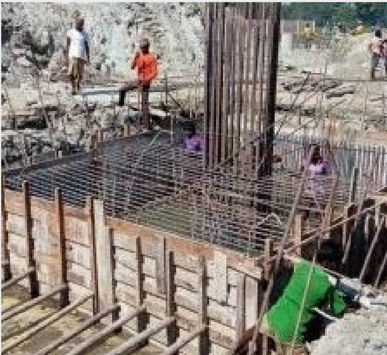
Tower-1 Pile Cap on 12-11-20
