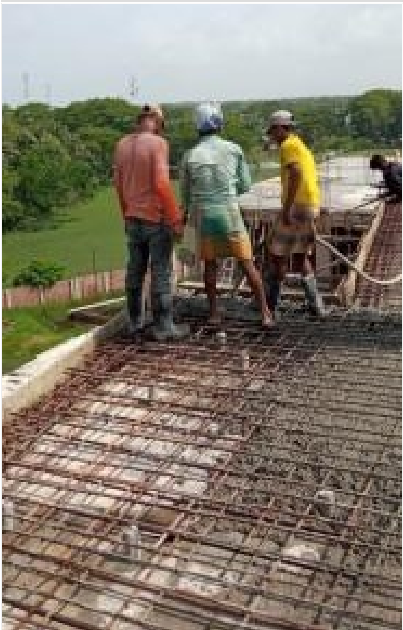
Tower-1-4th Floor Concreting on 26-06-21
