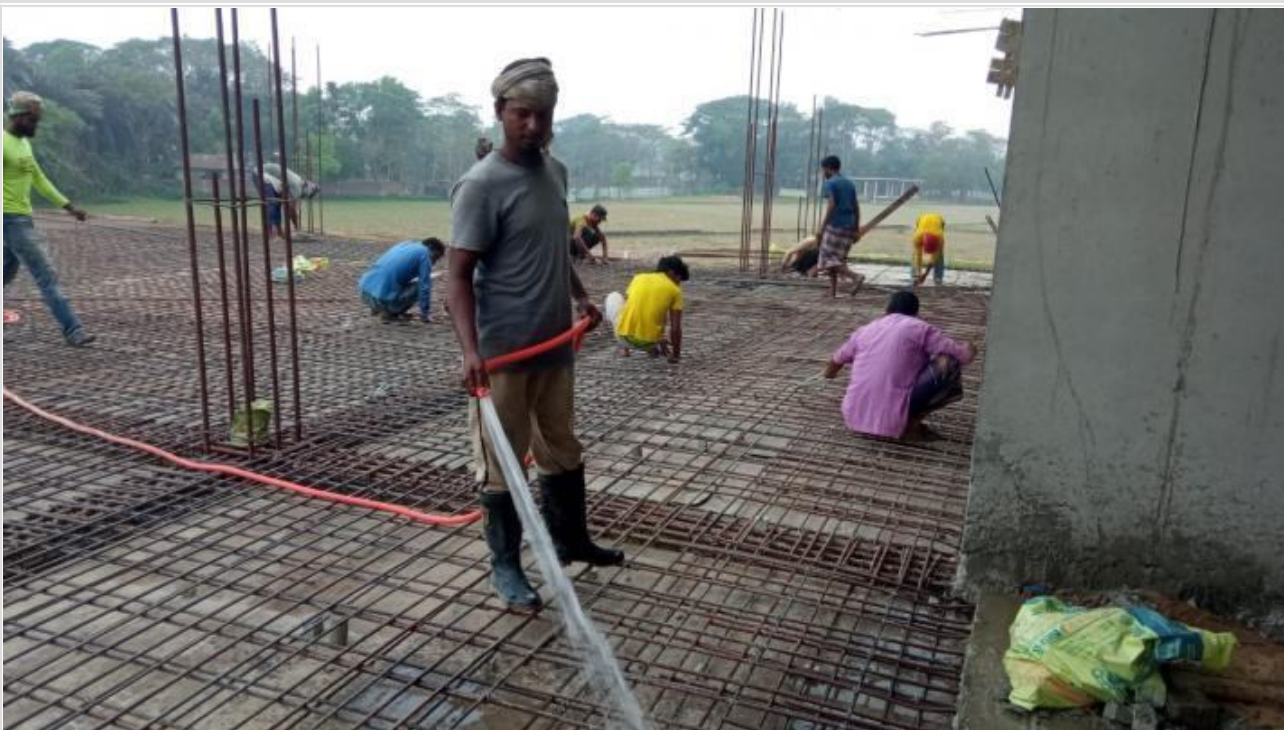
Restaurant-Double Height Slab Concreting on 02-03-21
