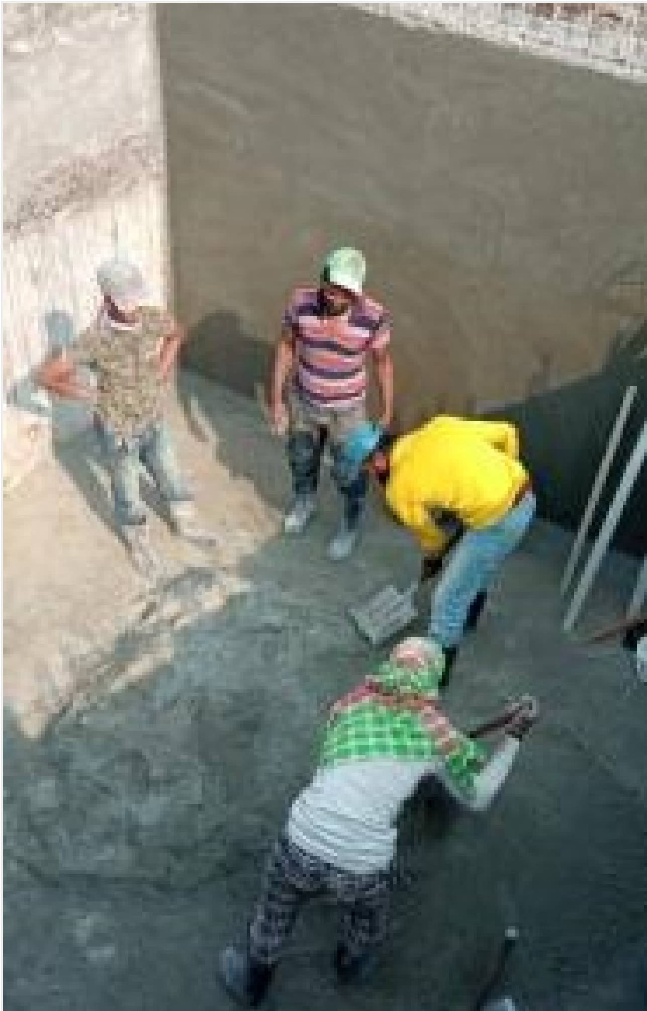
East Septic Tank Plastering on 01-02-22
