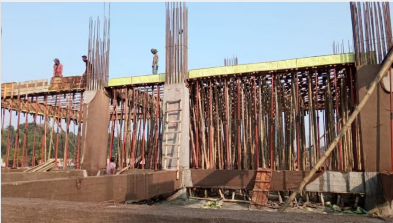
Tower-1-GF Beam Shuttering on 18-12-20
