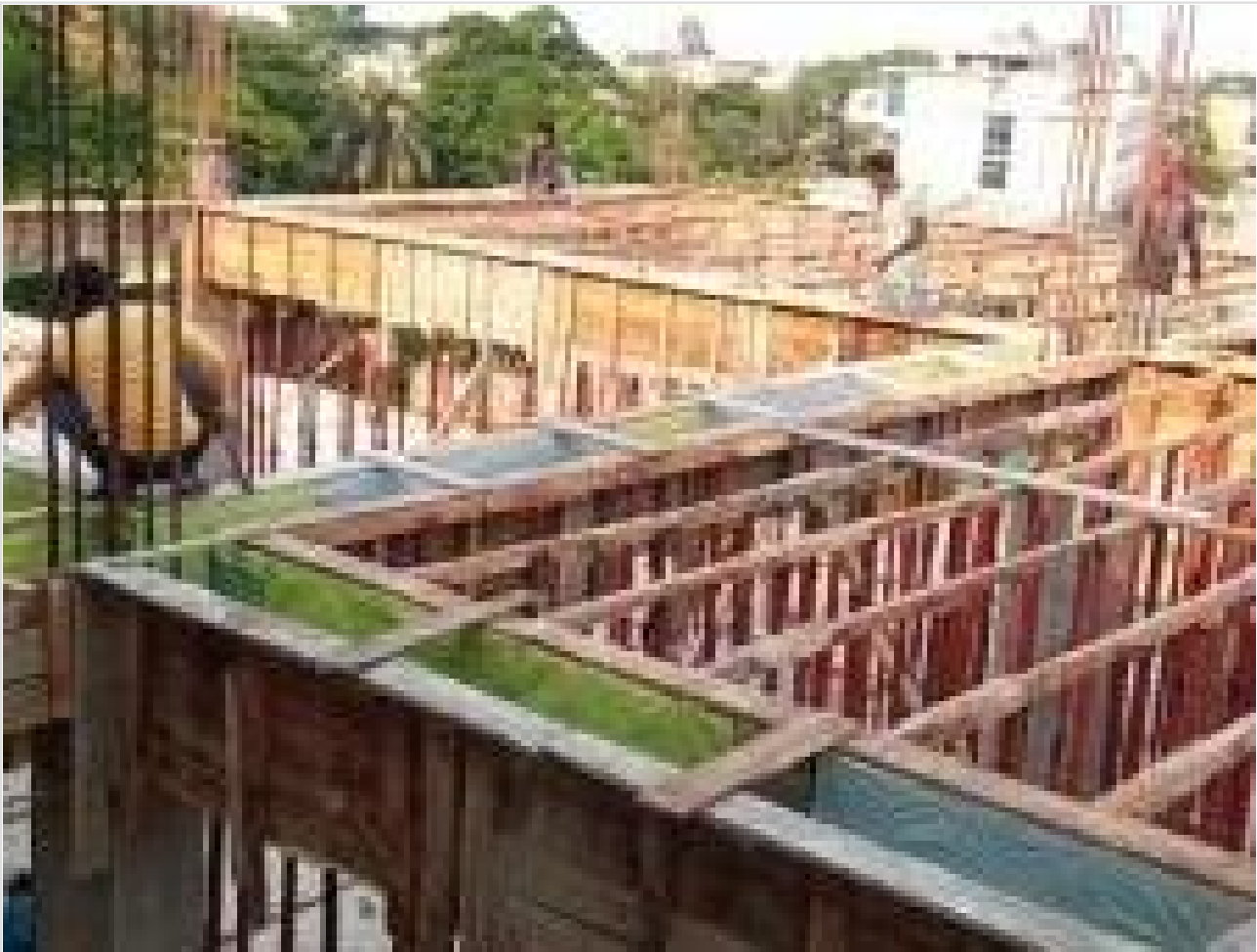
Beam Shuttering on 29-04-21
