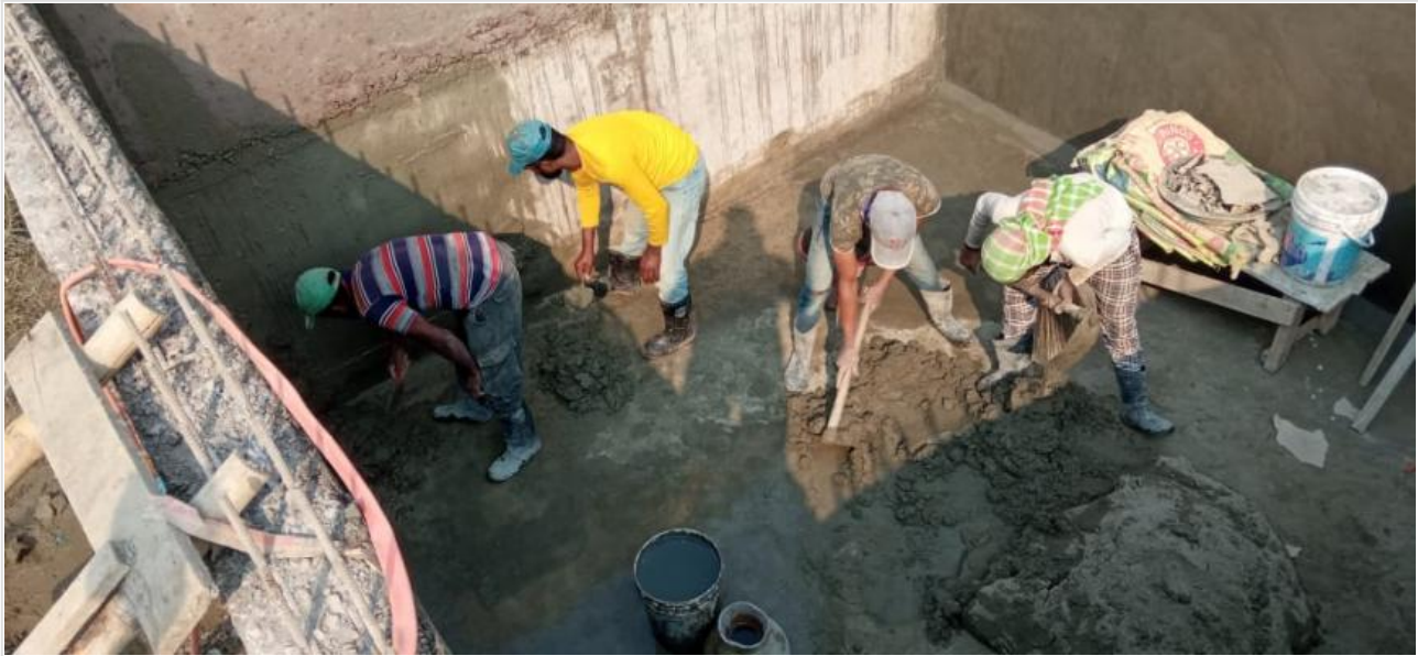
East Septic Tank Plastering on 01-02-22
