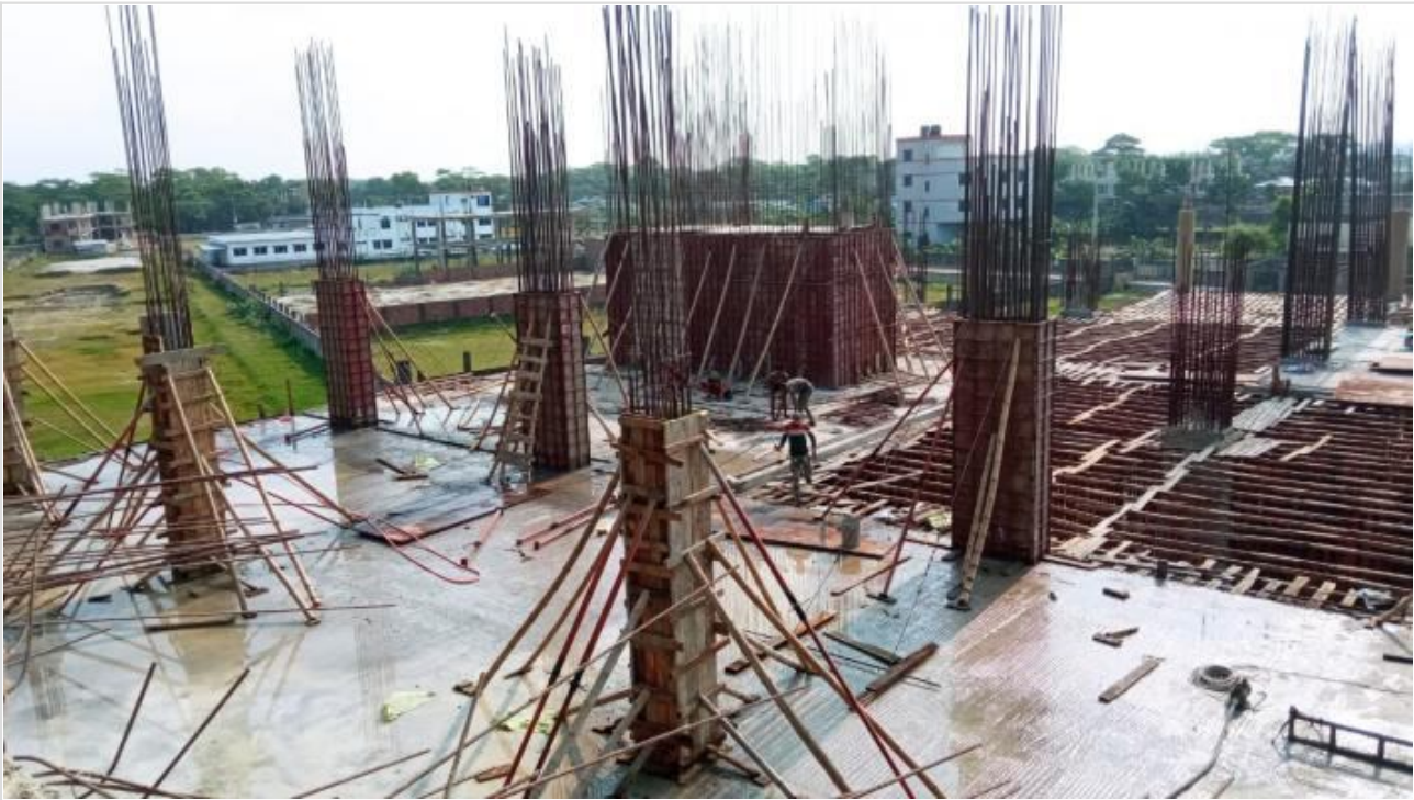
Column Concreting on 28-04-21
