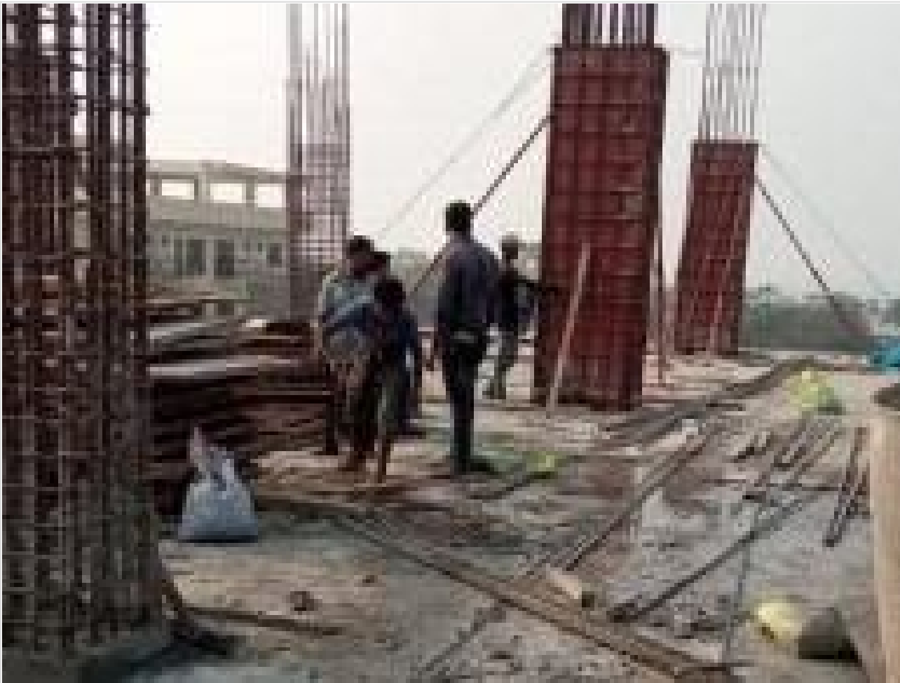
Column Shuttering Work on 25-03-21
