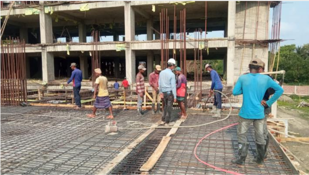
Tower-1-GF Roof Slab(G-I/6-7a)Concreting on 19-04-21
