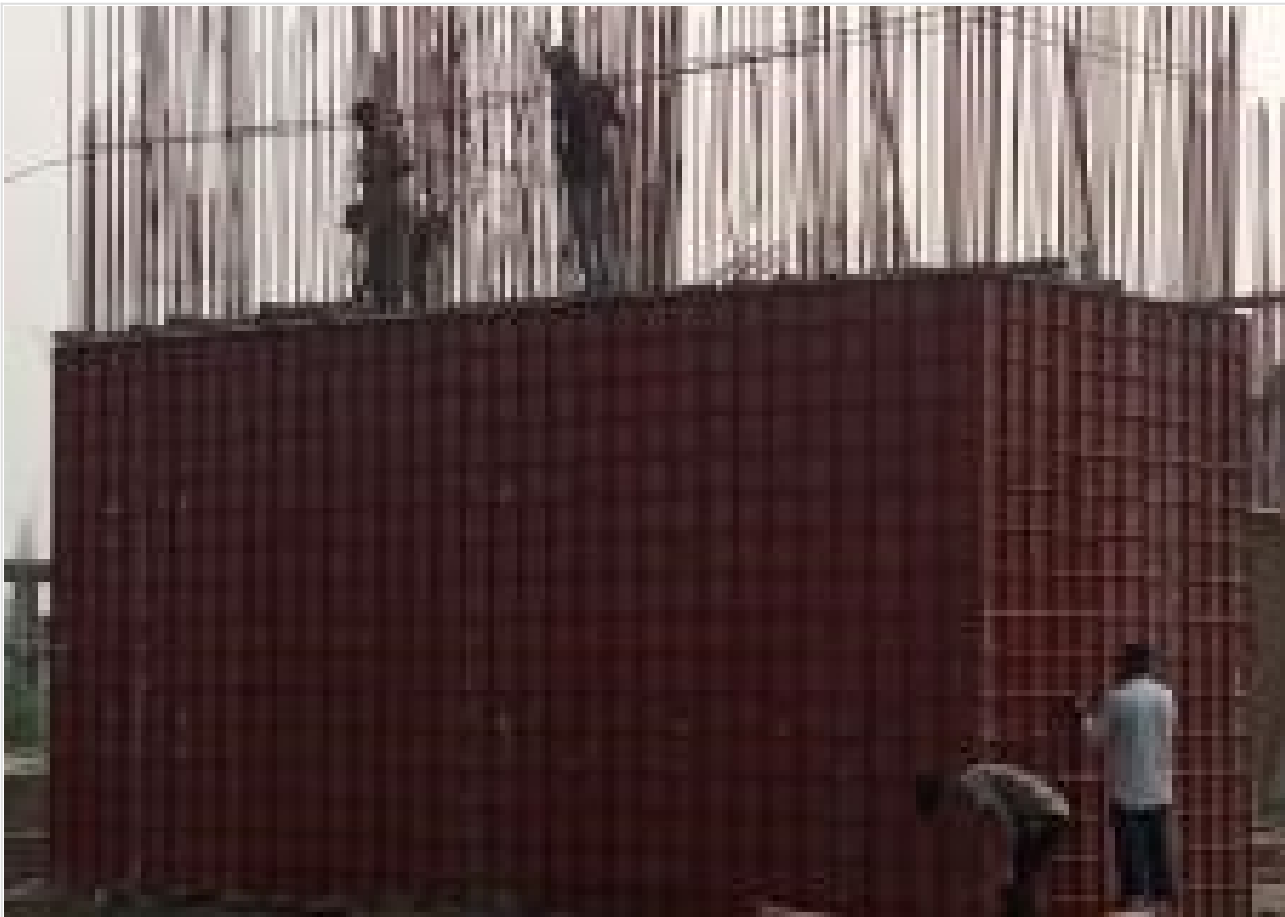
Lift Core Wall Shuttering on 24-03-21
