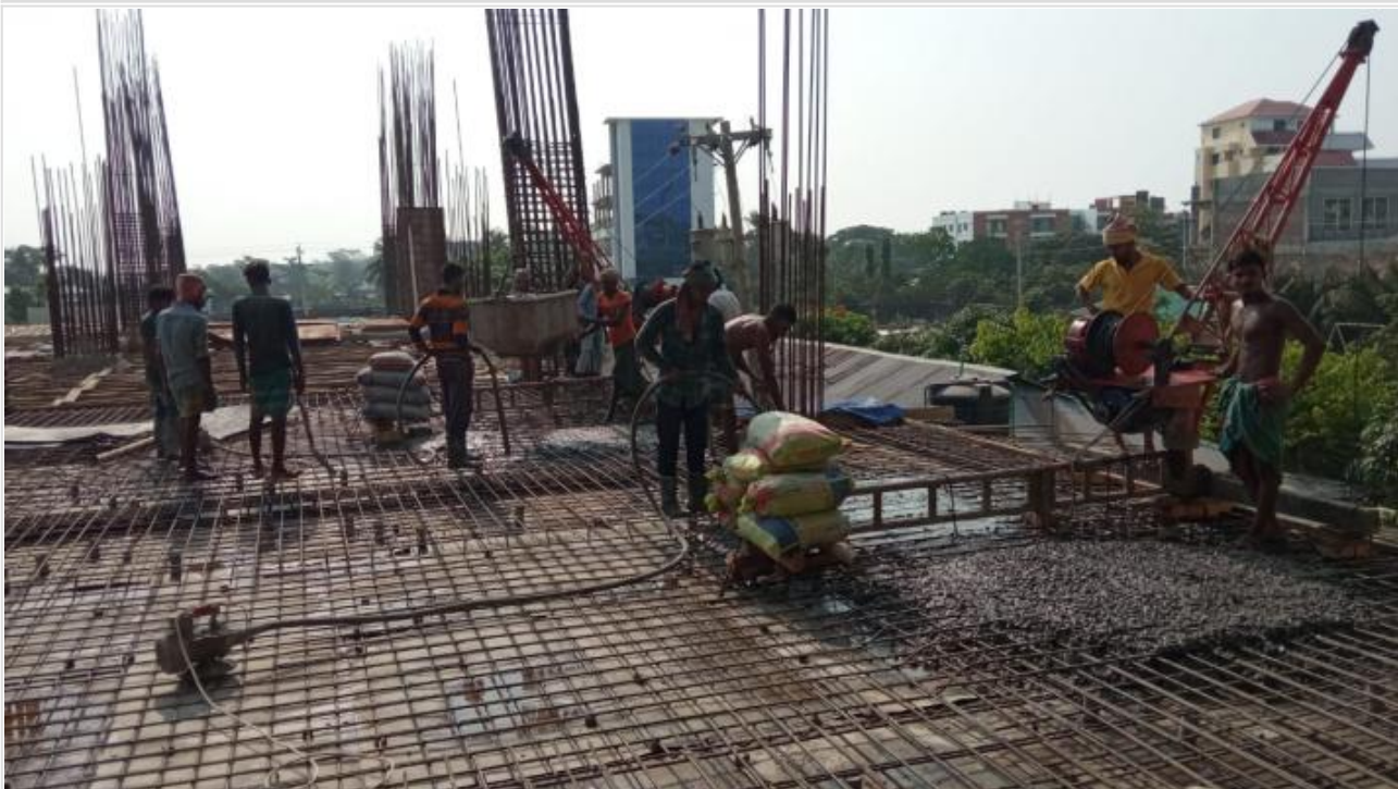
Between Tower1-2-GF Roof Slab-Concreting on 26-04-21
