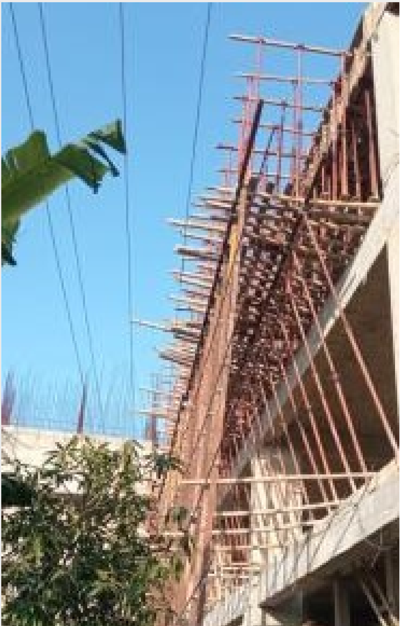
Tower-2-3rd Floor Slab Shuttering on 30-11-21
