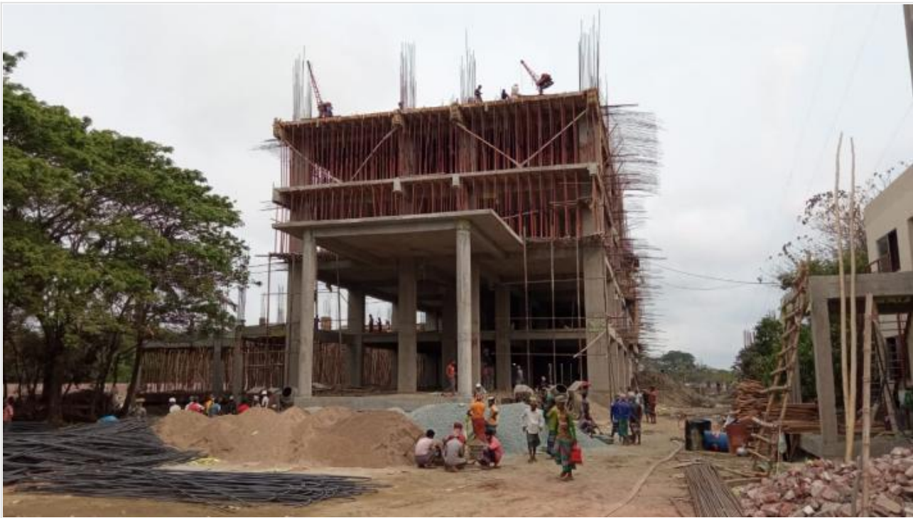
View From South on 11-03-21
