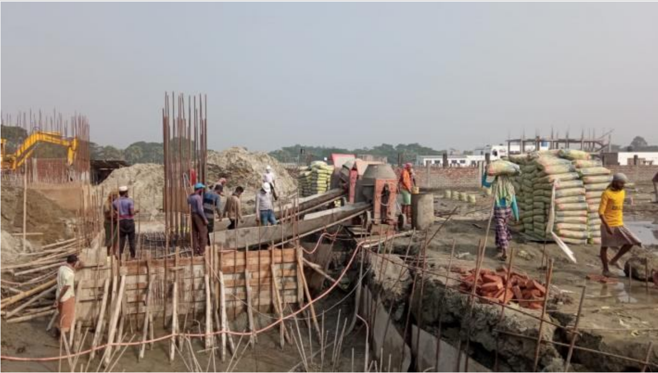
Tower-1-Pilecap Concreting on 12-12-20
