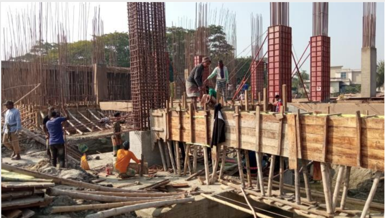
Tower-1-Grade Beam Shuttering on 24-12-20
