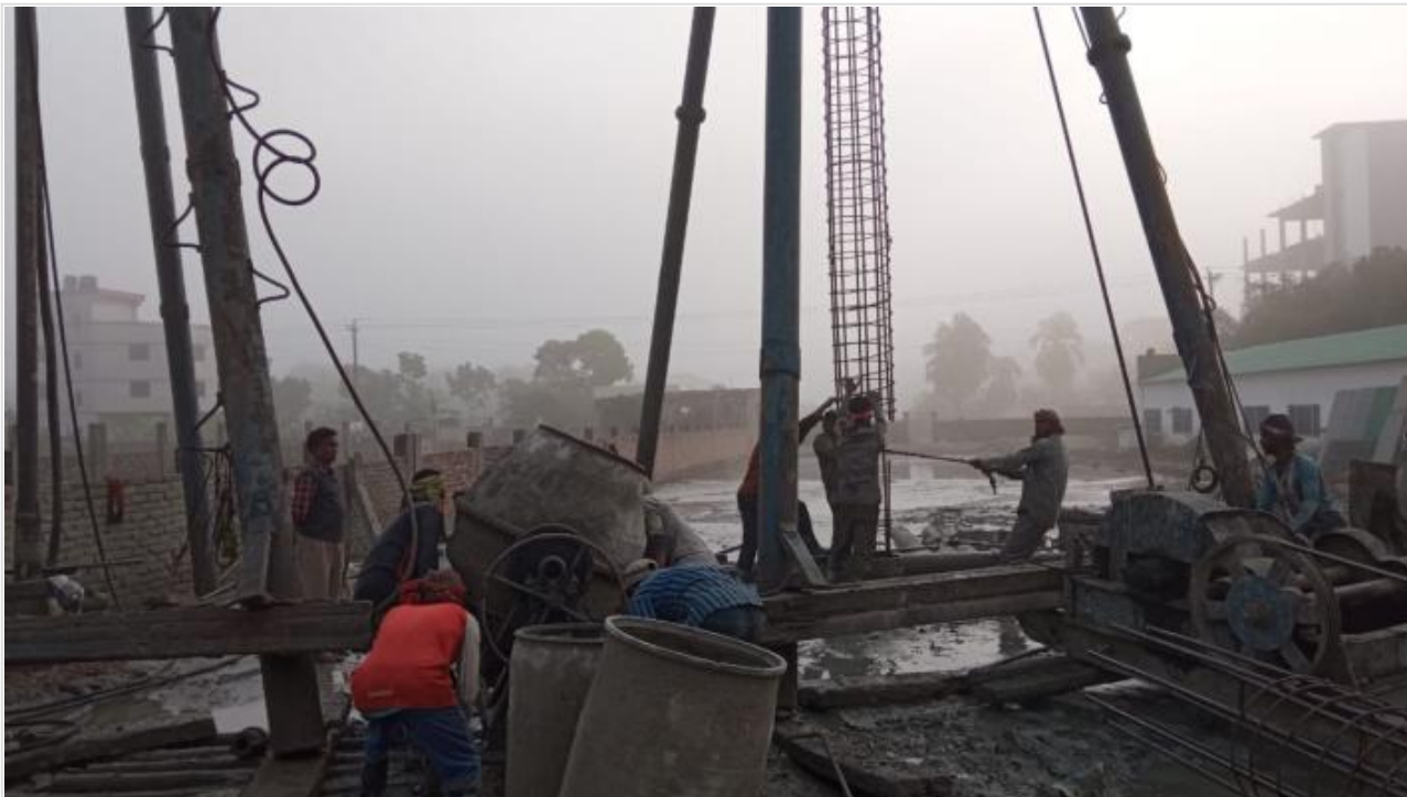
Tower-2-Pile Work on 04-12-20
