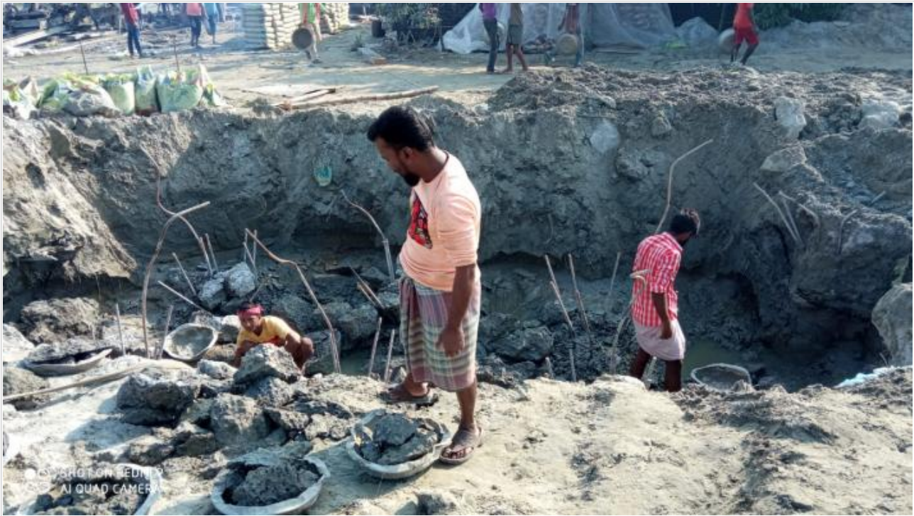
Tower-1-Pilehead breaking on 30-11-20
