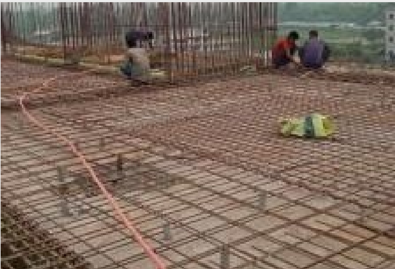
Restaurant GF Double Height Slab-6-9/A-B on 23-03-21
