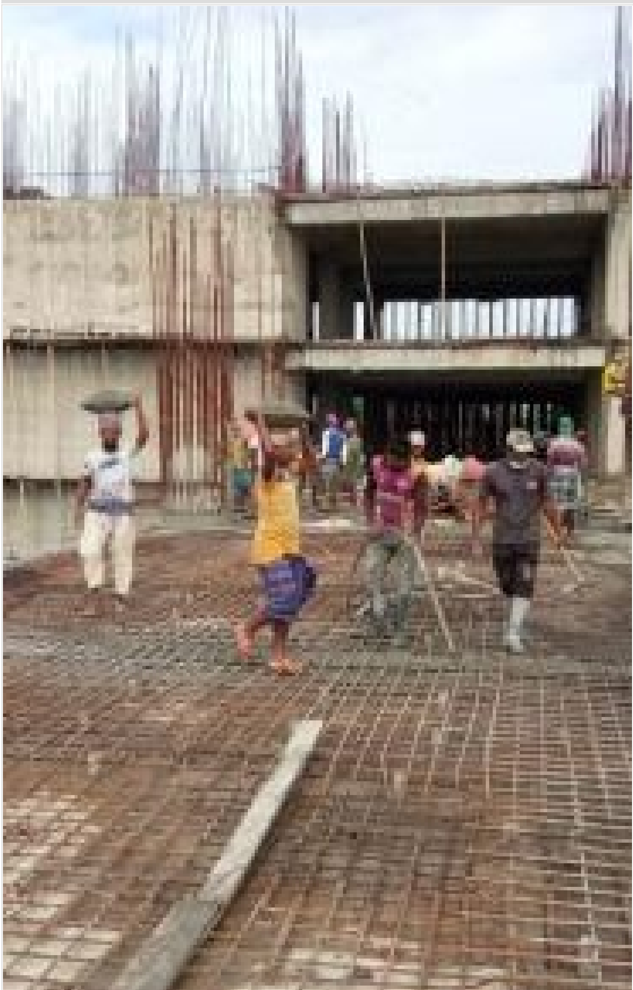
Tower-2:2nd floor slab concreting on 05-07-21
