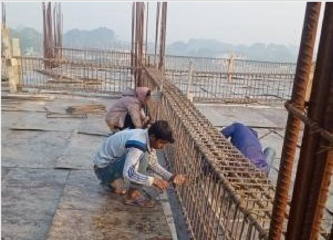
Tower-2-3rd Floor-Re-bar Work on 08-01-22
