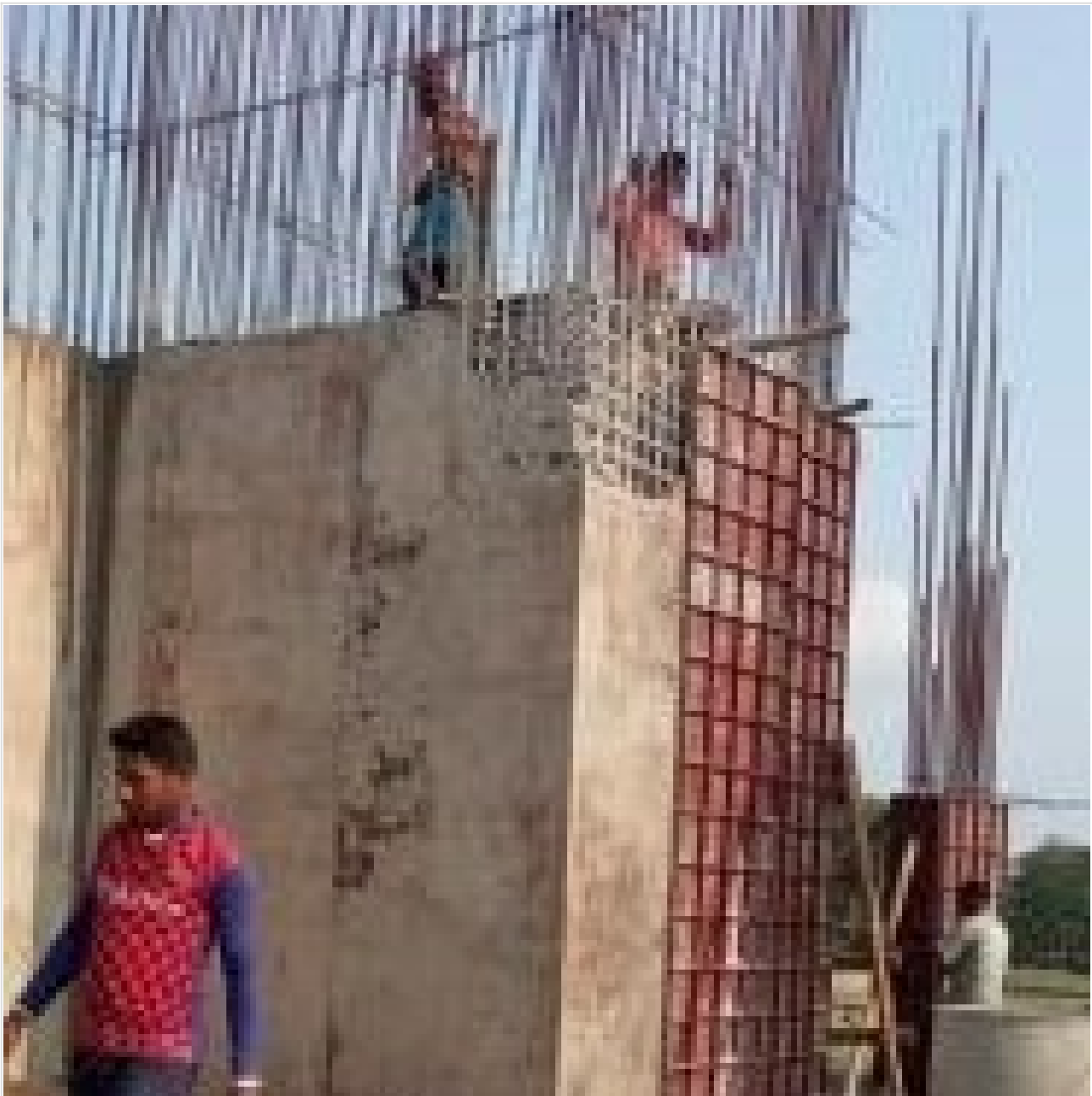
Tower-2-Lift Core Deshuttering on 02-05-21
