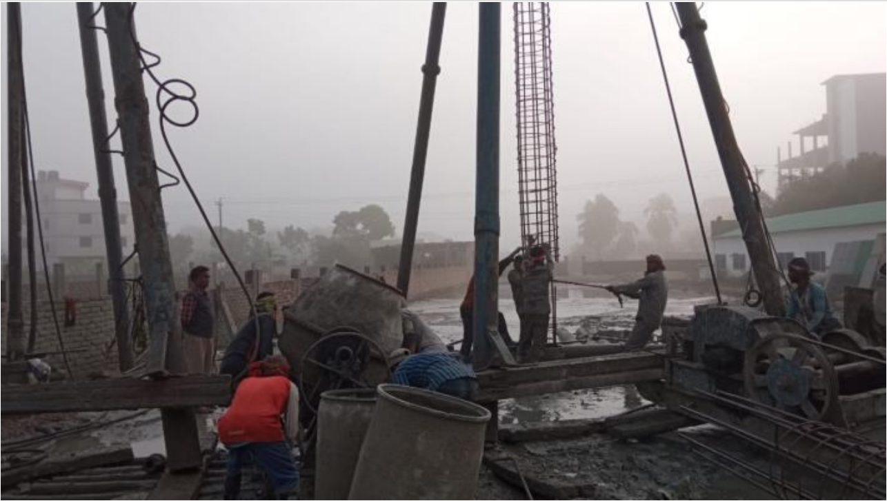
Tower-2-Pile Work on 04-12-20
