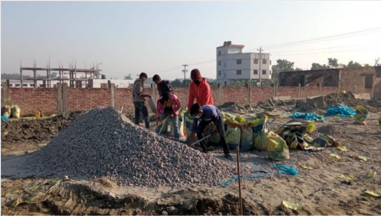
Tower-1-1st floor Roof Slab 2450sft Conc on 10-02-21
