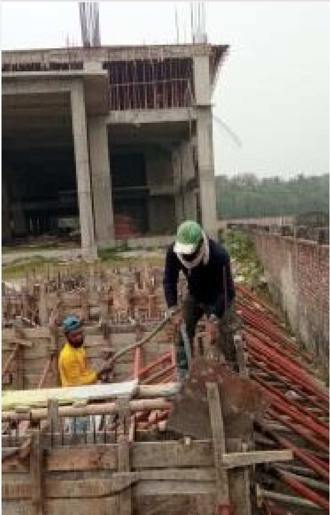
Septic Tank Wall Concreting on 27-01-22
