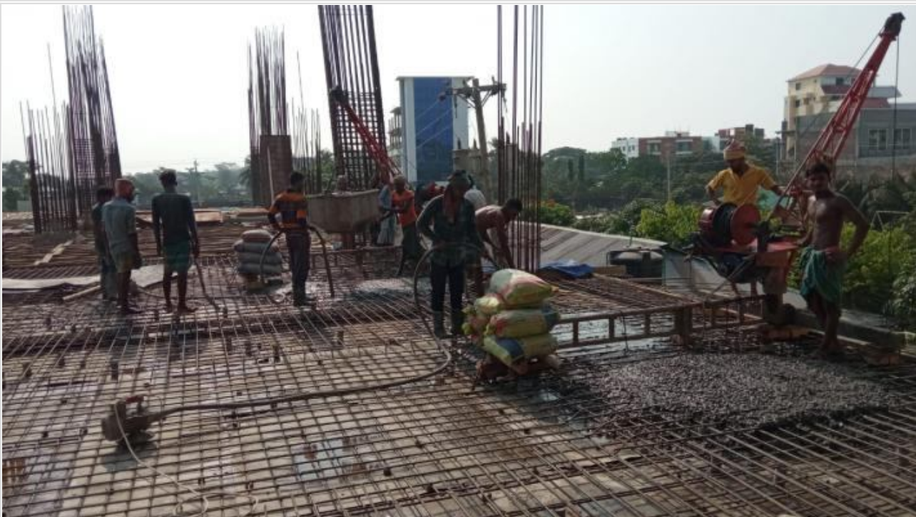
Between Tower1-2-GF Roof Slab-Concreting on 26-04-21
