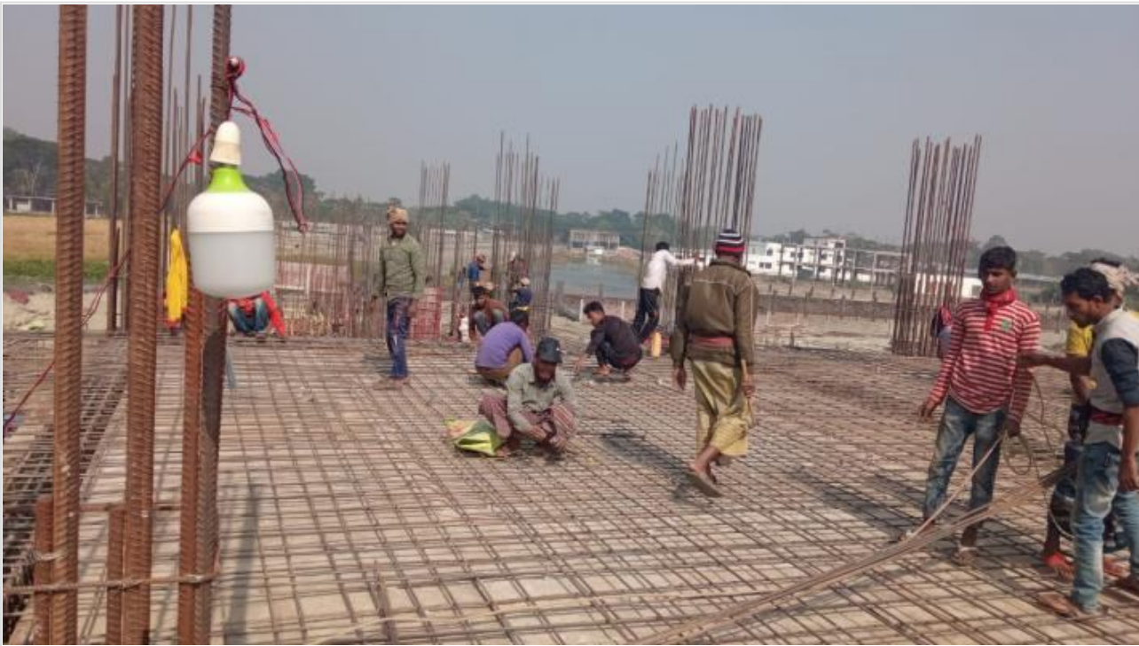
Tower-1-GF Slab Re-bar Work on 20-12-20
