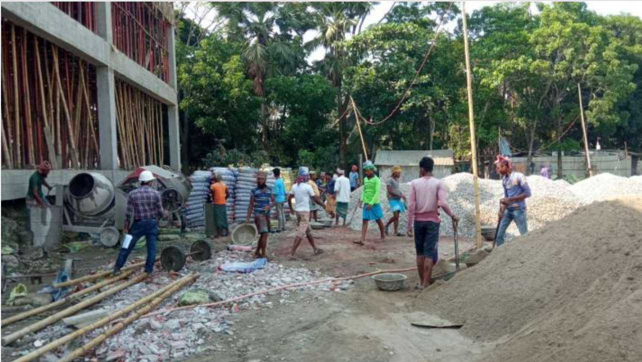
Restaurant GF Doubl Ht Slab-1-4/A-B-Conc on 24-04-21
