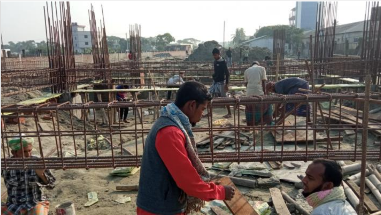
Tower-1-Grade Beam Re-bar Fabrication on 18-12-20
