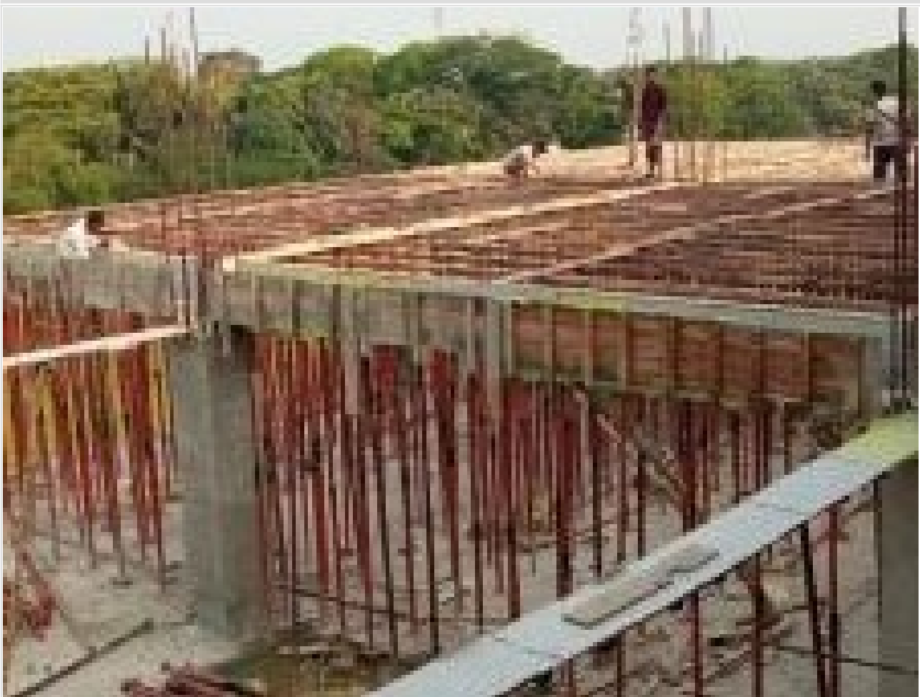
Beam Shuttering Work on 30-04-21
