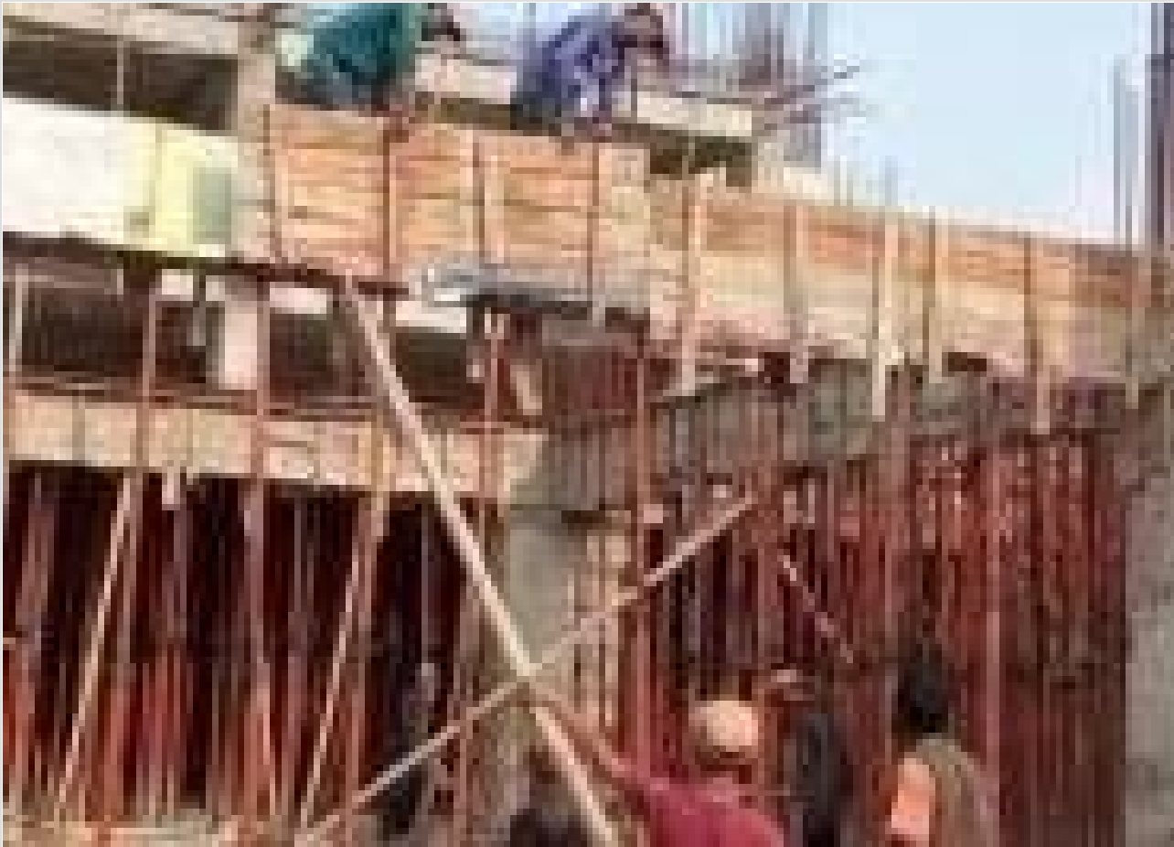
Beam Shuttering on 31-05-21
