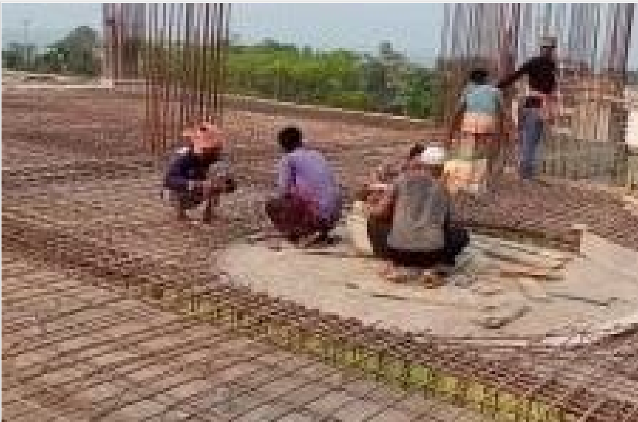
4th Floor Slab(3-5/B-E) Concreting-3600s on 24-03-21
