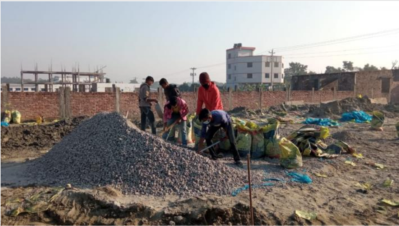
Tower-1-1st floor Roof Slab 2450sft Conc on 10-02-21
