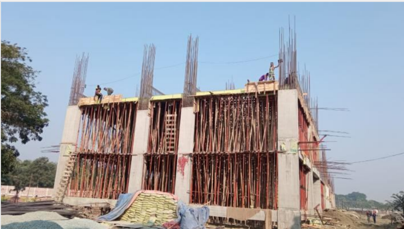
Tower-1-1st Floor Roof Slab Shuttering on 08-01-21
