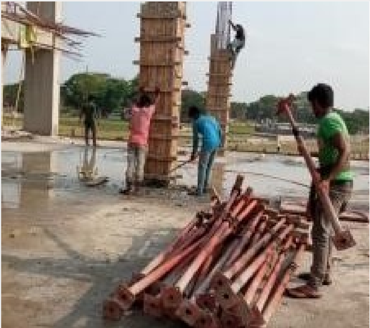
Column Concreting on 29-04-21
