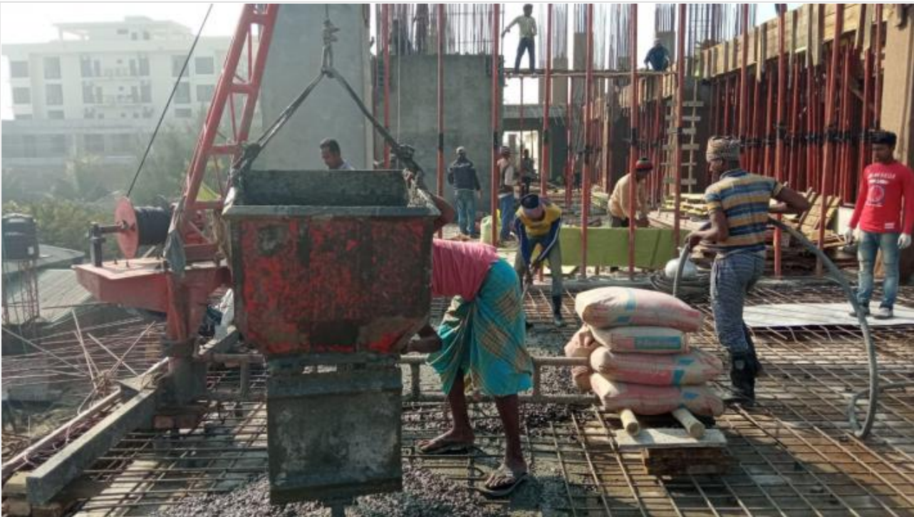
Tower-1-GF Roof Slab-4250sft Concreting on 27-01-21
