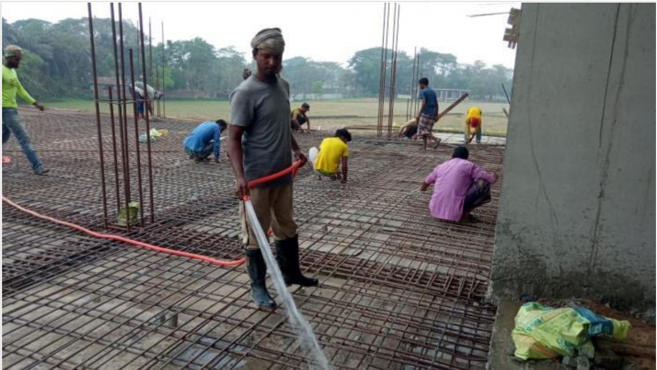
Restaurant-Double Height Slab Concreting on 02-03-21
