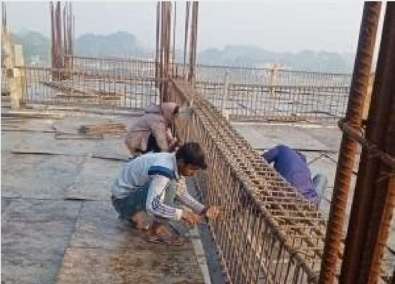
Tower-2-3rd Floor-Re-bar Work on 08-01-22
