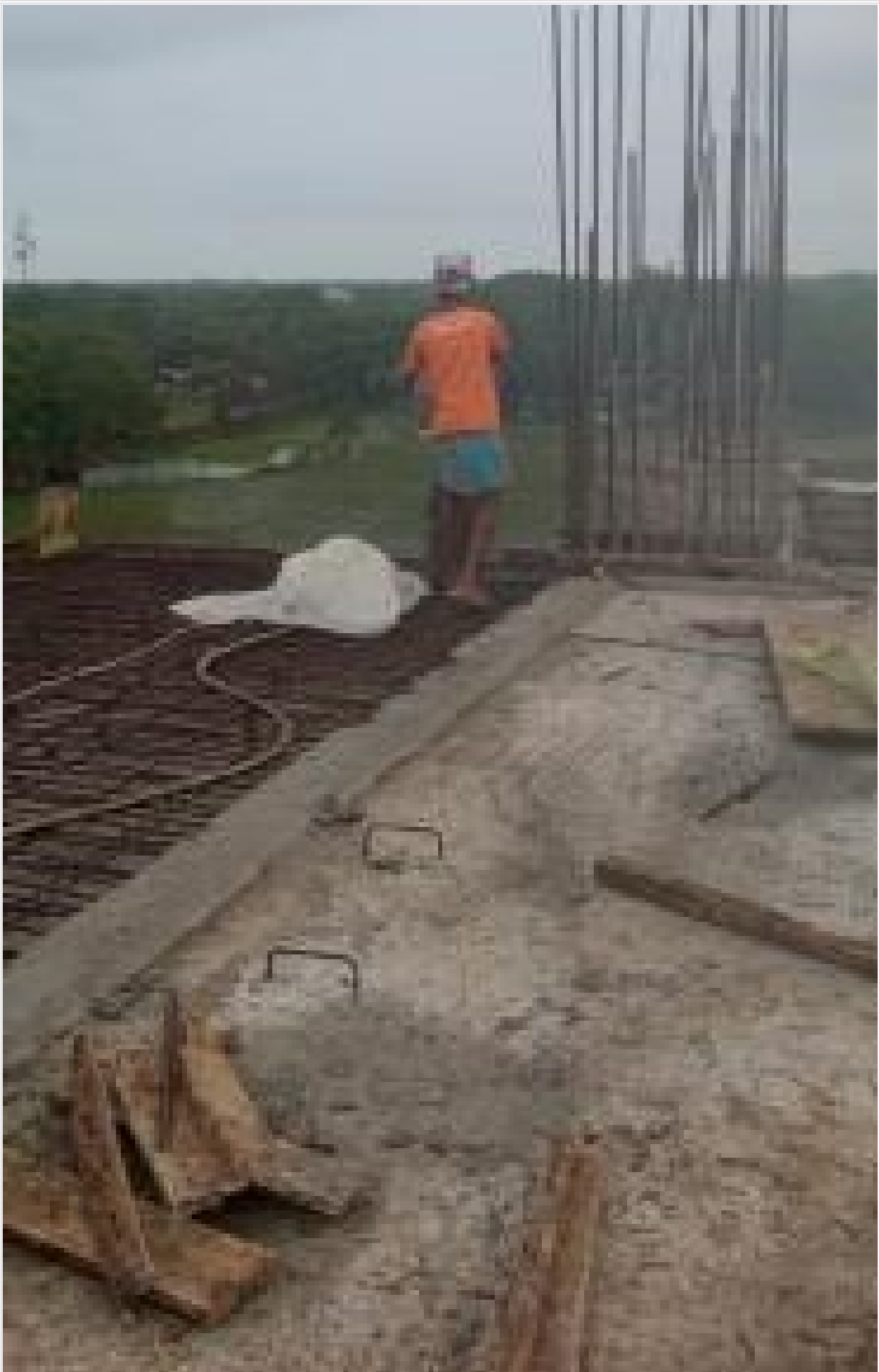
Tower-1-4th Floor Concreting on 22-06-21
