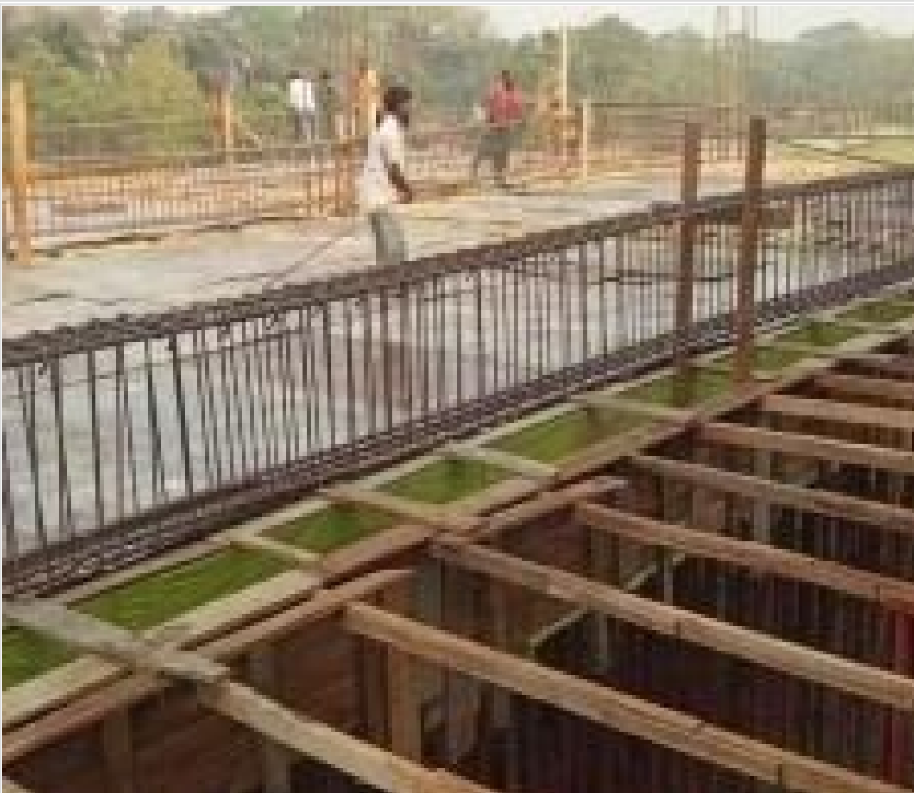
Tower-1-3rd Floor Roof Slab Shuttering on 13-03-21
