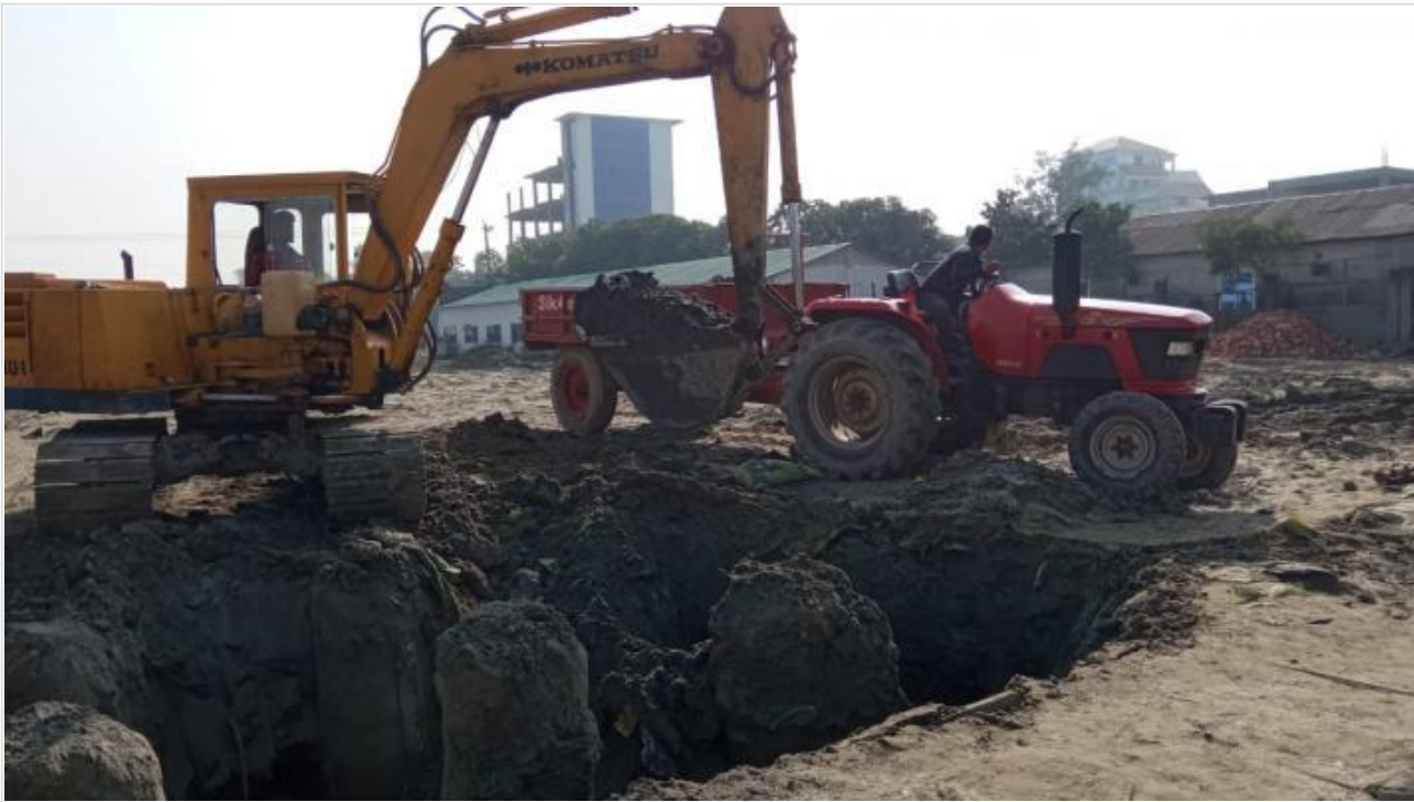
Tower-2-Excavation for Pile Head Breakin on 24-12-20
