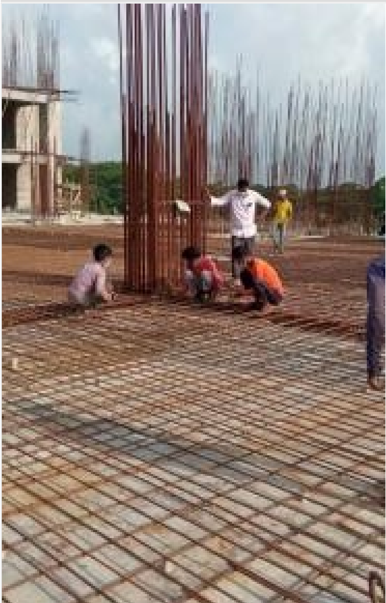
Tower-2:2nd floor slab re-bar work on 04-07-21
