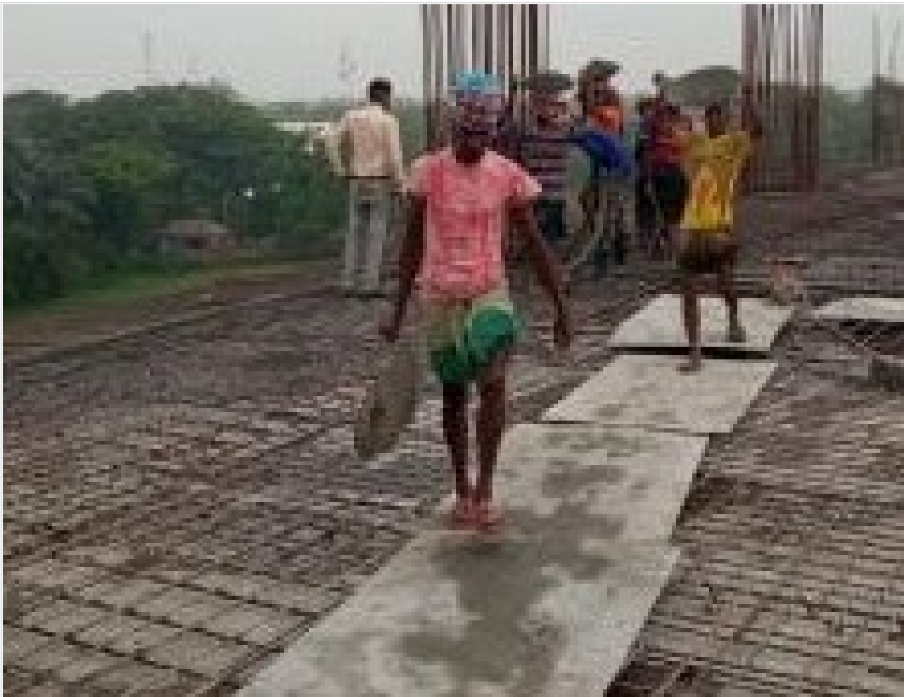
Tower-1-3rd Flr Roof Slab(B-E/5-6)Concret on 30-03-21
