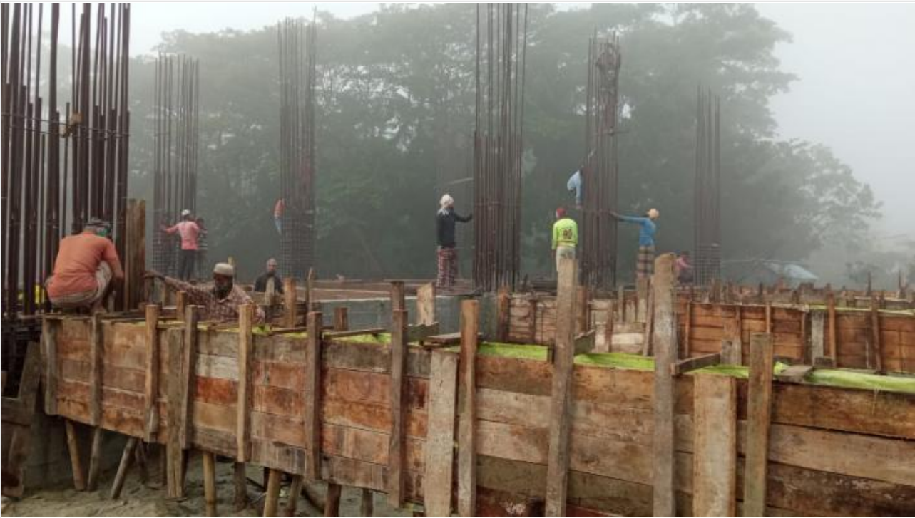
Tower-1 Grade Beam on 07-12-20
