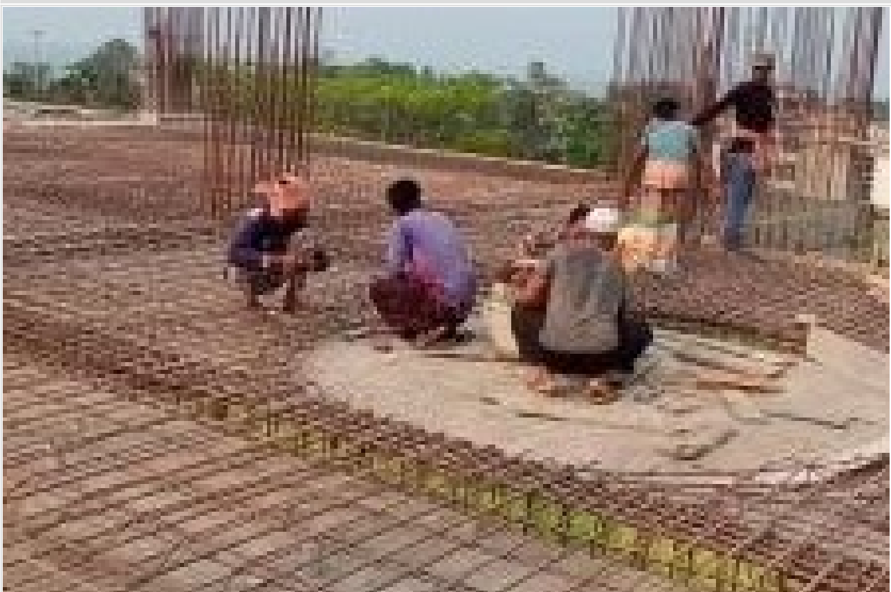
4th Floor Slab(3-5/B-E) Concreting-3600s on 24-03-21
