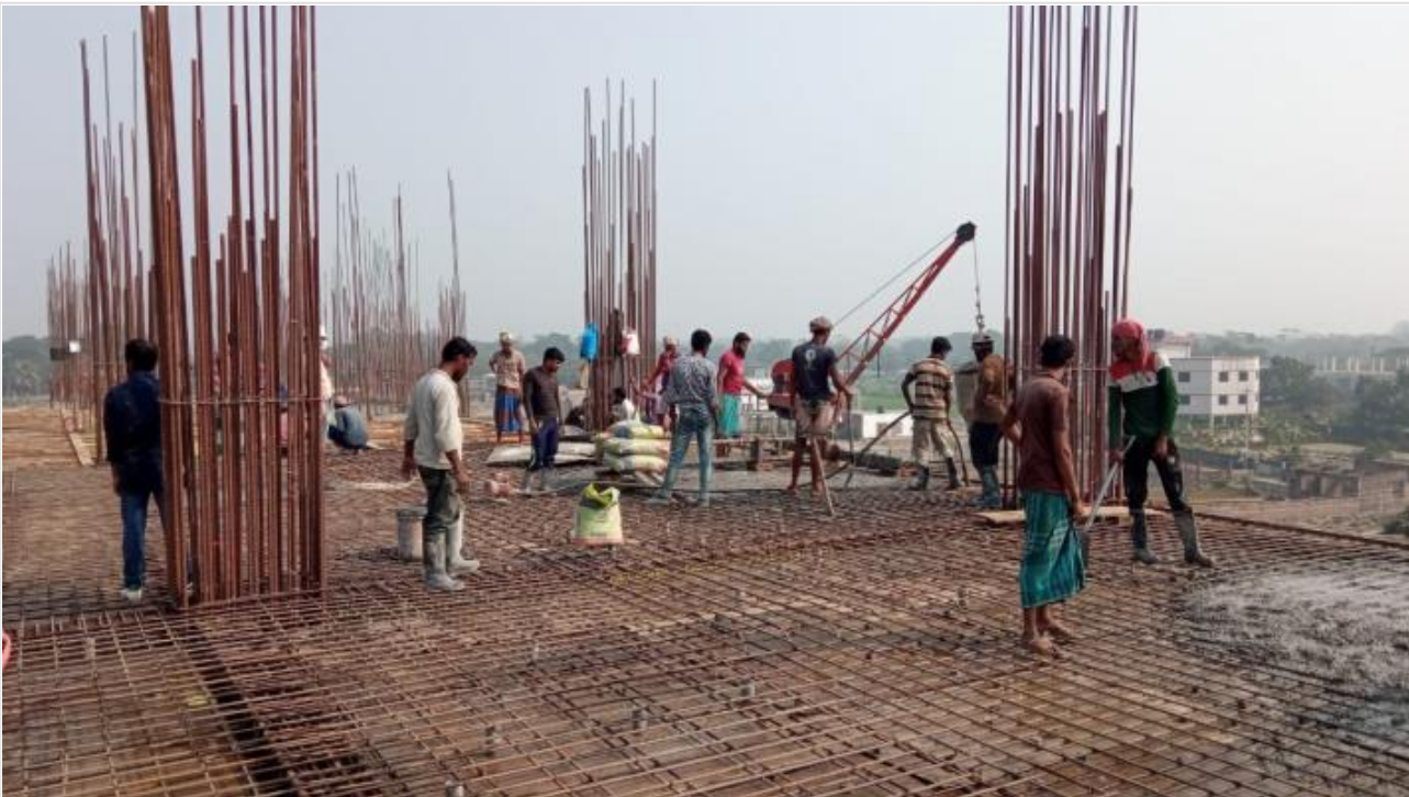
Tower-1-2nd Floor Roof Slab-3600sft Conc on 16-02-21
