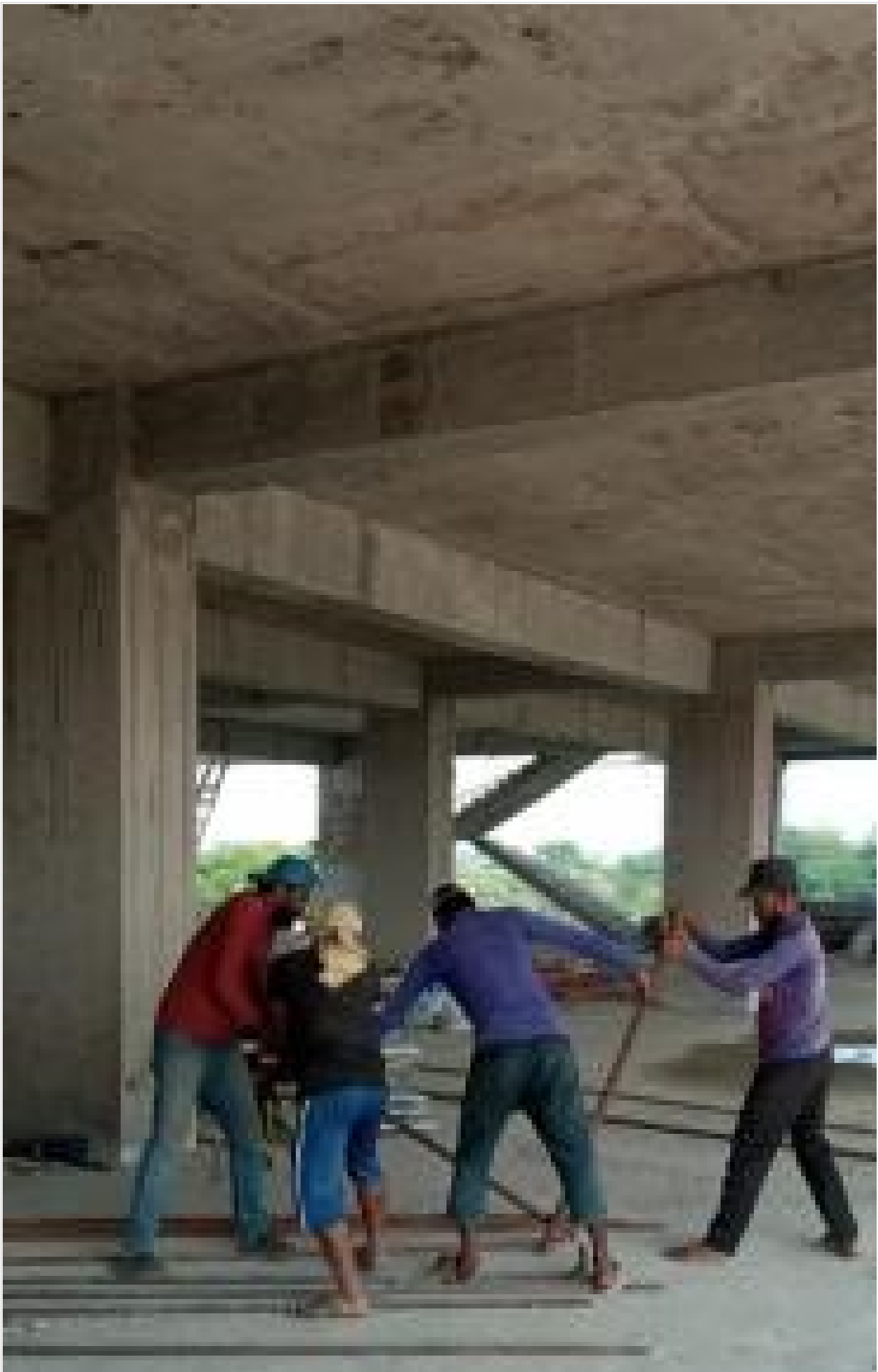
Tower-2-3rd Floor Beam Re-bar fabricatio on 01-11-21
