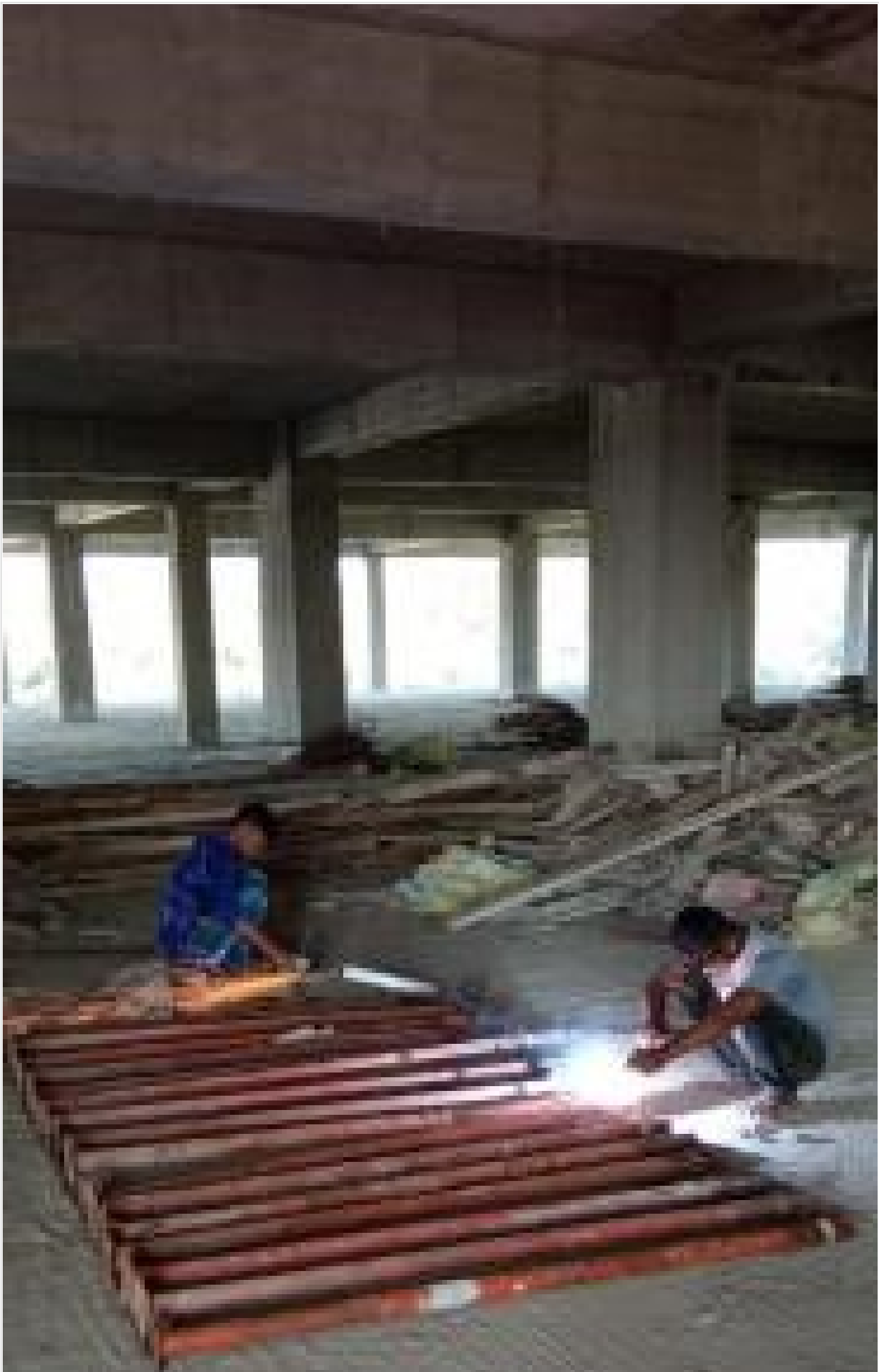
MS Prop Repairing on 01-12-21
