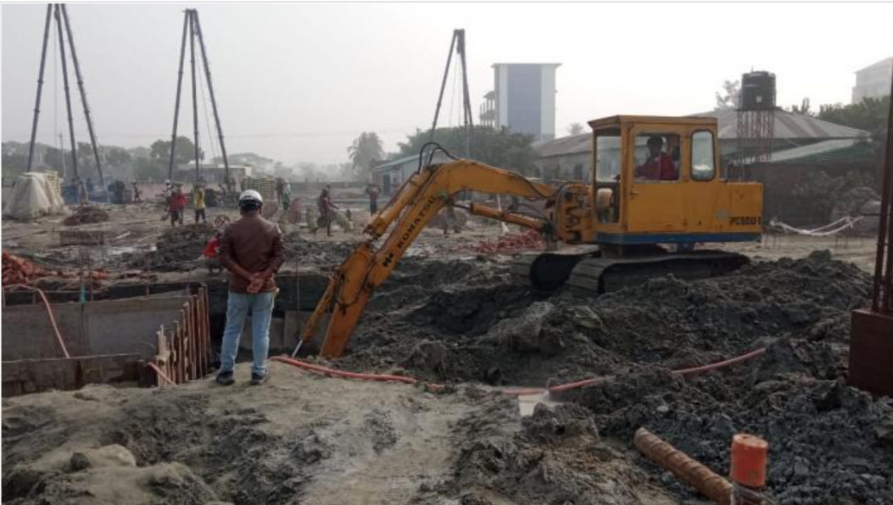
Tower-1-Excavation for Pile Cap on 09-12-20
