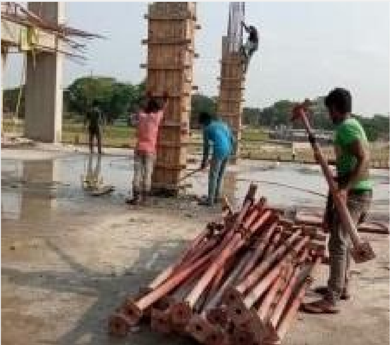
Column Concreting on 29-04-21
