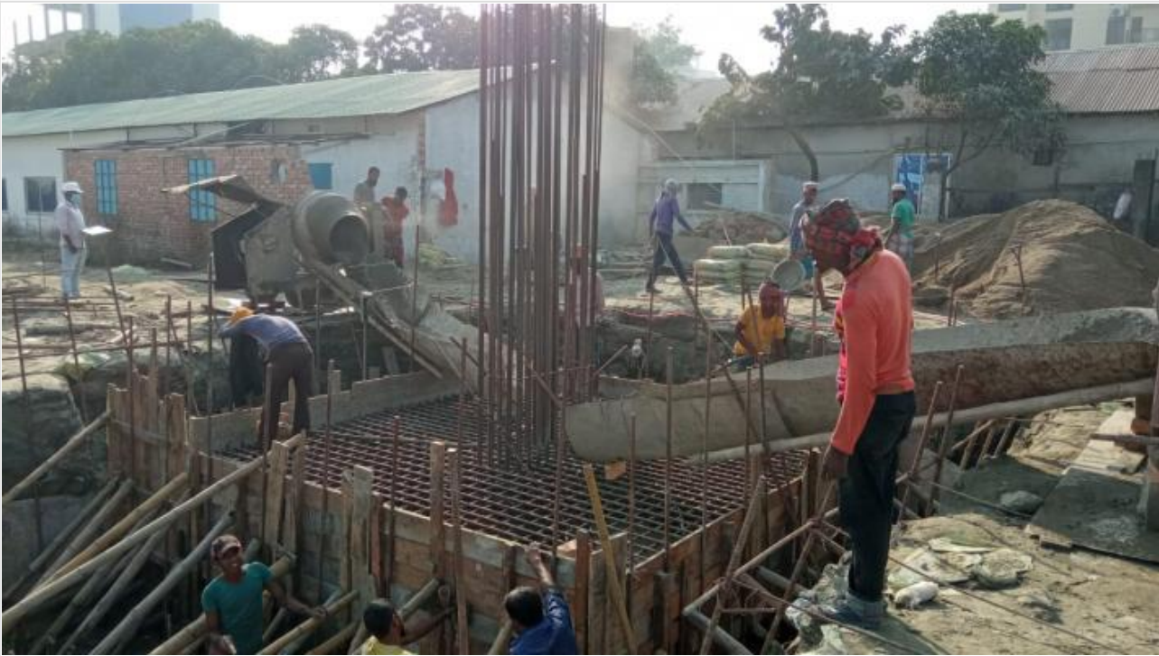
Tower-2-Pile Cap Concreting on 08-01-21
