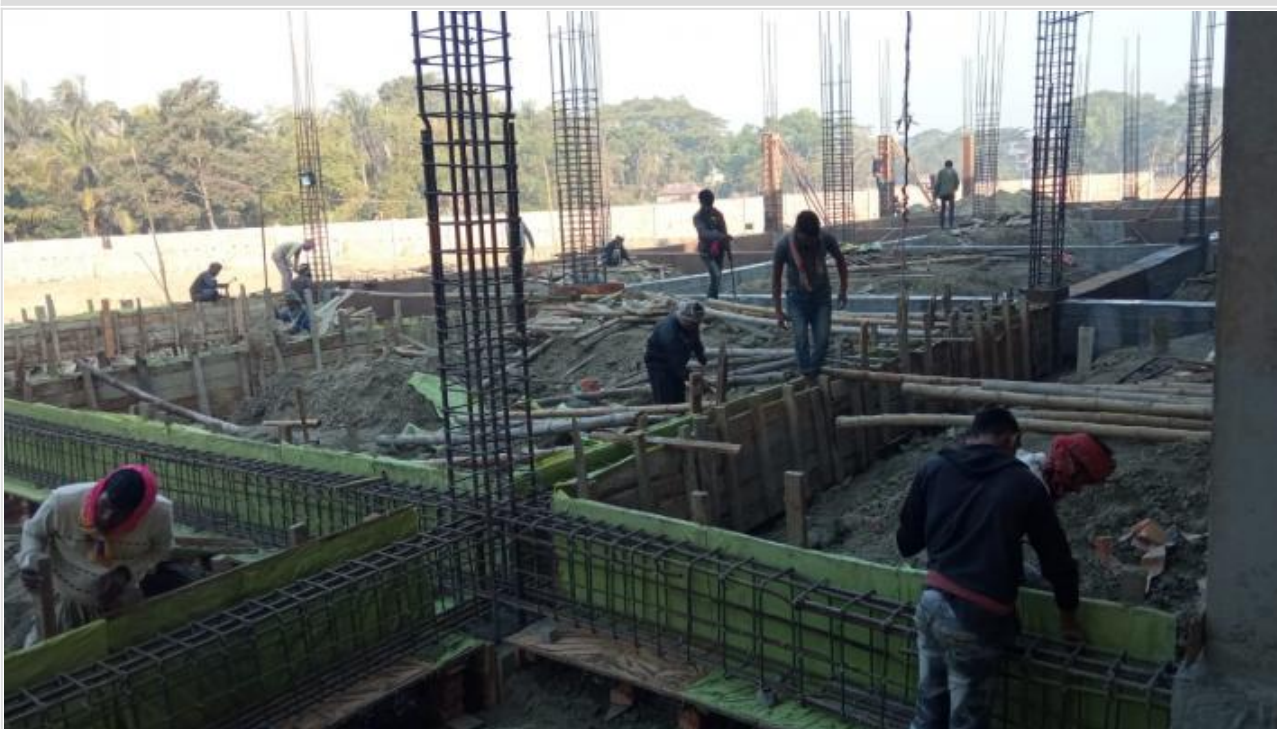
Tower-2-Grade Beam Shuttering on 10-02-21
