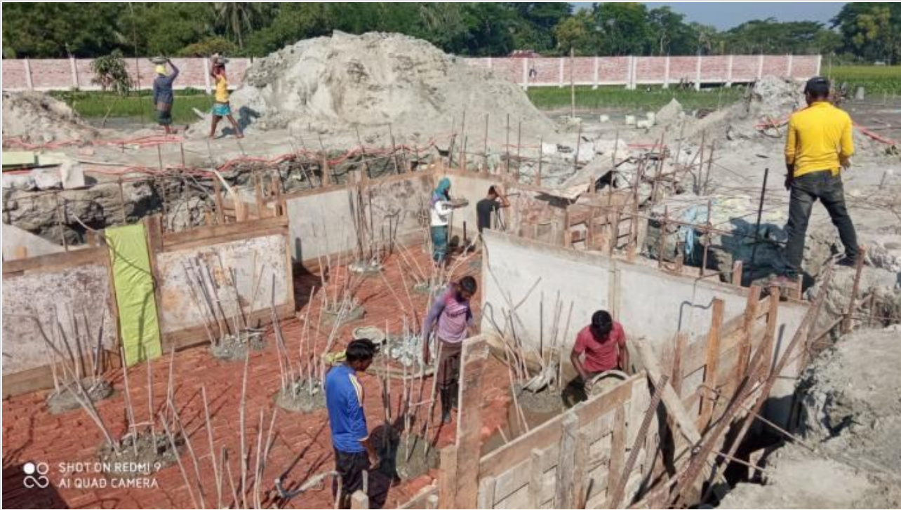
Tower-1-Pile Cap Work on 28-11-20
