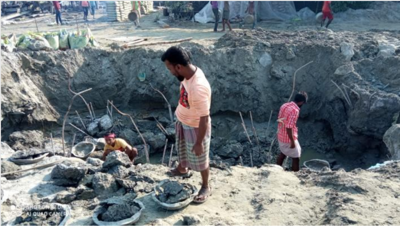
Tower-1-Pilehead breaking on 30-11-20
