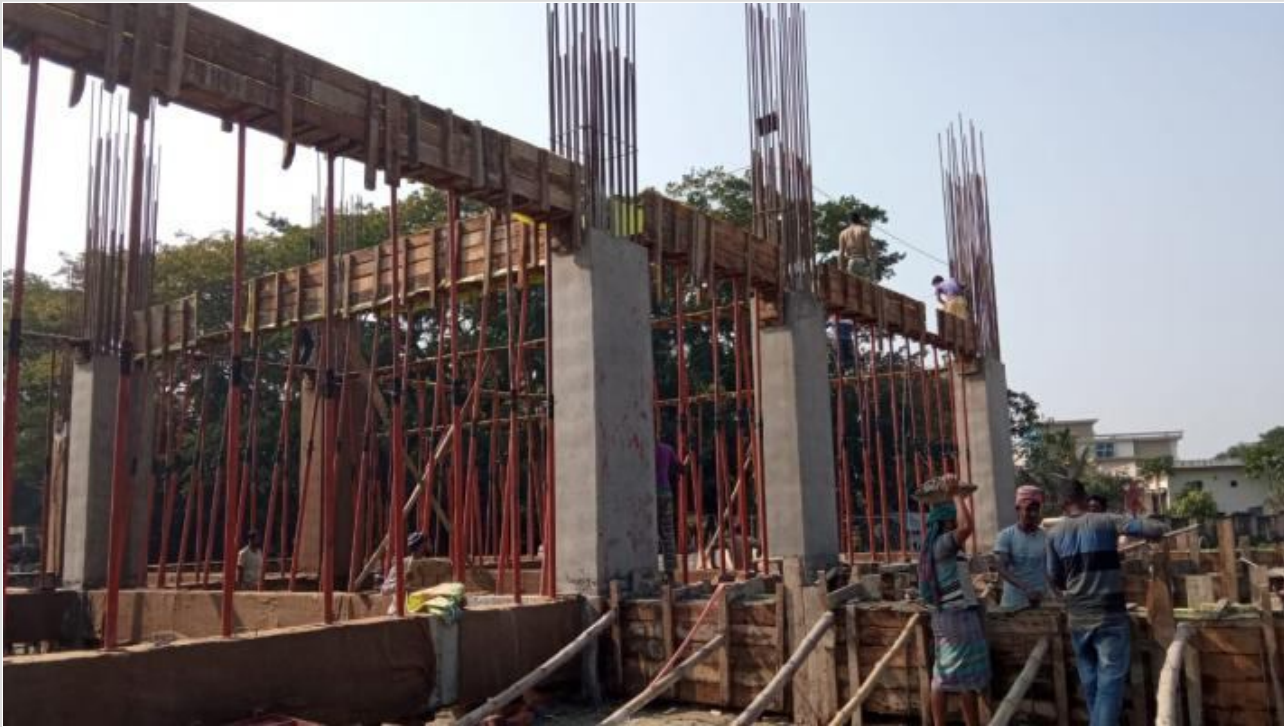
Tower-1-GF Beam Shuttering on 15-12-20
