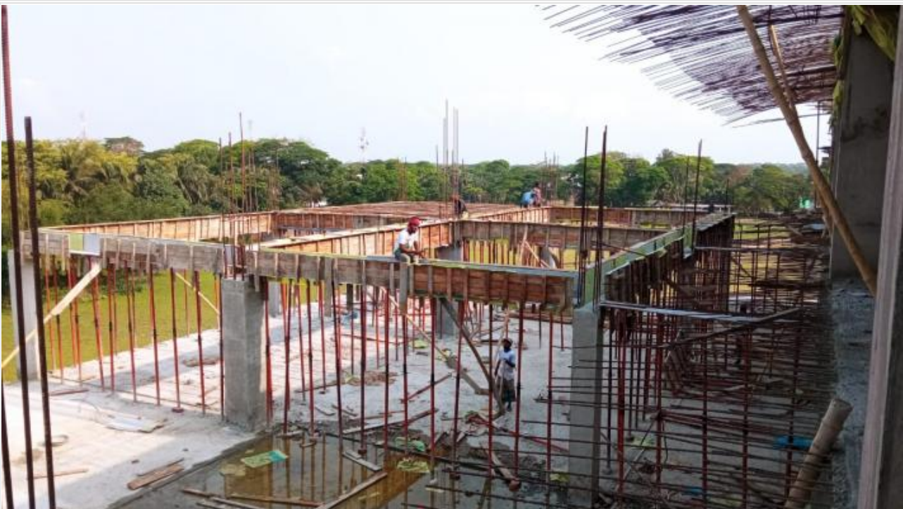
Beam Shuttering on 28-04-21
