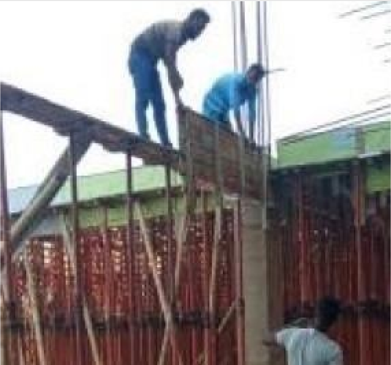
Roof Beam Shuttering on 09-05-21
