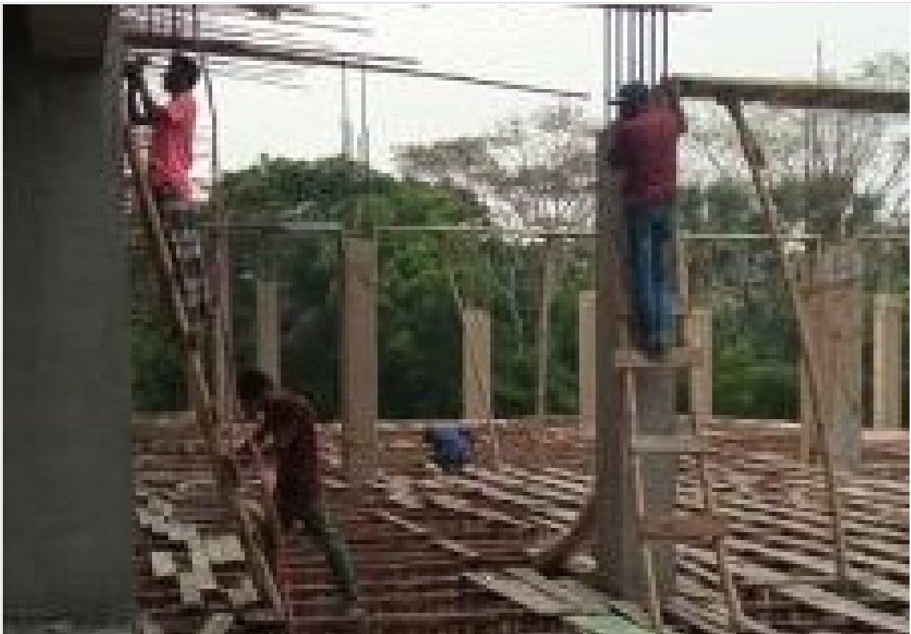
Tower-1-3rd Floor Roof Slab-Beam Shutter on 23-03-21
