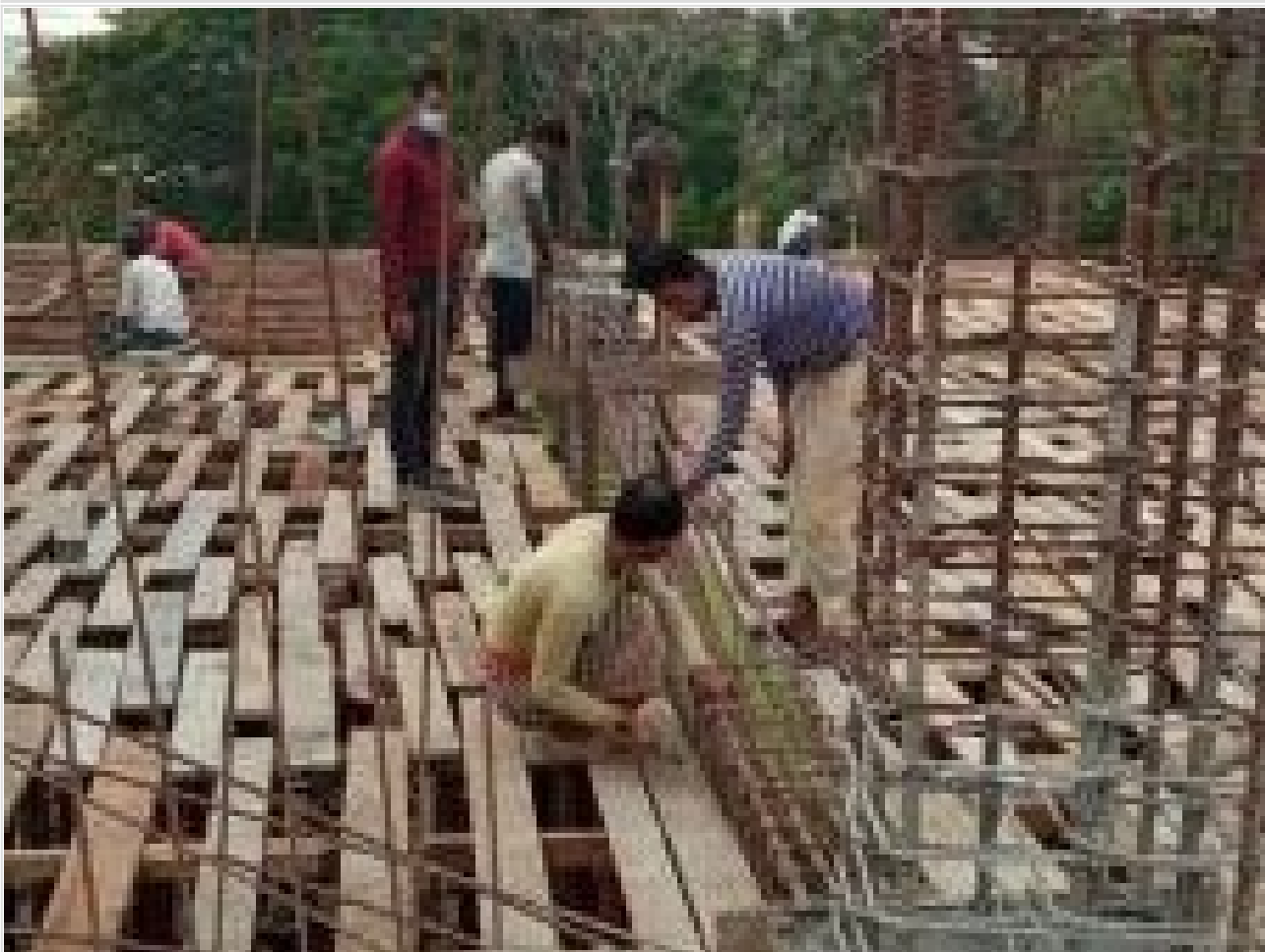
Restaurant-GF Double Ht Roof Slab-Re-bar on 30-03-21
