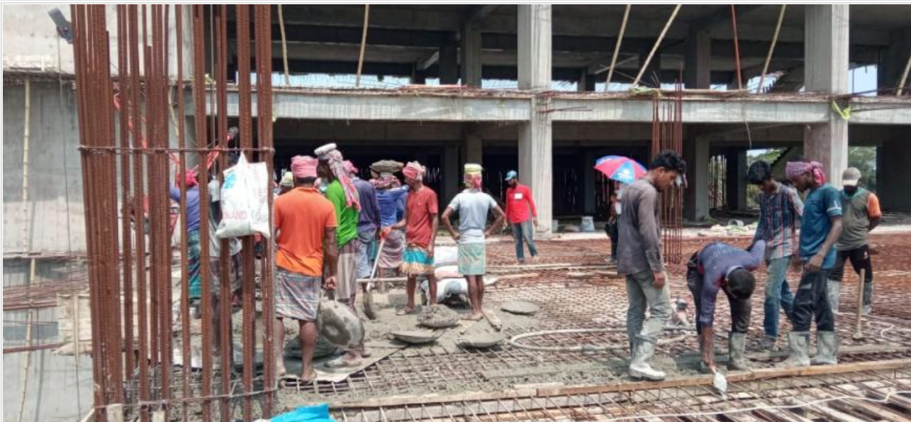
Between Tower1-2-1st Flr Roof Slab-Concr on 05-06-21
