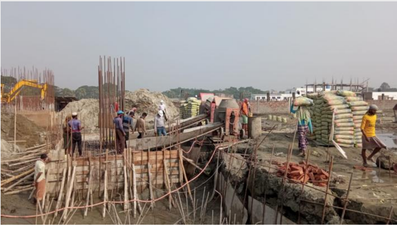
Tower-1-Pilecap Concreting on 12-12-20
