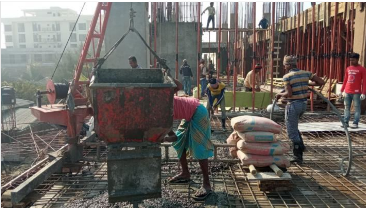
Tower-1-GF Roof Slab-4250sft Concreting on 27-01-21
