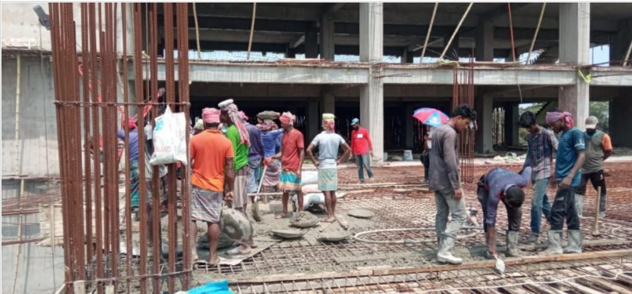
Between Tower1-2-1st Flr Roof Slab-Concr on 05-06-21
