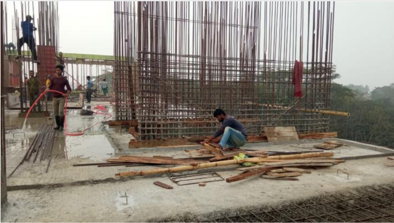
Tower-1-2nd Floor Roof Curing on 25-02-21
