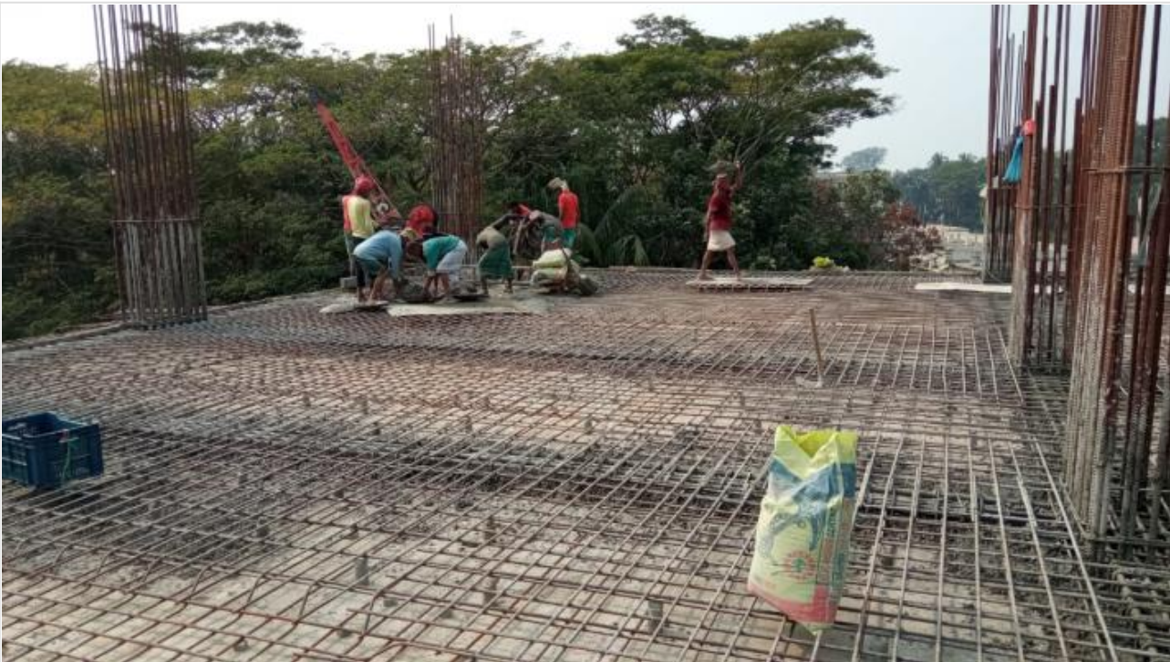
Tower-1-1st Floor Roof Slab 3600 sft Co on 11-01-21
