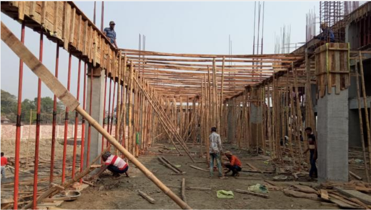
Restaurant Area Slab Shuttering on 23-02-21
