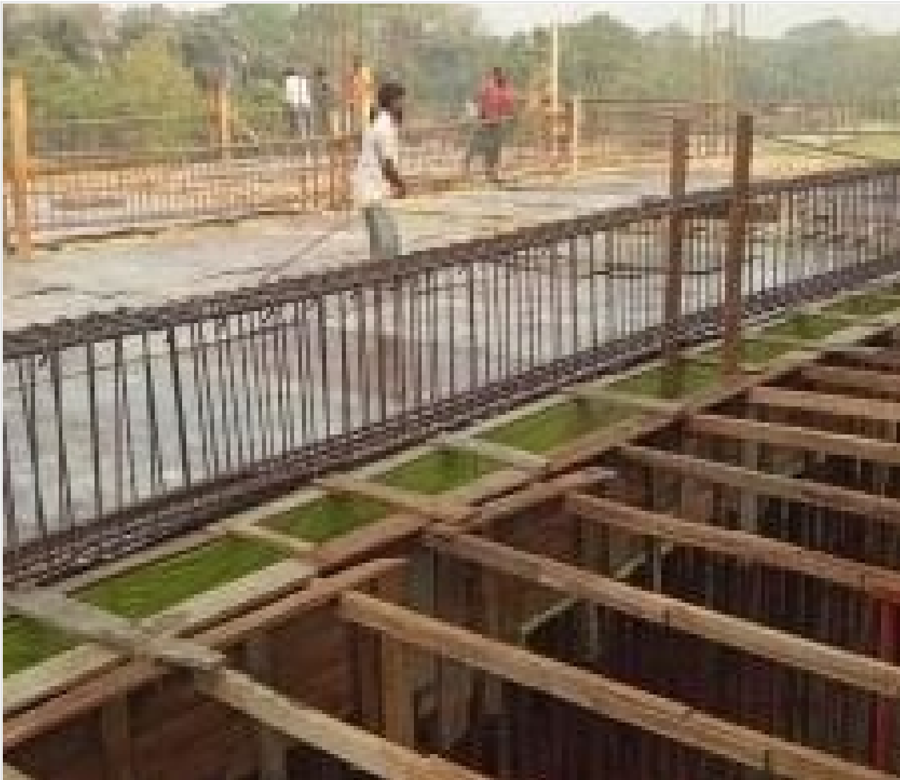
Tower-1-3rd Floor Roof Slab Shuttering on 13-03-21
