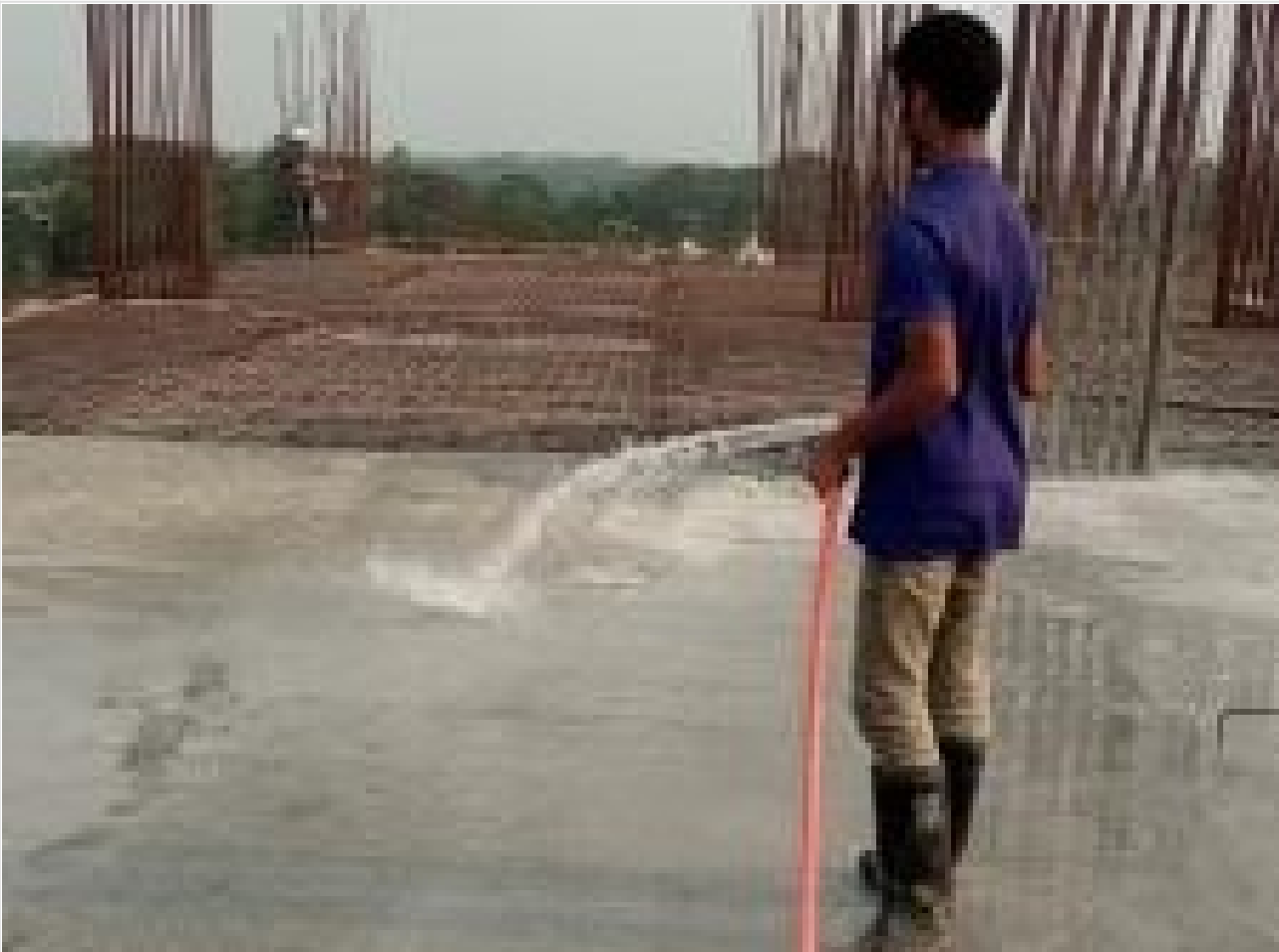
Tower-1-3rd Floor Roof Slab Curing on 31-03-21
