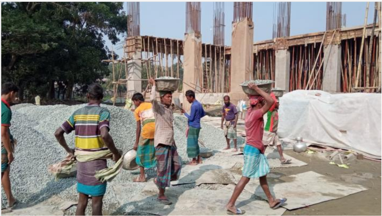
Tower-1-GF Roof Slab Concreting on 21-12-20
