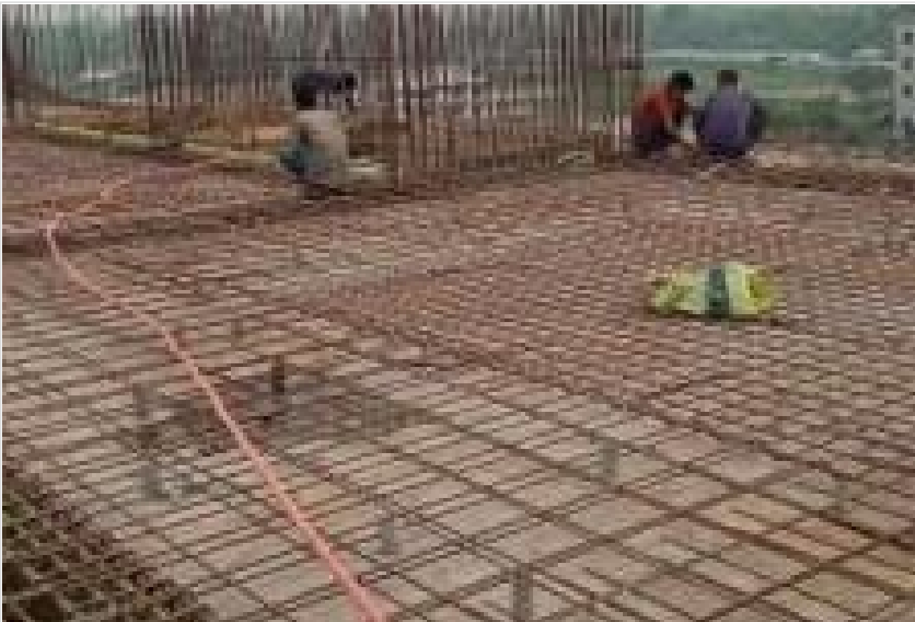
Restaurant GF Double Height Slab-6-9/A-B on 23-03-21
