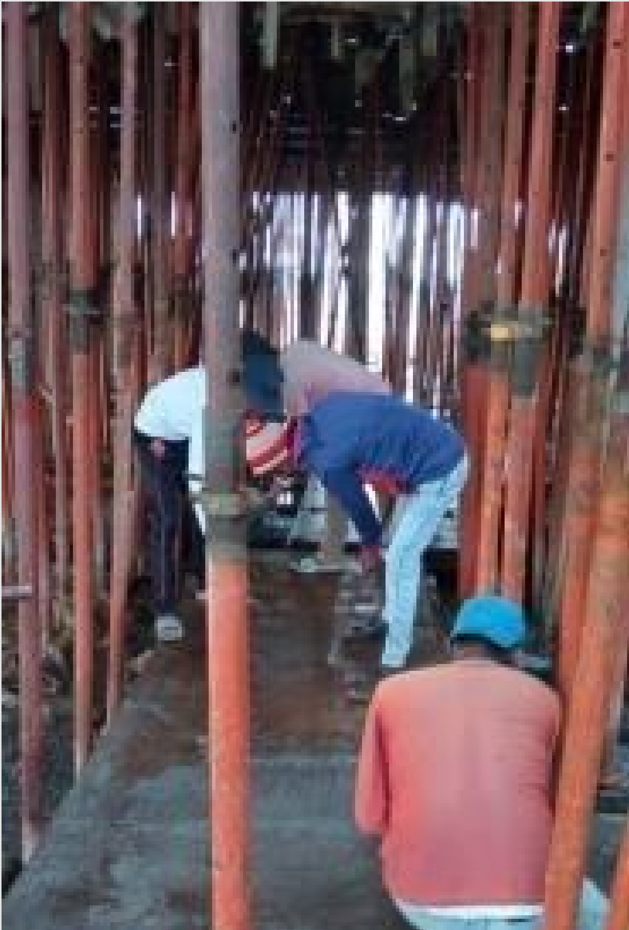
Column/Wall Steel Shutter Cleaning, Oili on 21-02-22
