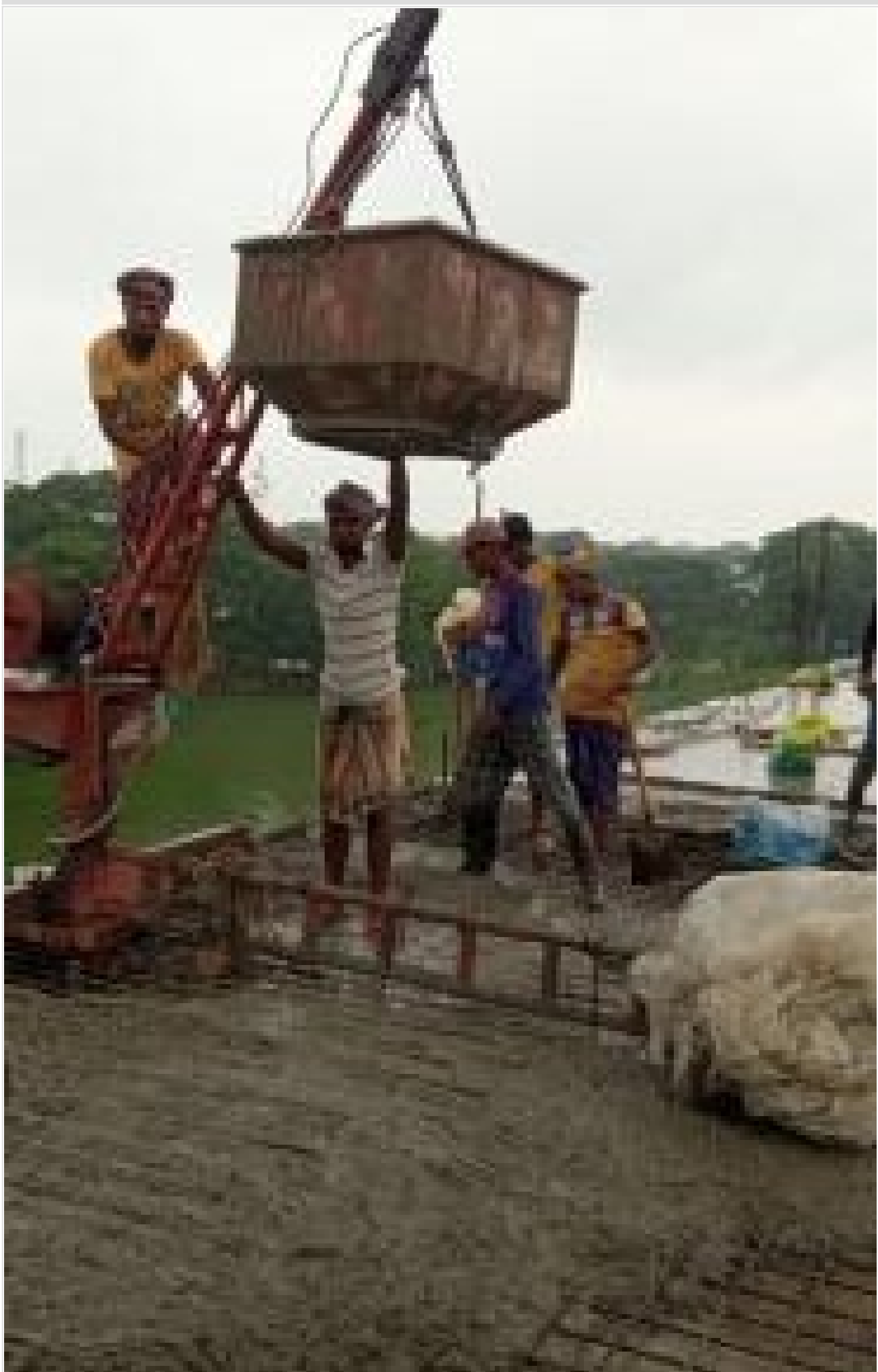
Restaurant-3rd Floor Slab Concreting on 16-06-21
