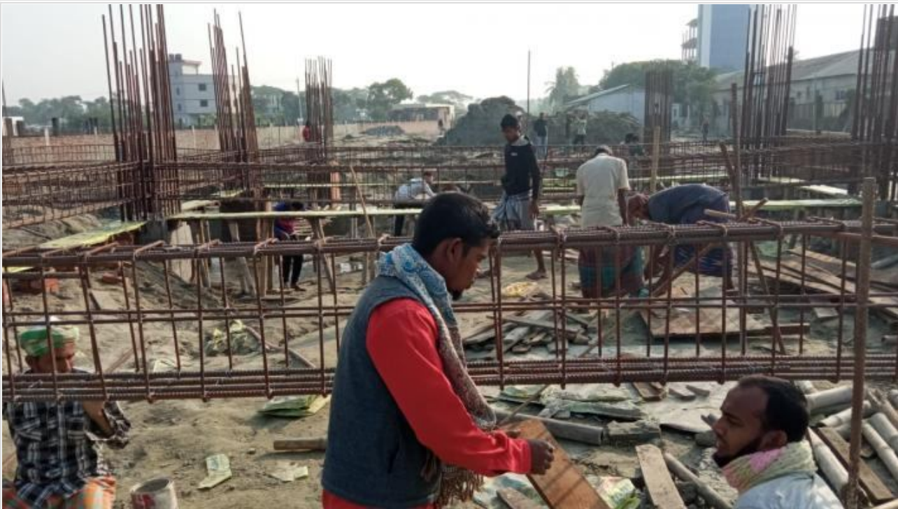
Tower-1-Grade Beam Re-bar Fabrication on 18-12-20
