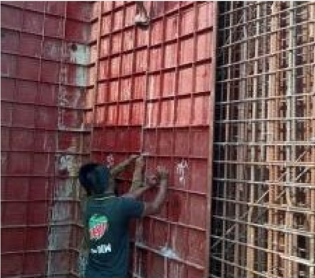
Lift Core Wall Shuttering on 26-04-21
