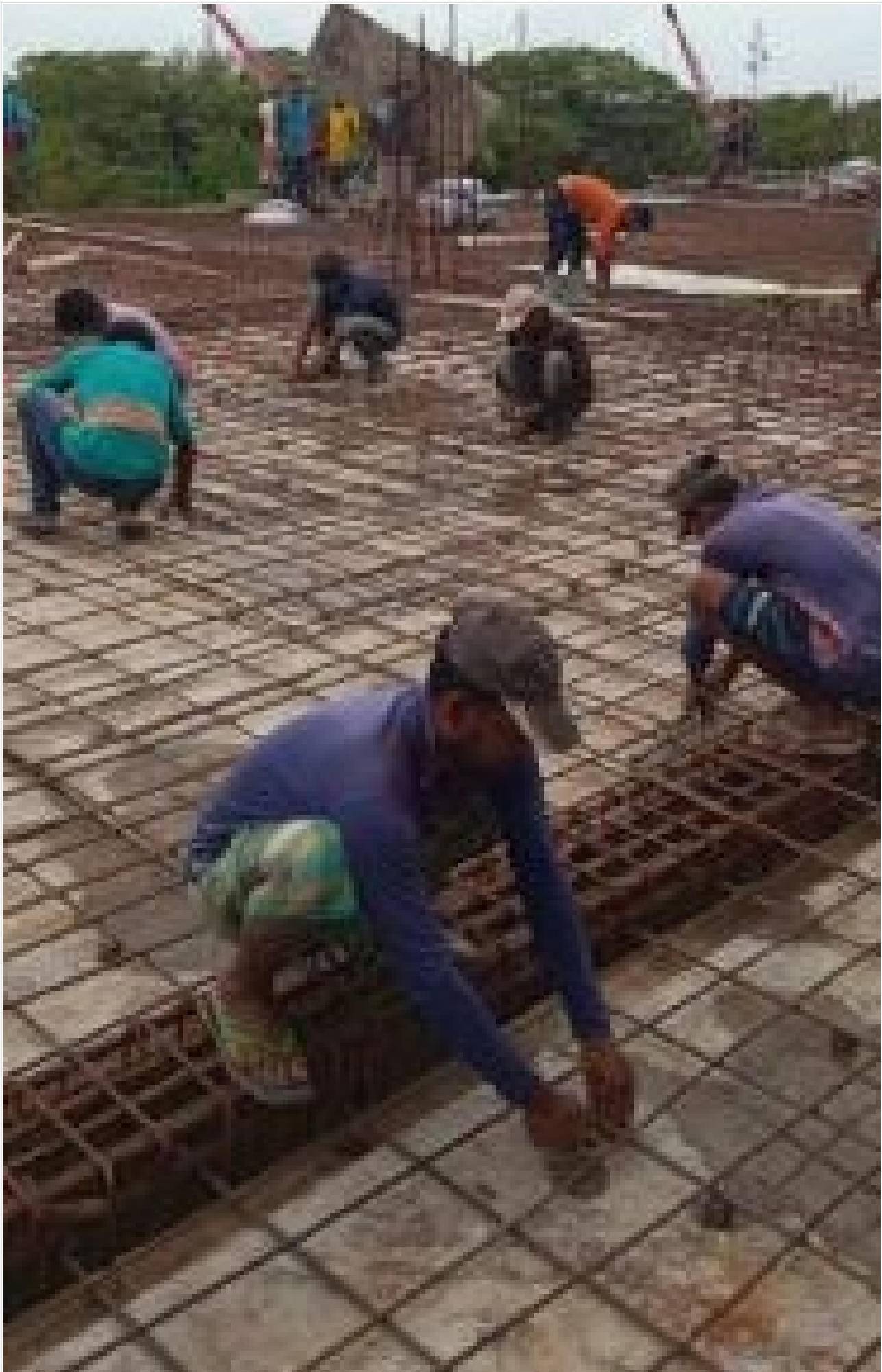
Restaurant-3rd Floor Slab Re-bar Work on 12-06-21
