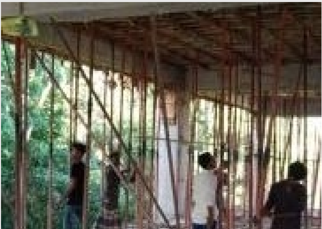
Restaurant GF Double Height Roof Slab on 24-05-21
