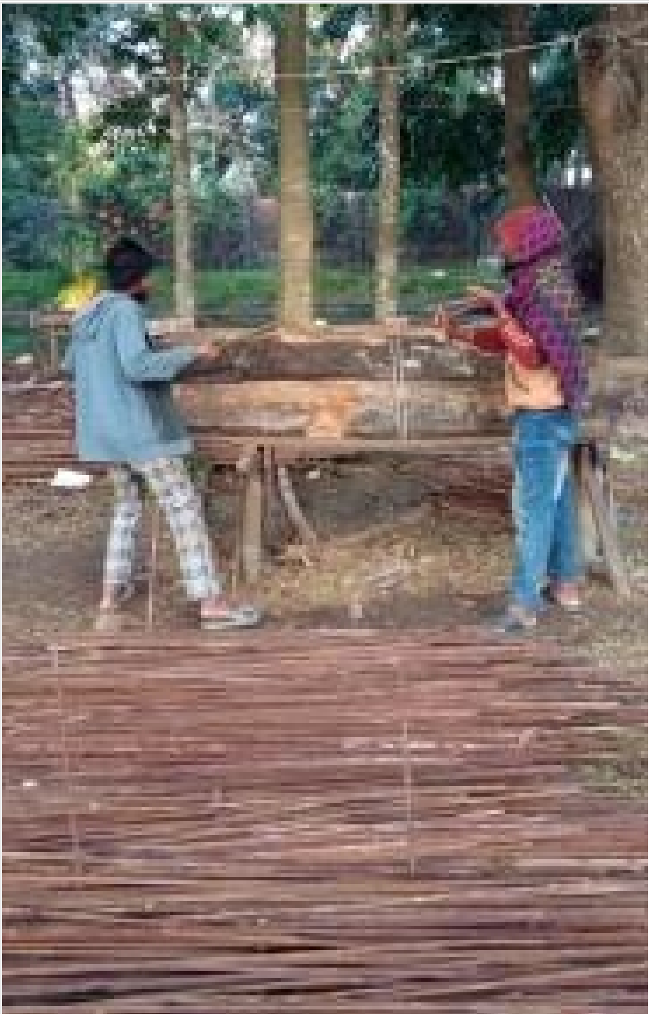
Re-bar Fabrication on 31-12-21
