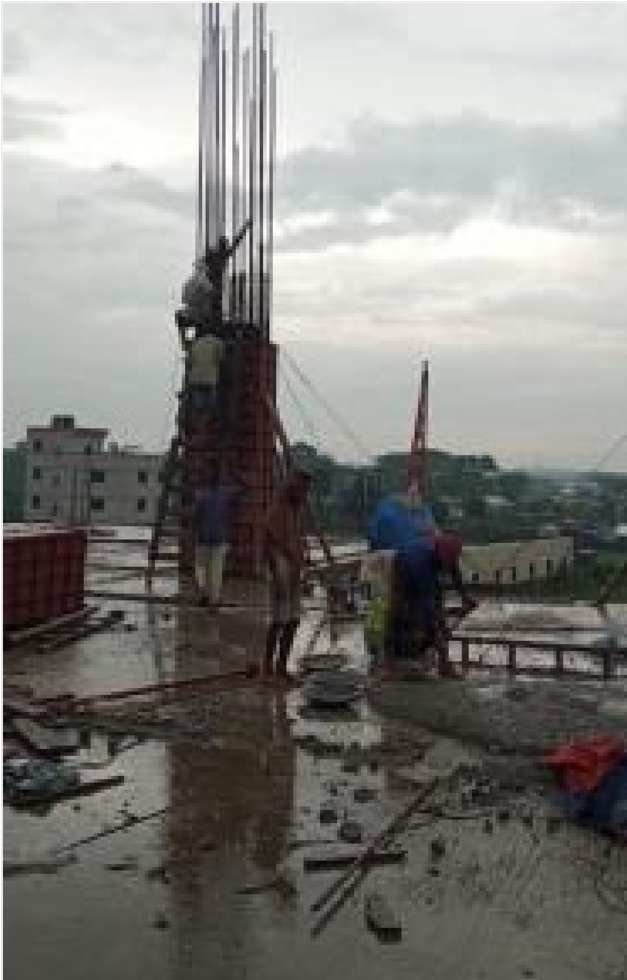
Tower-2-2nd Floor Column Concreting on 28-10-21
