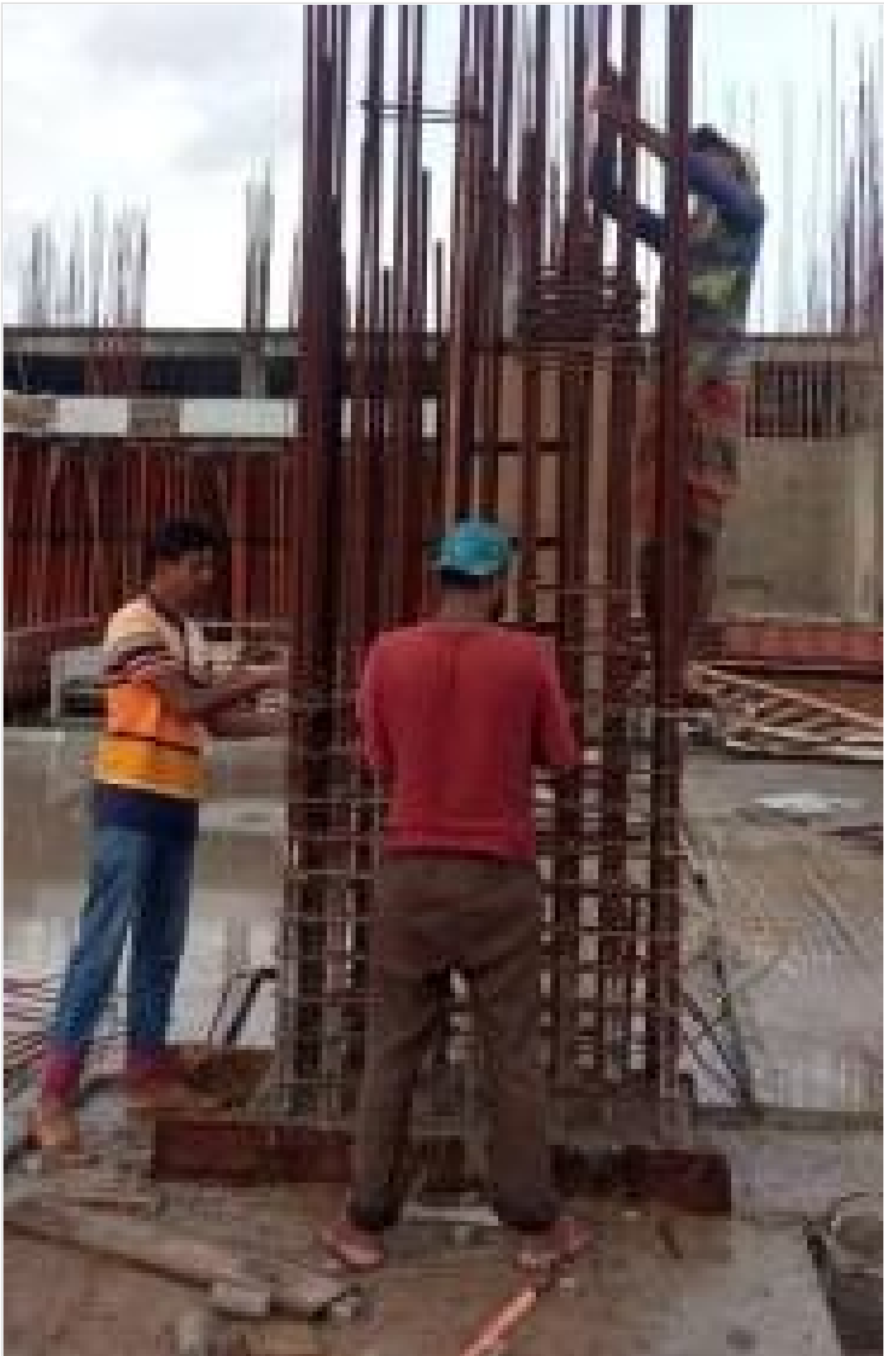
Tower-2-2nd Floor-Column Re-bar Work on 17-10-21
