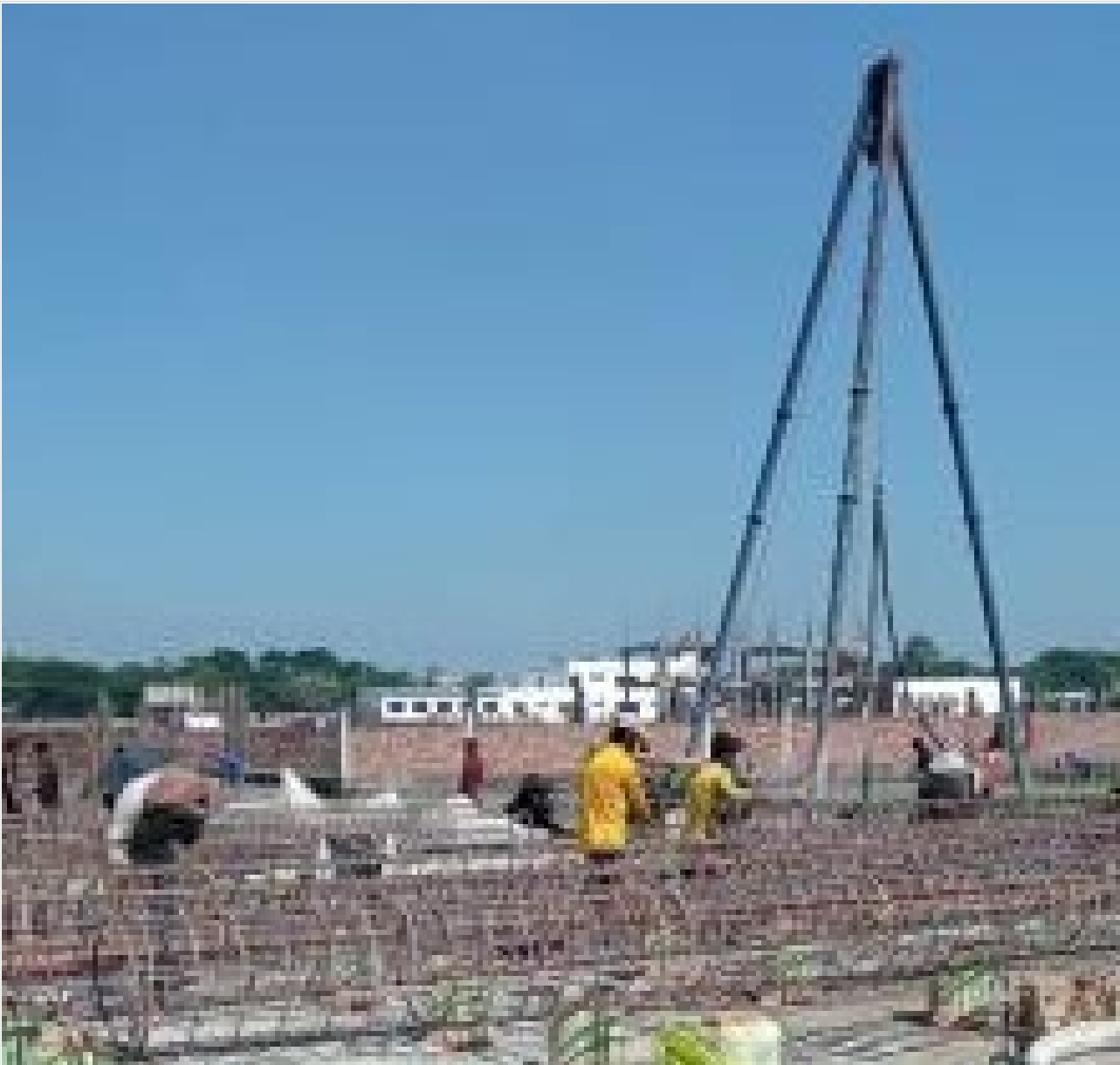
Tower-2-Pile Work on 12-11-20
