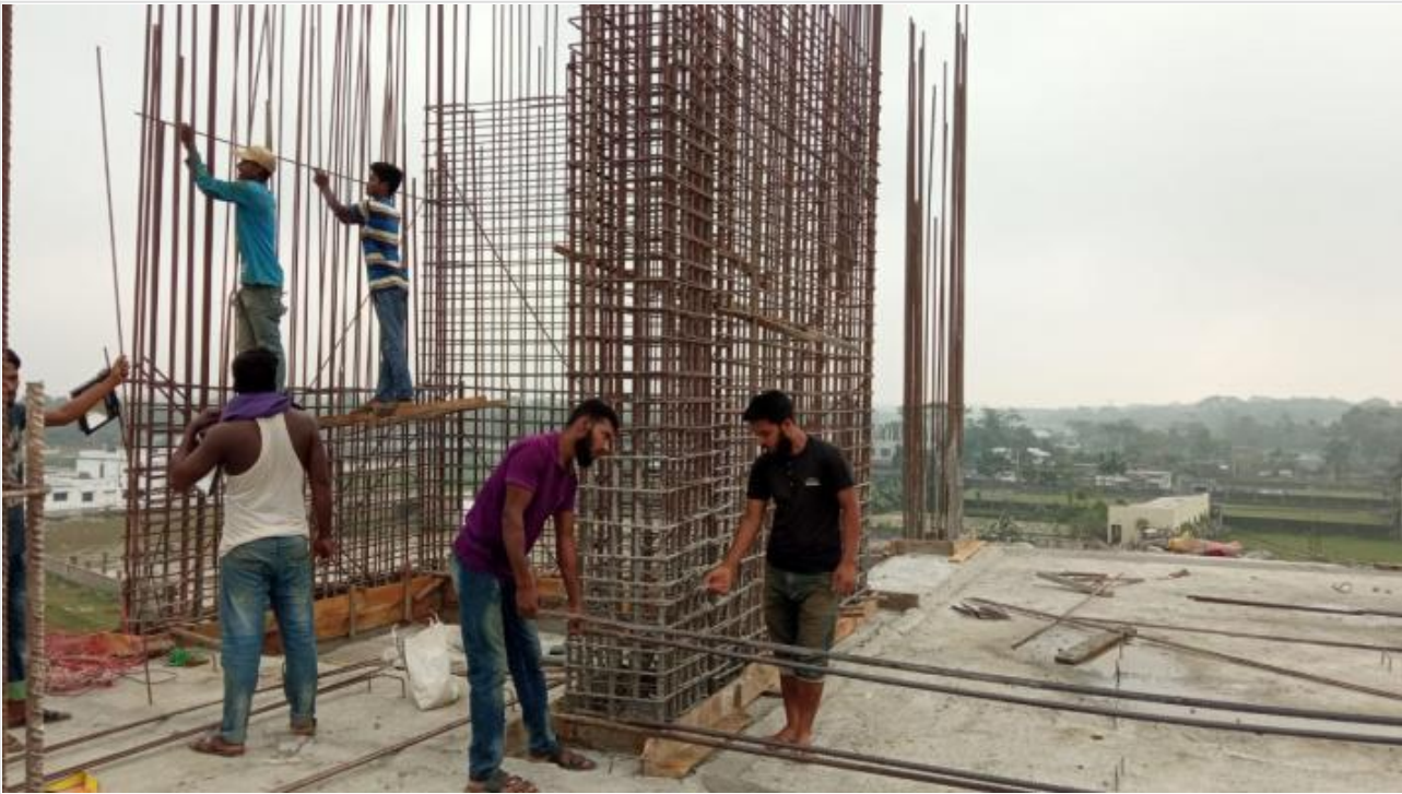
Tower-1-3rd Floor Lift Core Re-bar Work on 02-03-21
