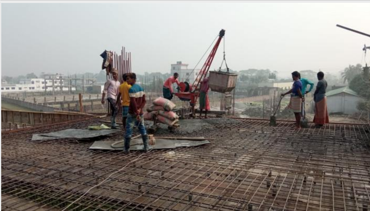
Tower-1-GF Roof Slab 1800 sft Concreting on 18-01-21
