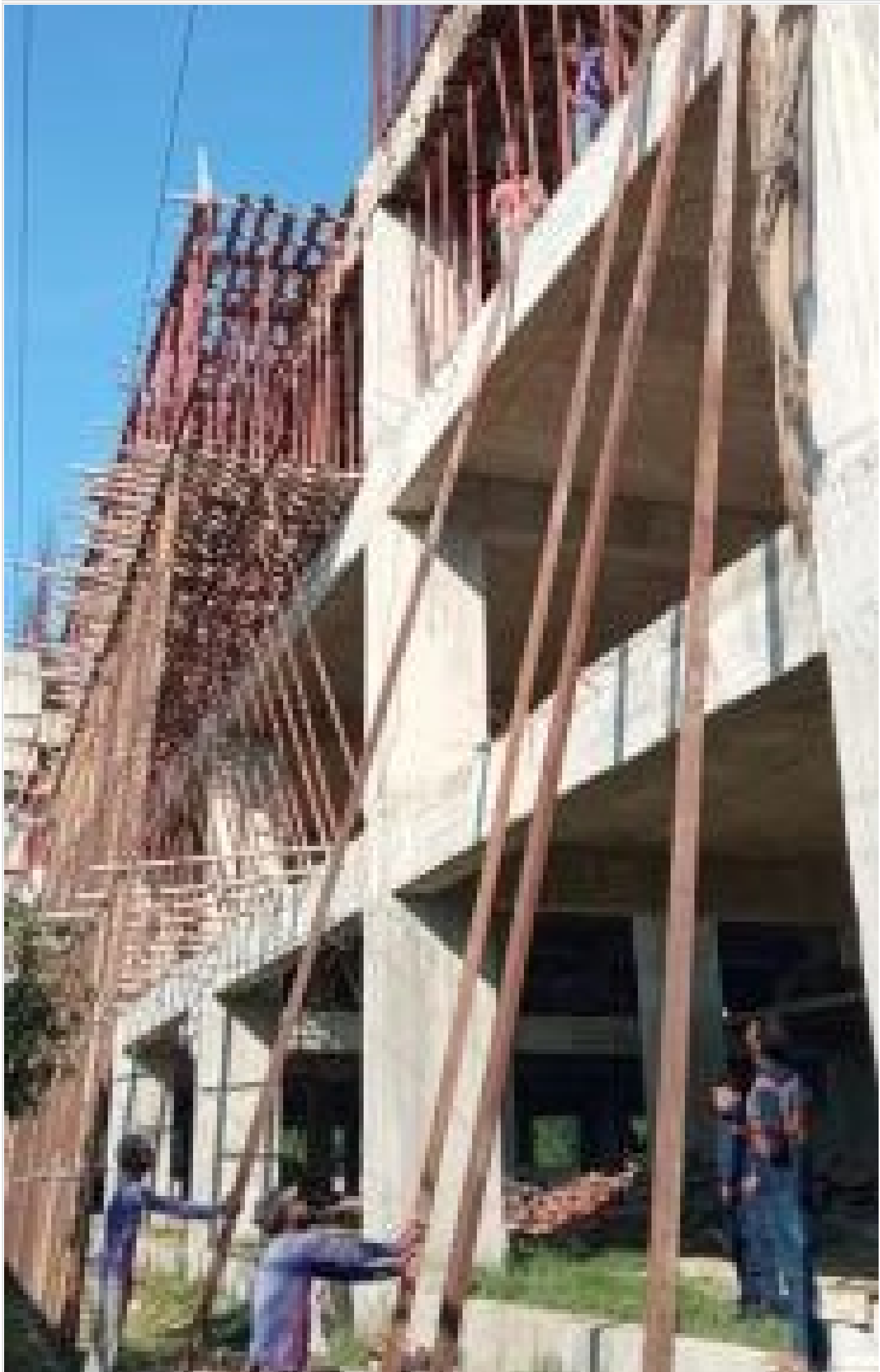
Tower-2-3rd Floor Slab-shuttering on 01-12-21
