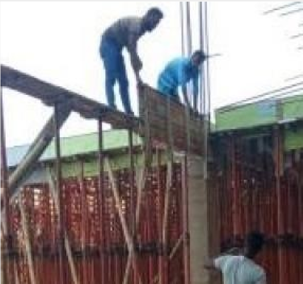
Roof Beam Shuttering on 09-05-21
