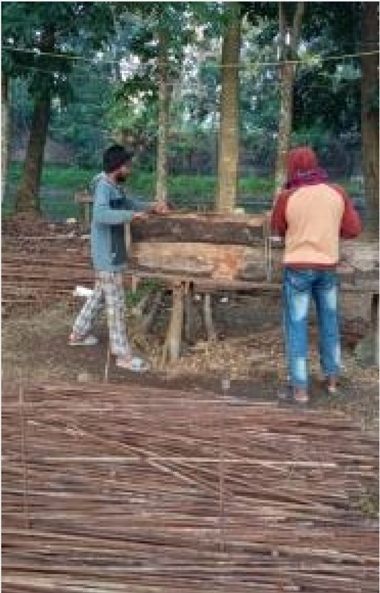
Re-bar Fabricating on 01-01-22
