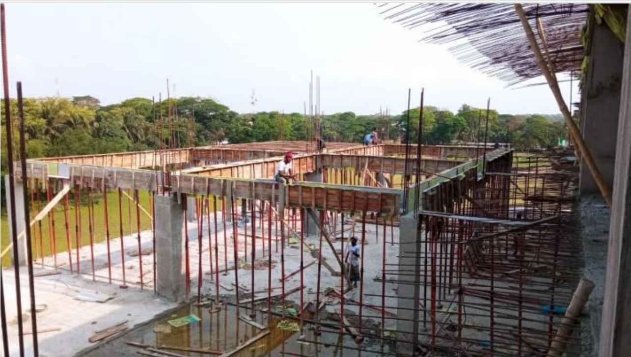
Beam Shuttering on 28-04-21
