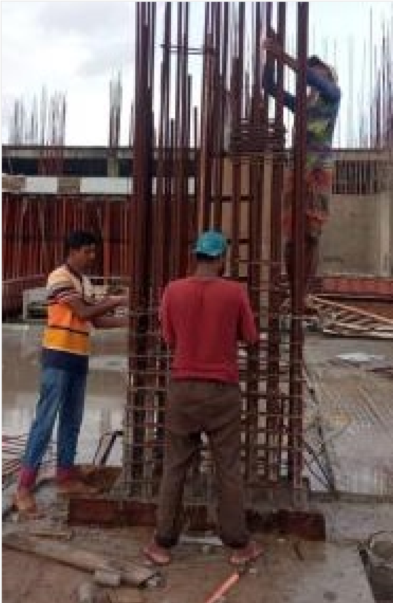
Tower-2-2nd Floor-Column Re-bar Work on 17-10-21
