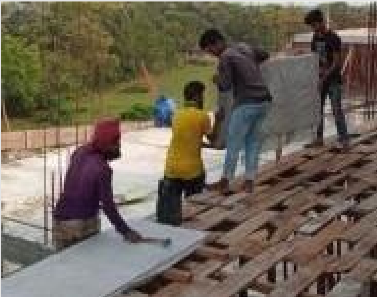
Slab Shuttering on 31-05-21
