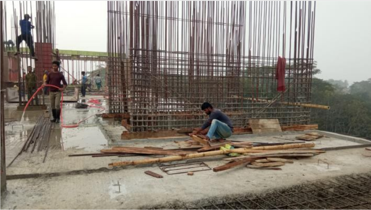
Tower-1-2nd Floor Roof Curing on 25-02-21
