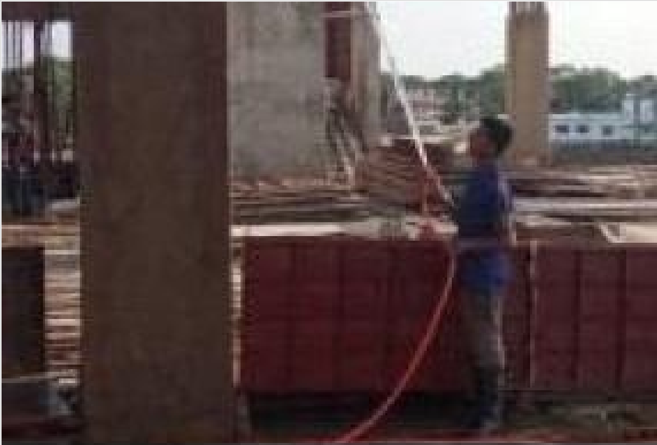
Curing Work on 09-05-21
