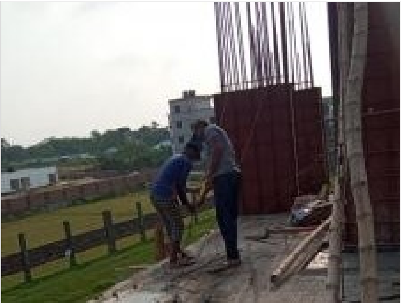
Column Shuttering Work on 30-04-21
