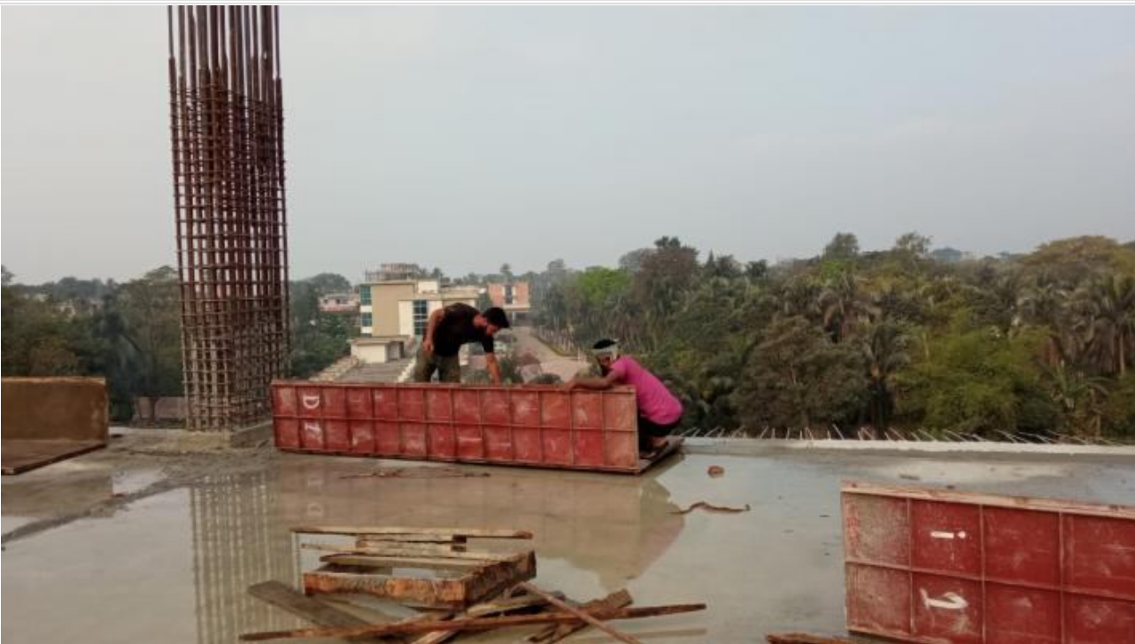
Tower-1-3rd Floor Column Shuttering on 28-02-21
