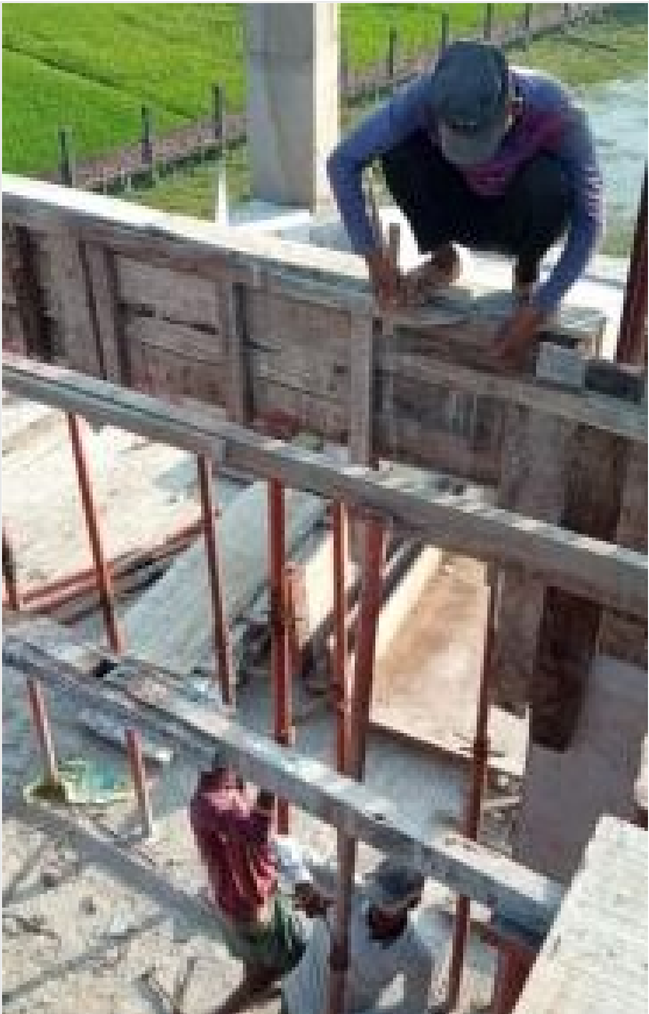
Tower-2-3rd Floor Beam shuttering on 14-11-21
