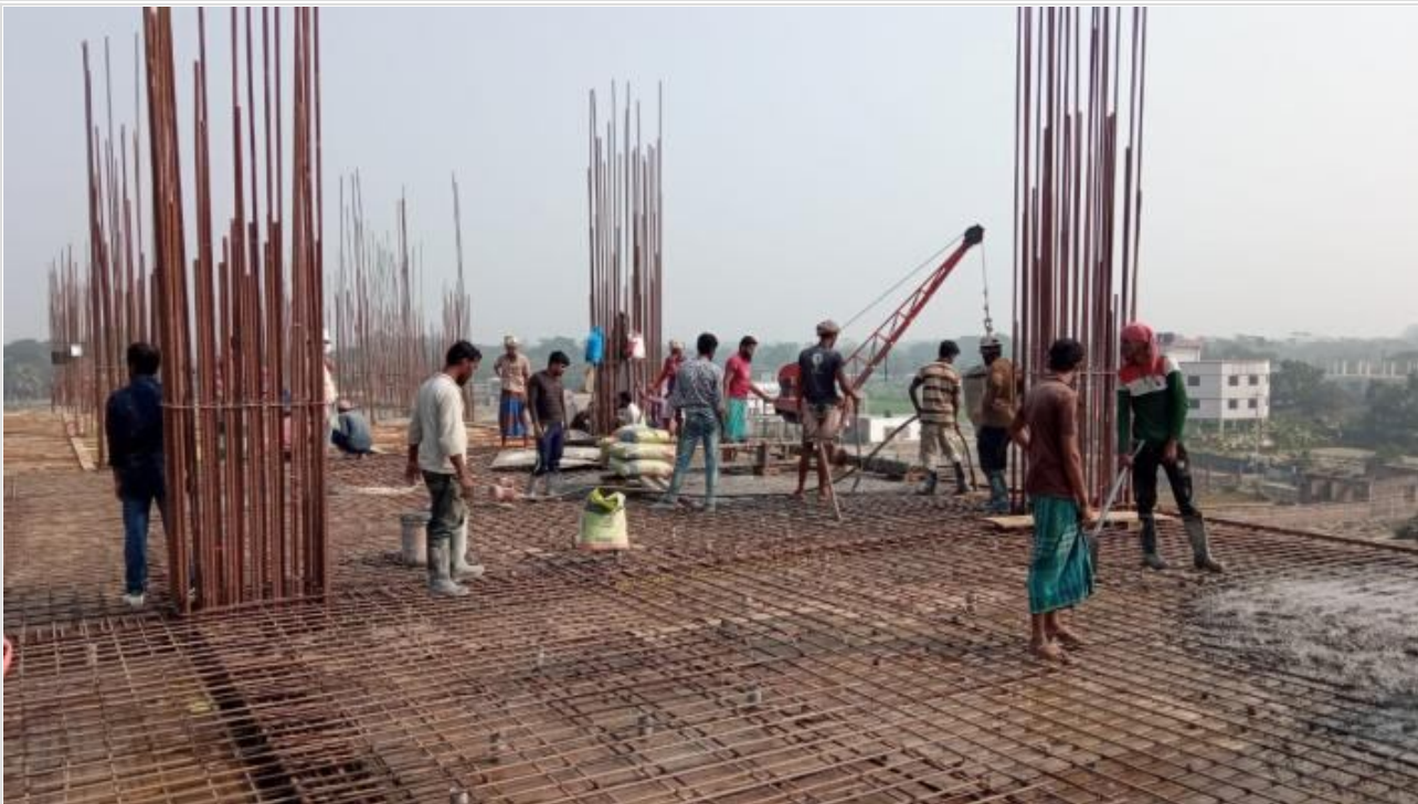
Tower-1-2nd Floor Roof Slab-3600sft Conc on 16-02-21
