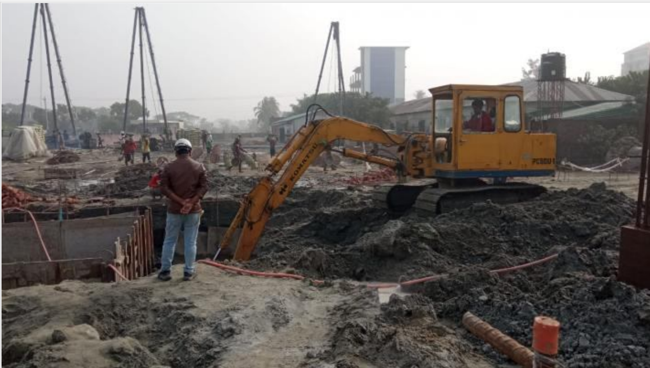
Tower-1-Excavation for Pile Cap on 09-12-20
