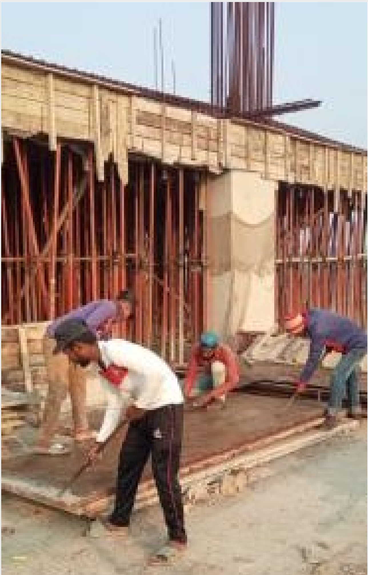
Column/Wall Steel Shutter Cleaning, Oili on 21-02-22
