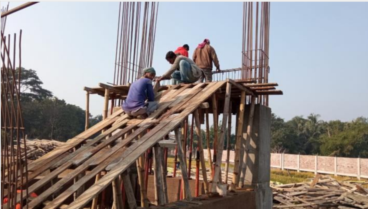
Tower-1-GF Stair Shuttering on 27-12-20
