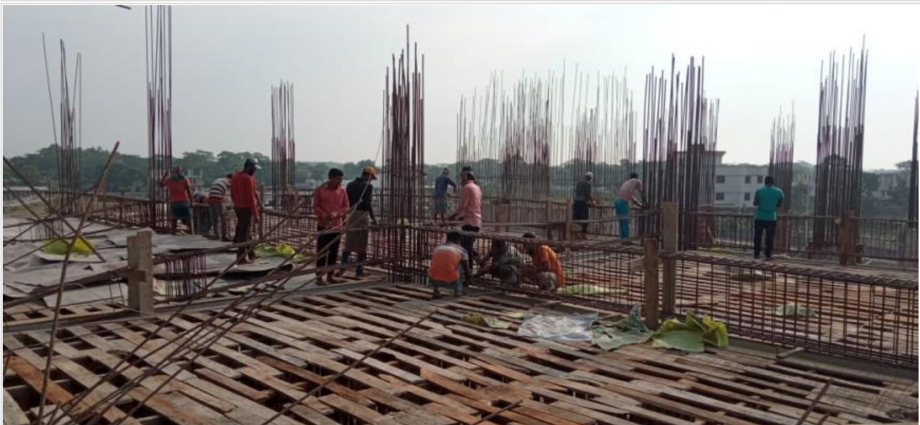
Roof Slab Shuttering on 04-05-21
