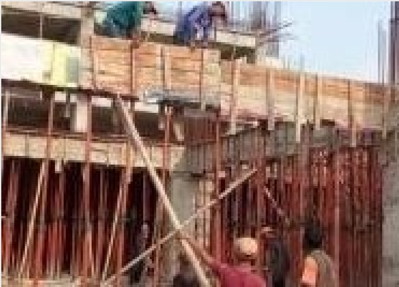
Beam Shuttering on 31-05-21
