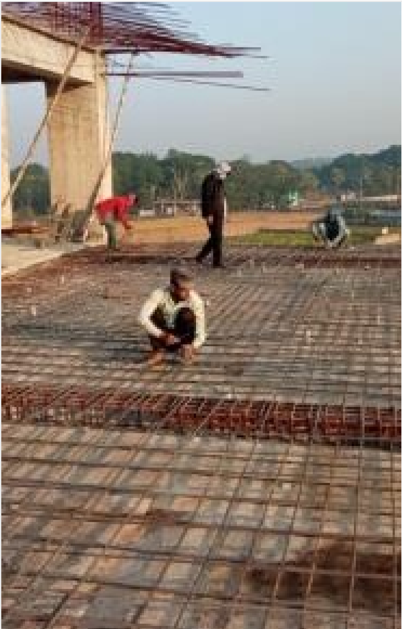
Tower-2:3rd floor slab re-bar work on 31-12-21
