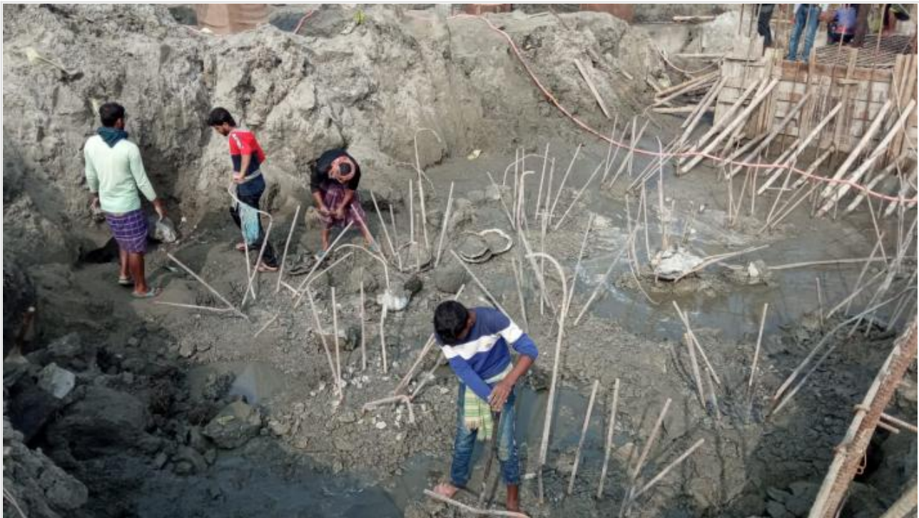
Tower-1-Pile Cap Re-bar Fabrication on 12-12-20
