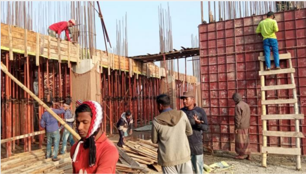
Tower-1-Lift Core and Slab Shuttering on 27-01-21
