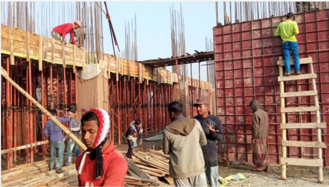
Tower-1-Lift Core and Slab Shuttering on 27-01-21
