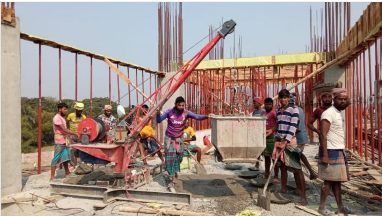
Tower-1-1st Floor Roof Slab 3600 sft Con on 07-02-21
