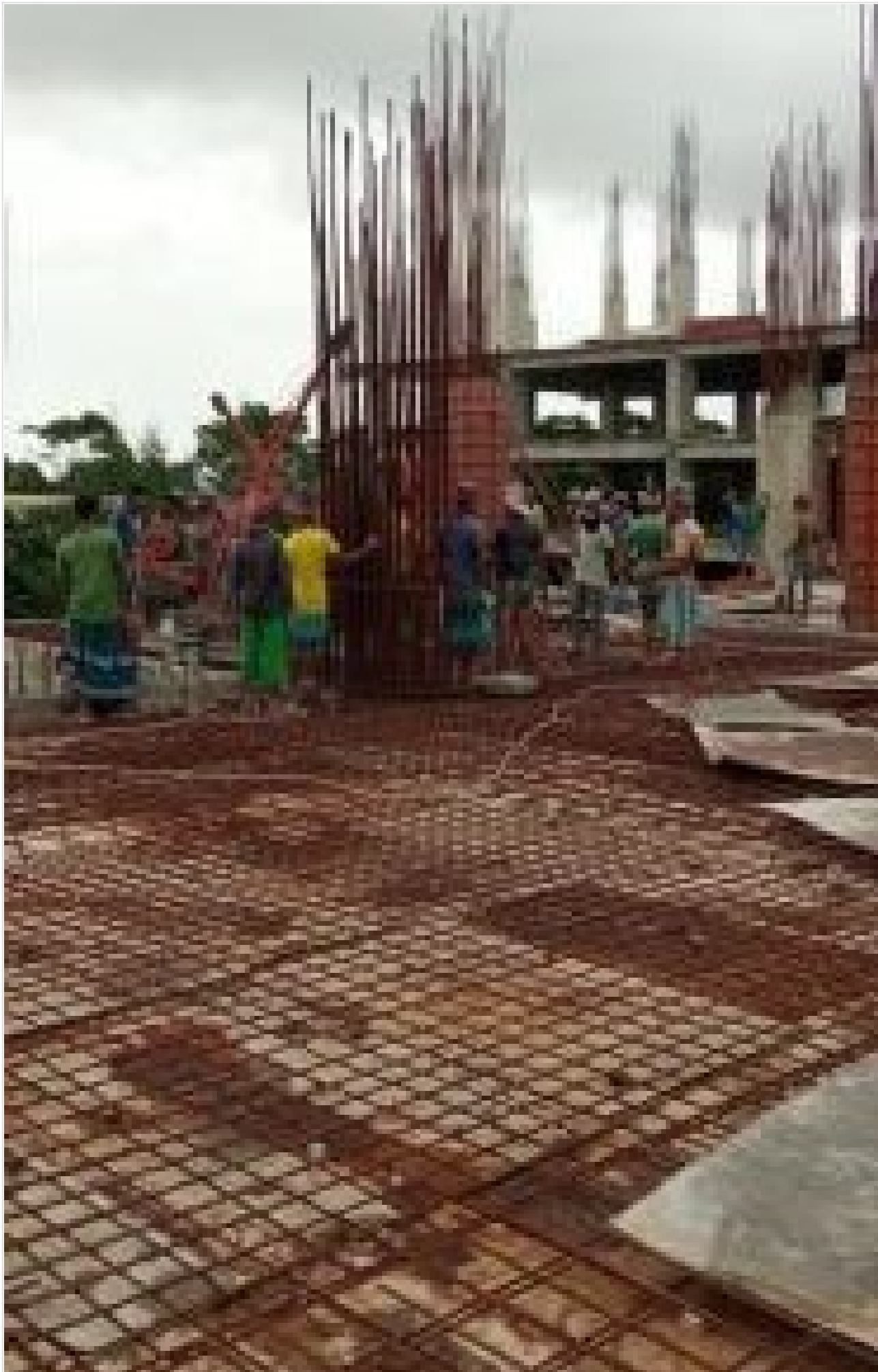
Tower-2:2nd floor slab concreting on 26-09-21
