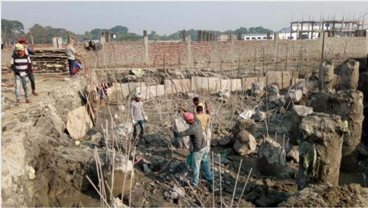
Tower-2-Pile Head Breaking on 27-12-20
