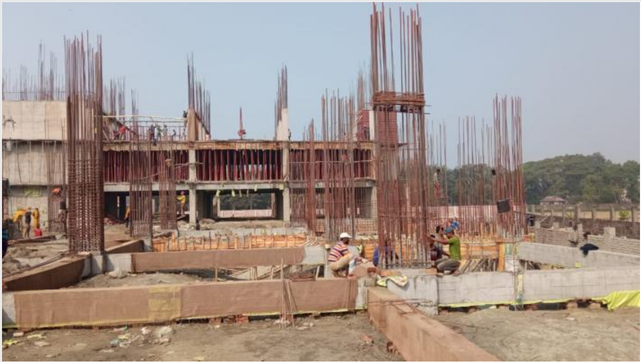
Tower-2-Column Re-bar Work on 16-02-21
