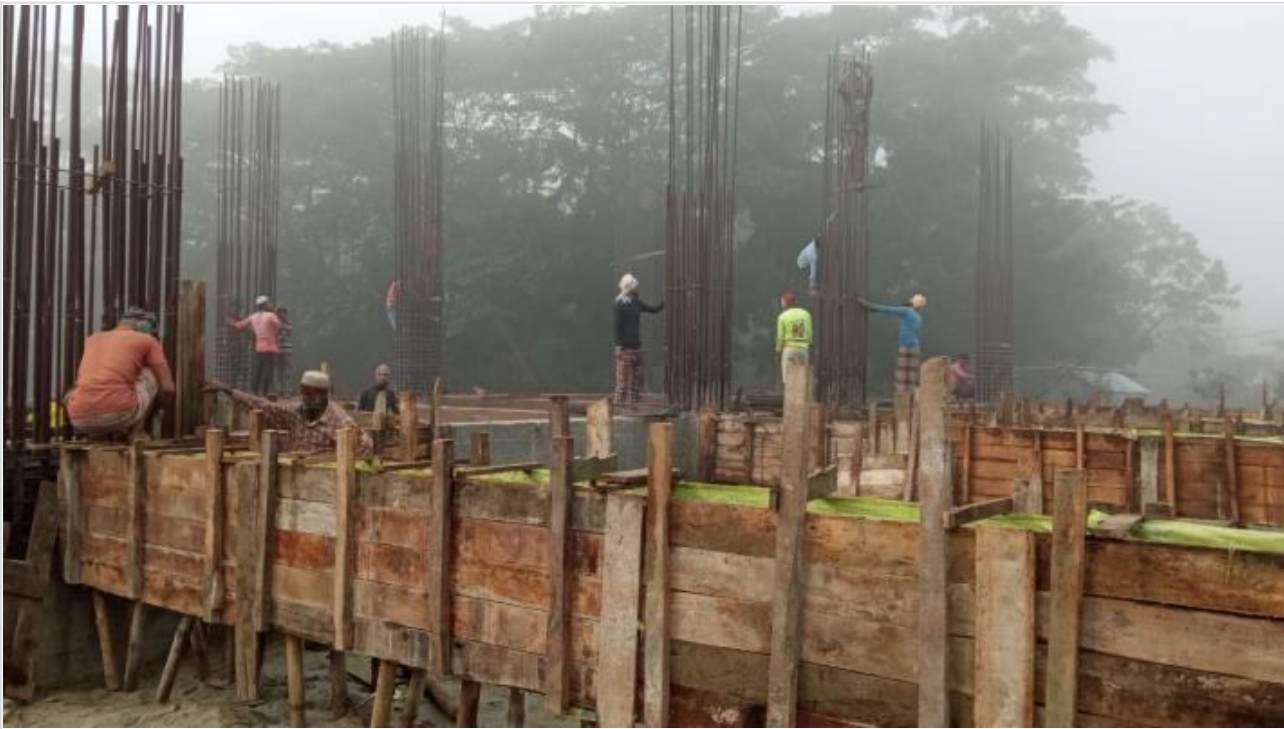
Tower-1 Grade Beam on 07-12-20
