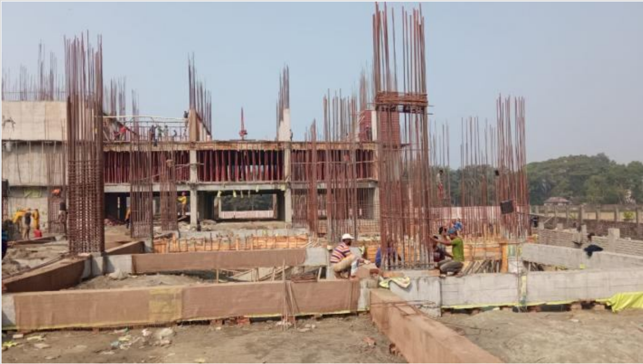
Tower-2-Column Re-bar Work on 16-02-21
