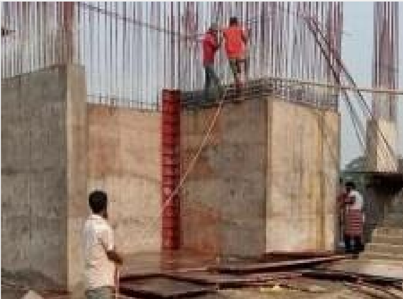
Tower-2: Lift Wall De-shuttering Work on 25-03-21
