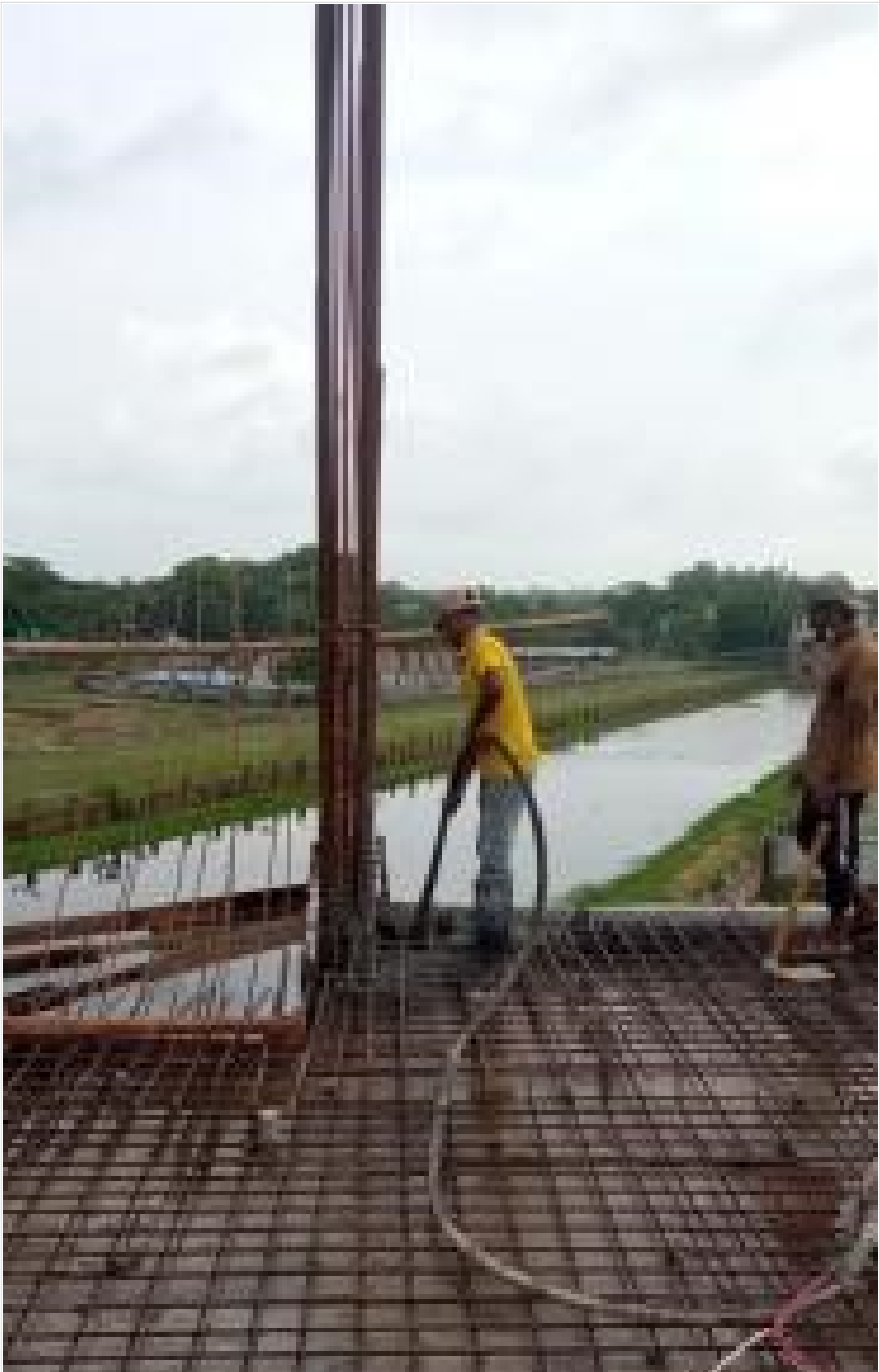
Tower-2:2nd floor slab concreting on 04-07-21
