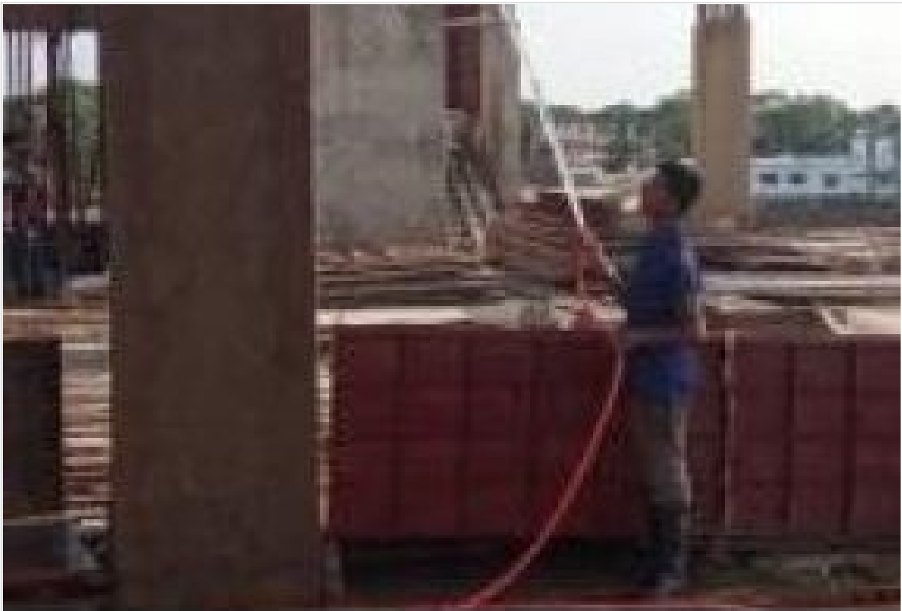
Curing Work on 09-05-21
