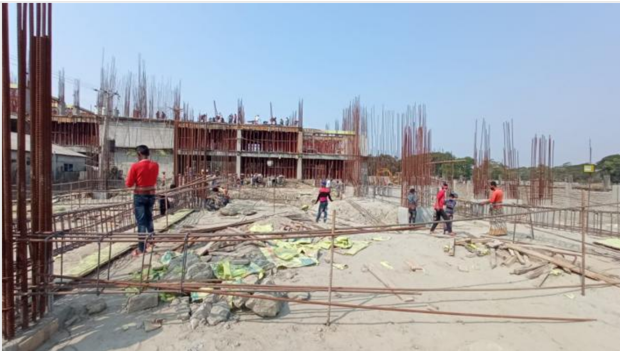
Tower-1-1st Floor Roof Slab Concreting on 07-02-21
