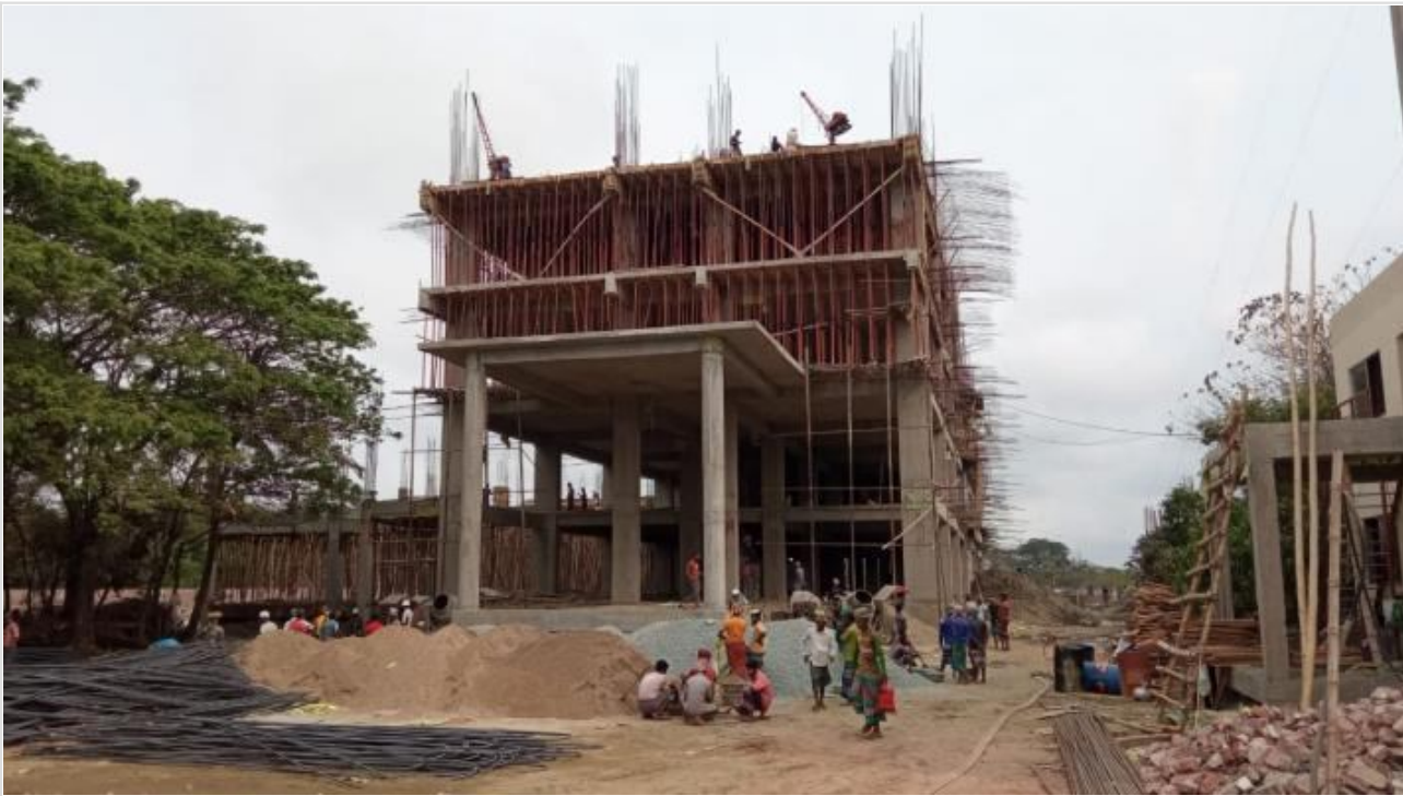
View From South on 11-03-21
