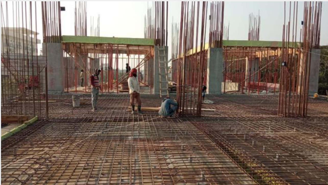
Tower-1-1st Floor Roof Slab 3600 sft Con on 05-02-21
