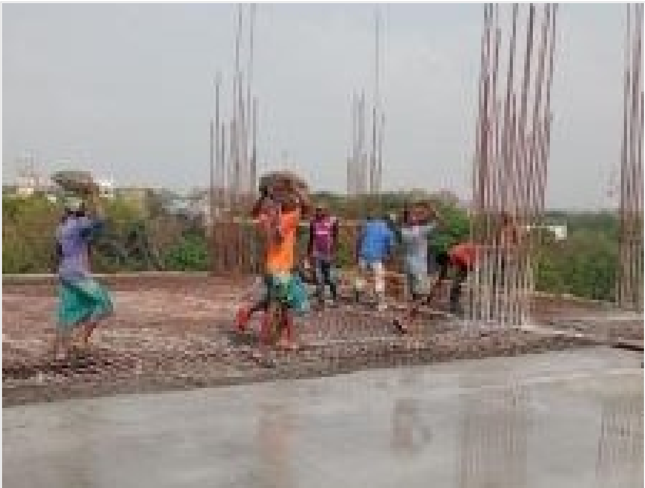
Tower-1-3rd Floor Roof Slab Curing on 01-04-21
