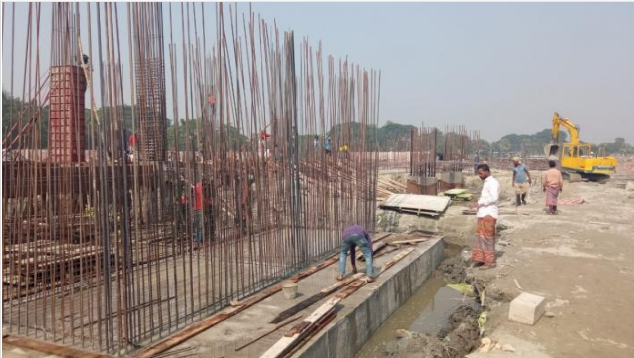
Tower-1-Lift Core Re-bar Work on 20-12-20
