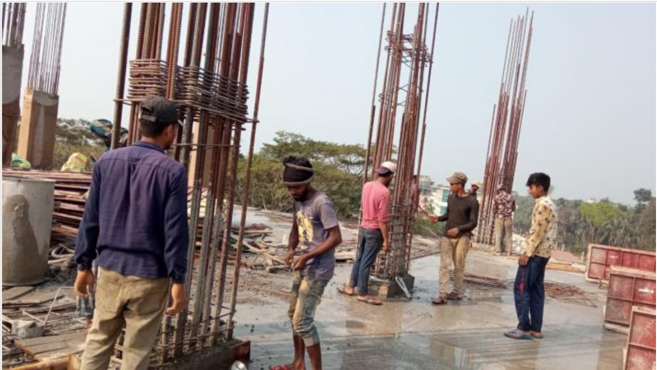
Tower-1-3rd Floor Column Re-bar Work on 23-02-21
