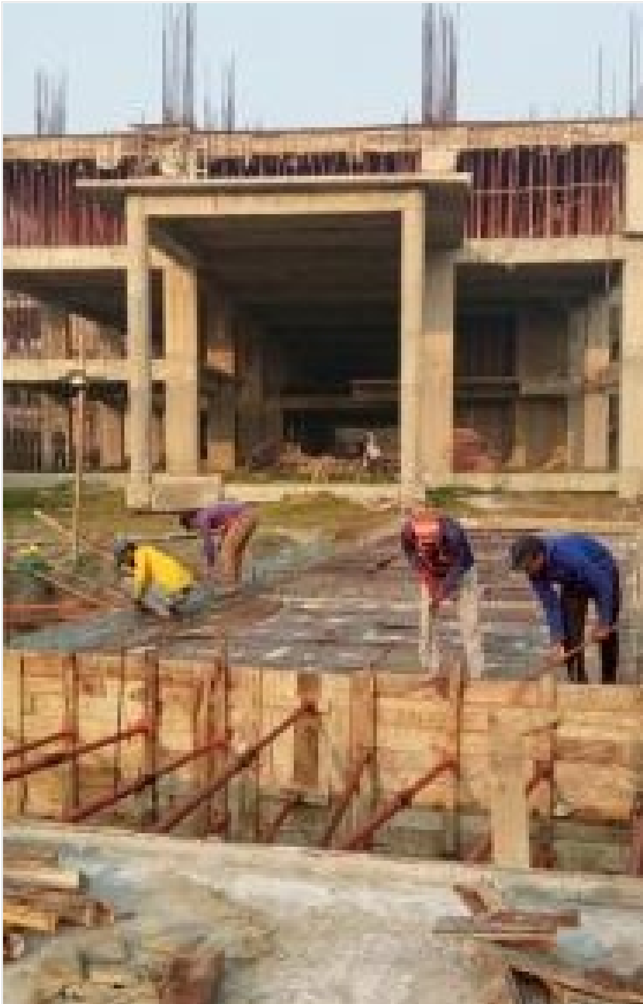
East Septic Tank Slab Shuttering on 10-02-22
