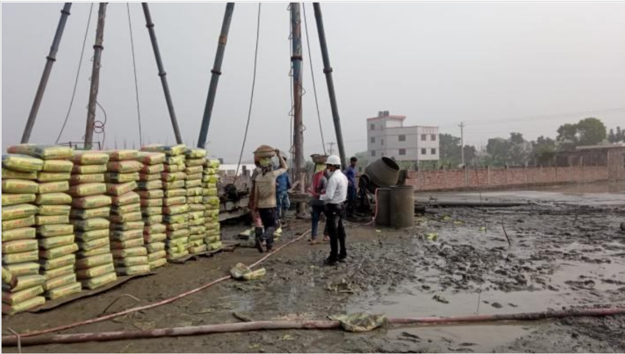
Tower-2-Pile Work on 09-12-20
