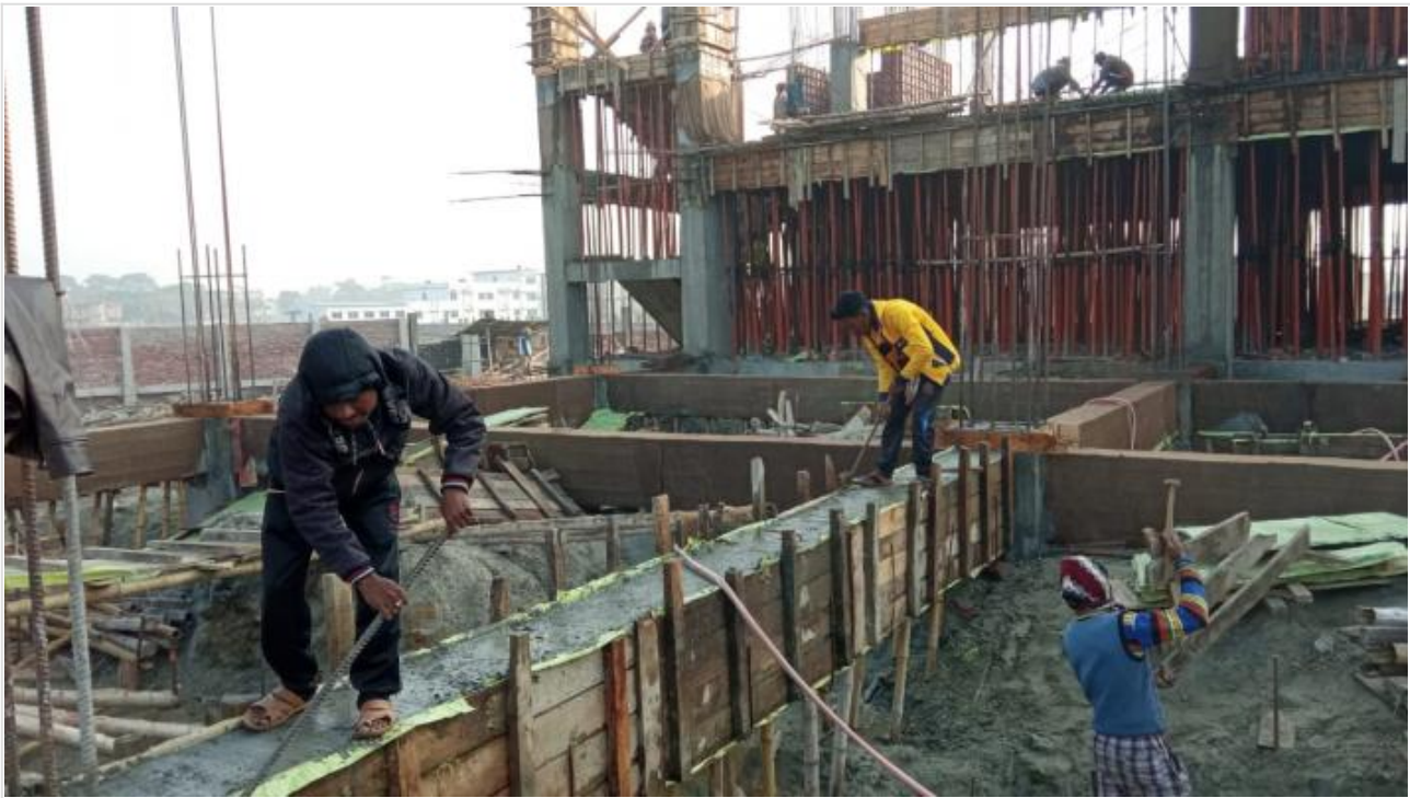
Tower-2-GB Shutter Removing on 05-02-21
