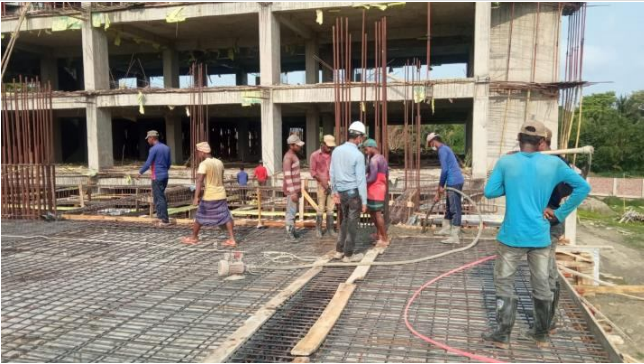
Tower-1-GF Roof Slab(G-I/6-7a)Concreting on 19-04-21
