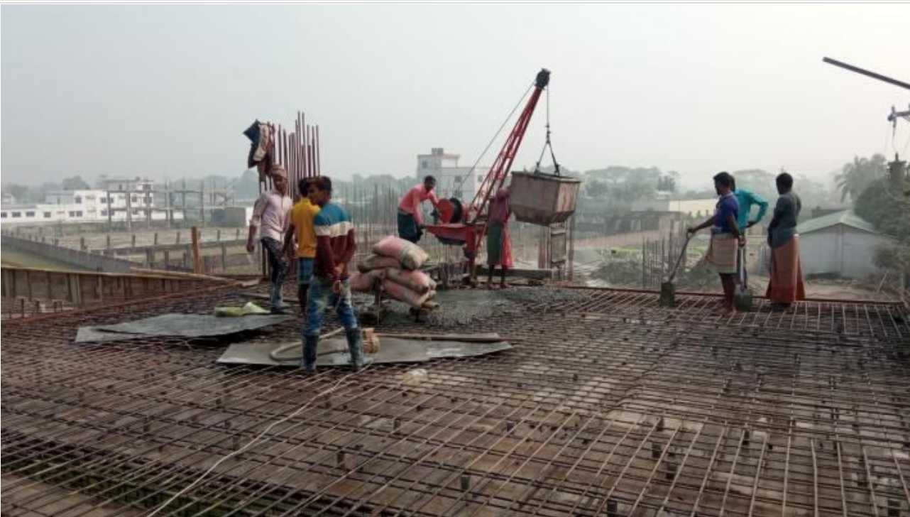
Tower-1-GF Roof Slab 1800 sft Concreting on 18-01-21
