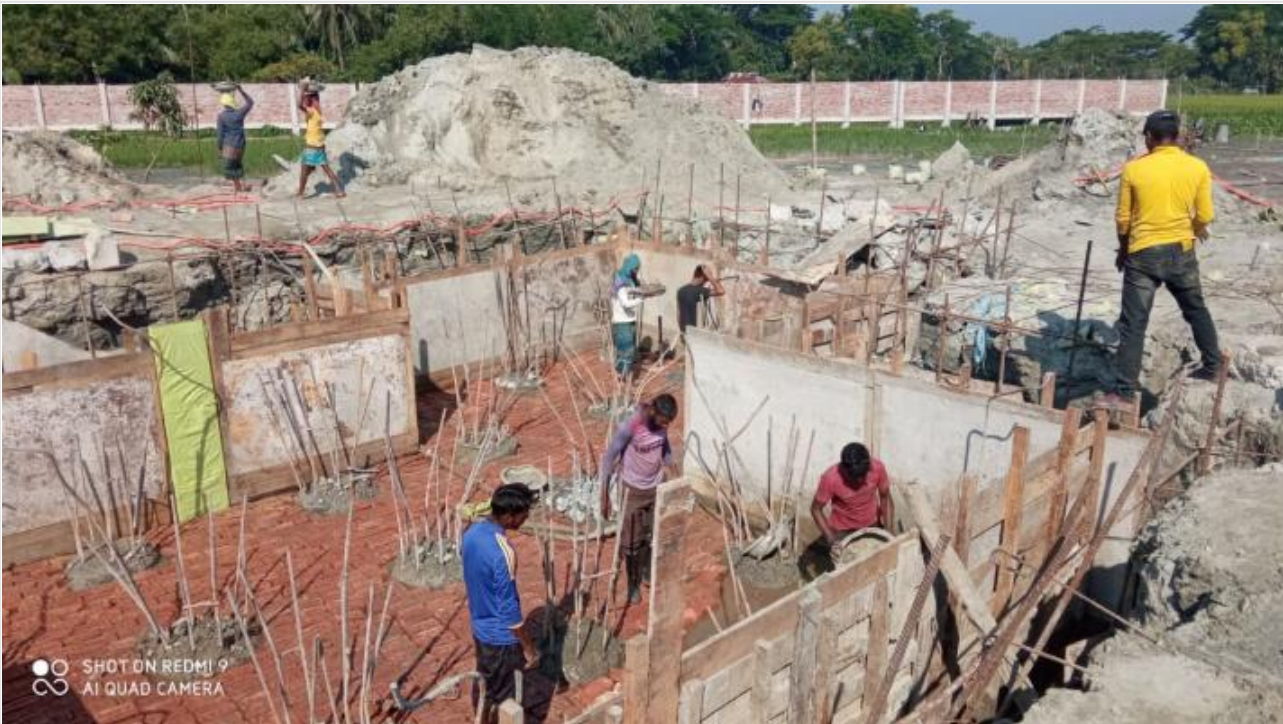
Tower-1-Pile Cap Work on 28-11-20
