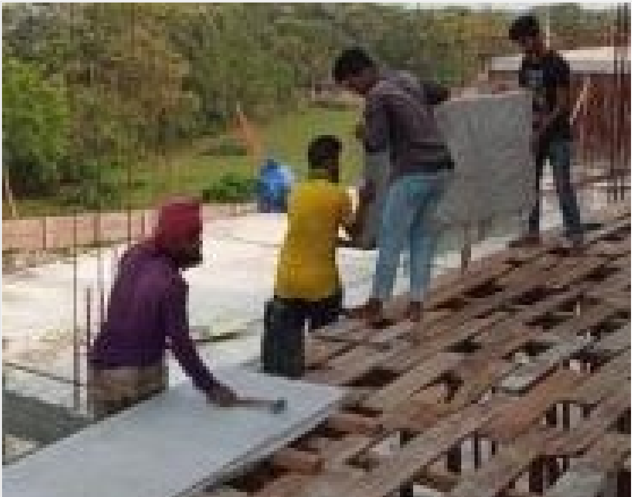
Slab Shuttering on 31-05-21
