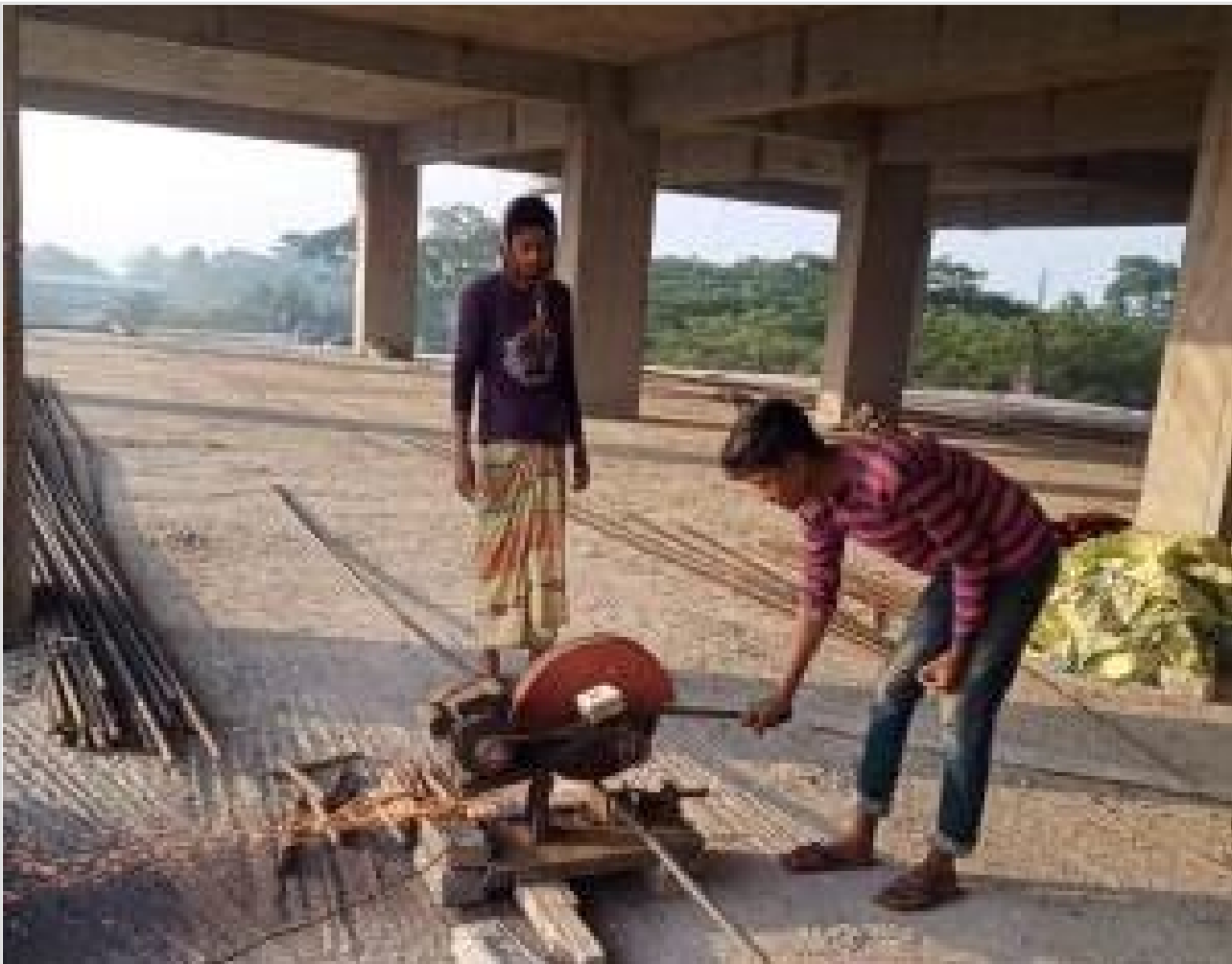
Re-bar Cutting on 08-01-22
