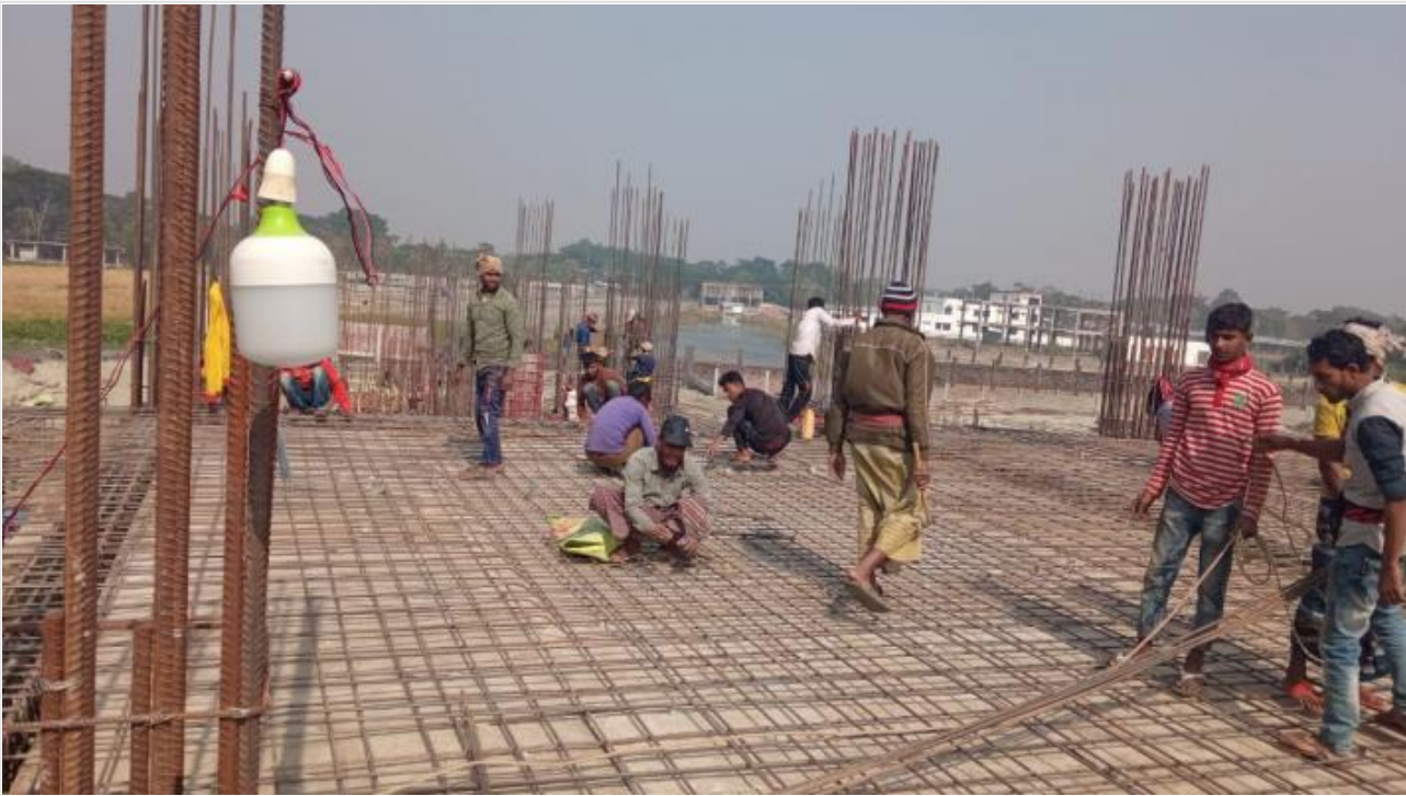
Tower-1-GF Slab Re-bar Work on 20-12-20
