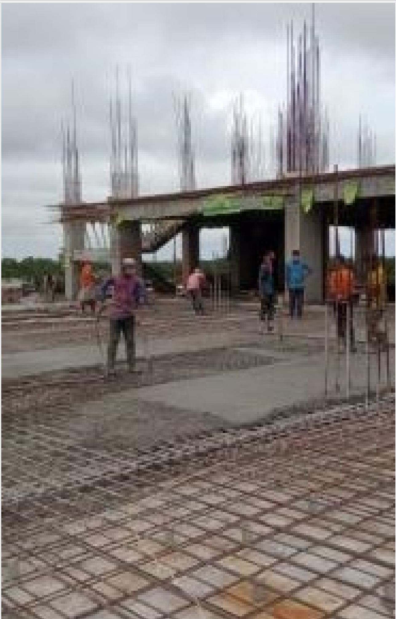
Restaurant-3rd Floor Slab Concreting on 12-06-21
