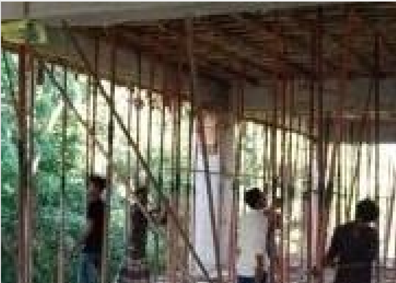
Restaurant GF Double Height Roof Slab on 24-05-21
