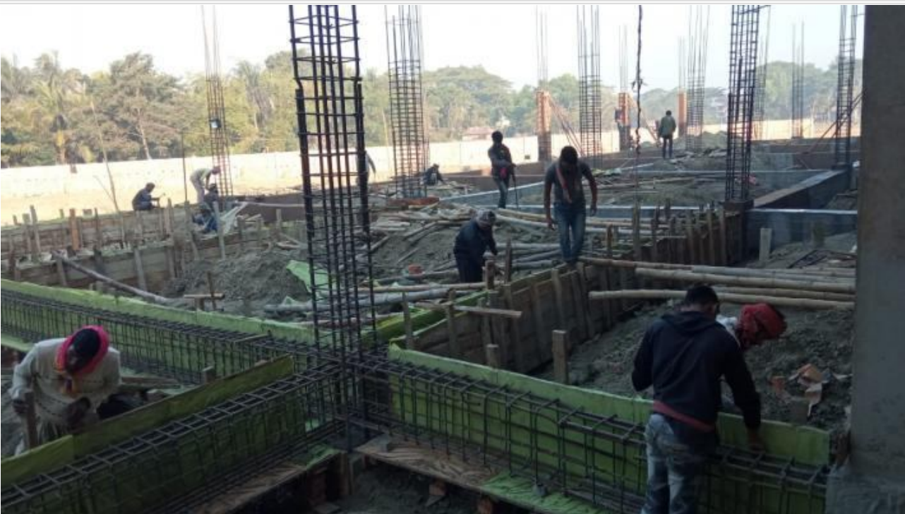
Tower-2-Grade Beam Shuttering on 10-02-21
