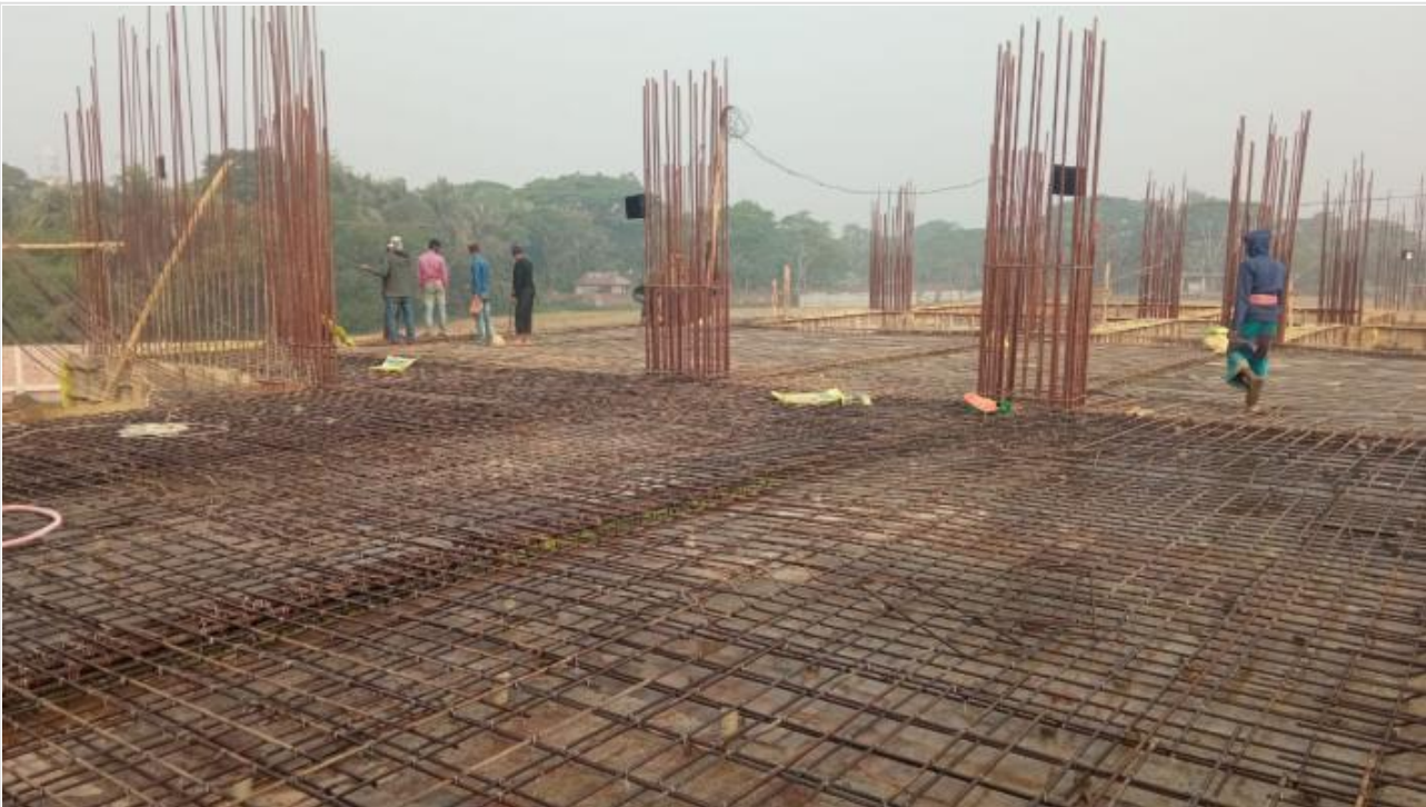
Tower-1-GF Roof Slab-3600sft Concreting on 16-01-21
