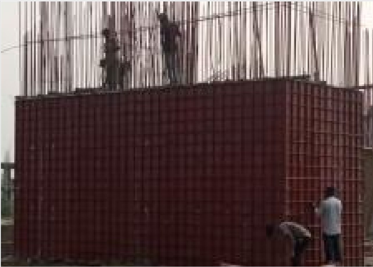
Lift Core Wall Shuttering on 24-03-21
