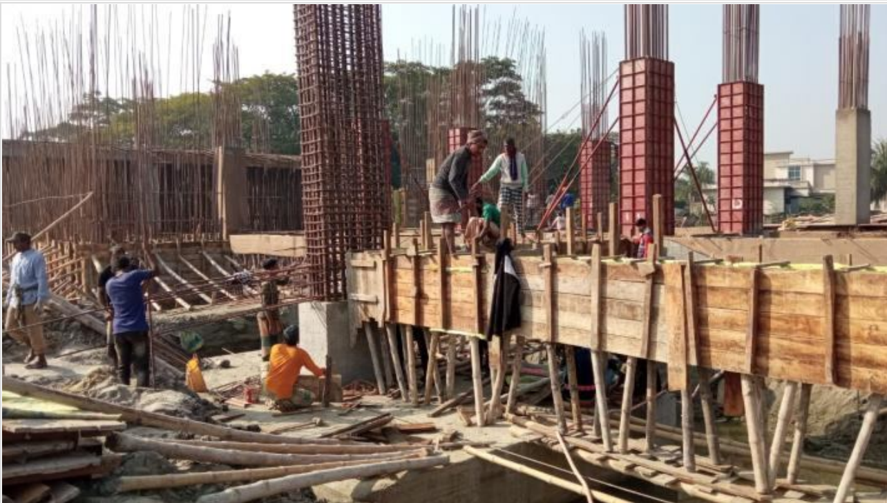
Tower-1-Grade Beam Shuttering on 24-12-20
