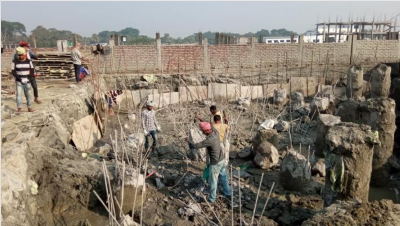
Tower-2-Pile Head Breaking on 27-12-20
