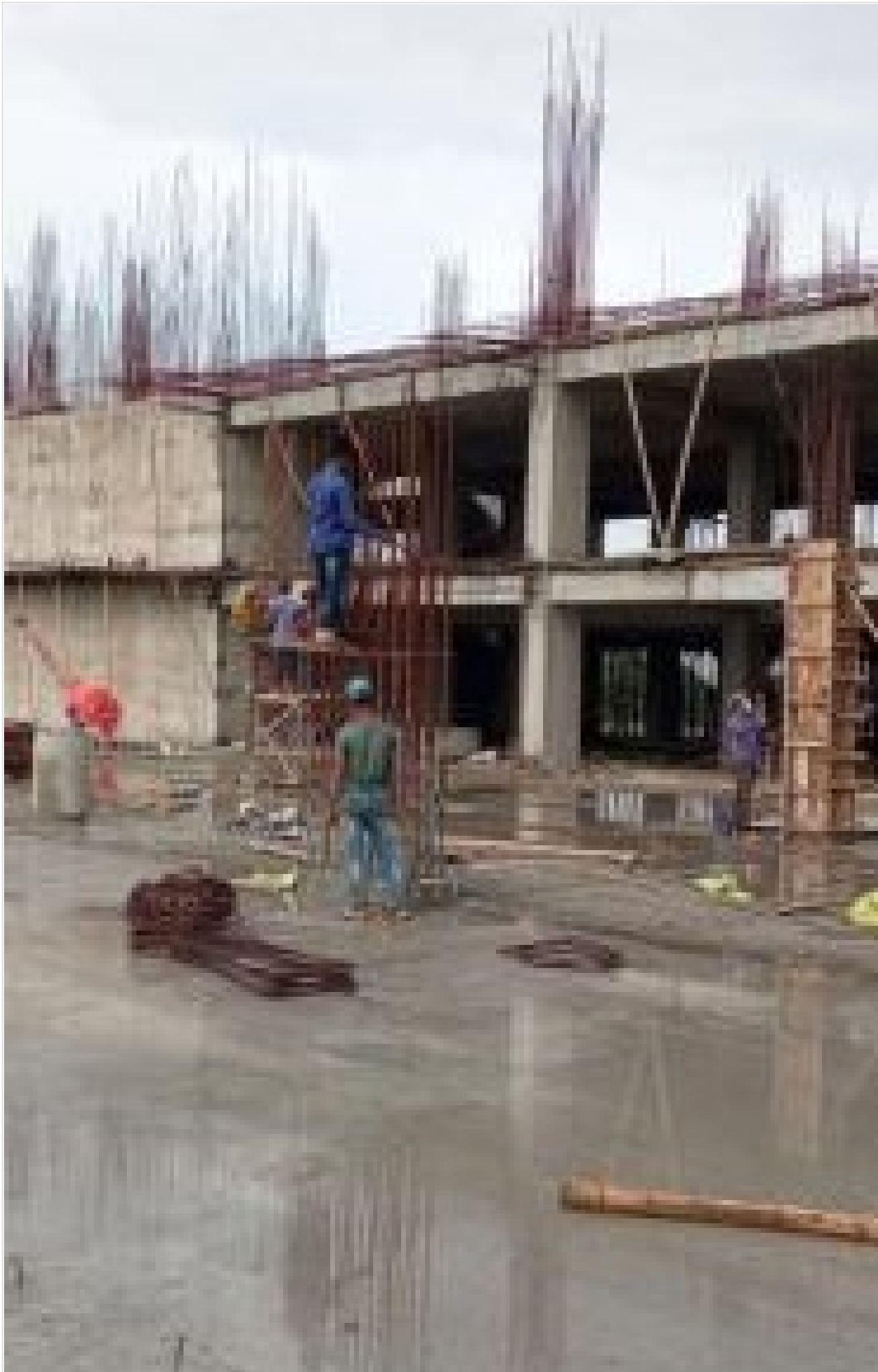
Tower-2-Column Rod binding-shuttering on 05-07-21
