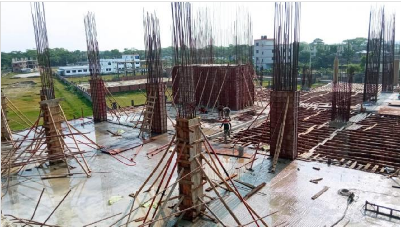
Column Concreting on 28-04-21
