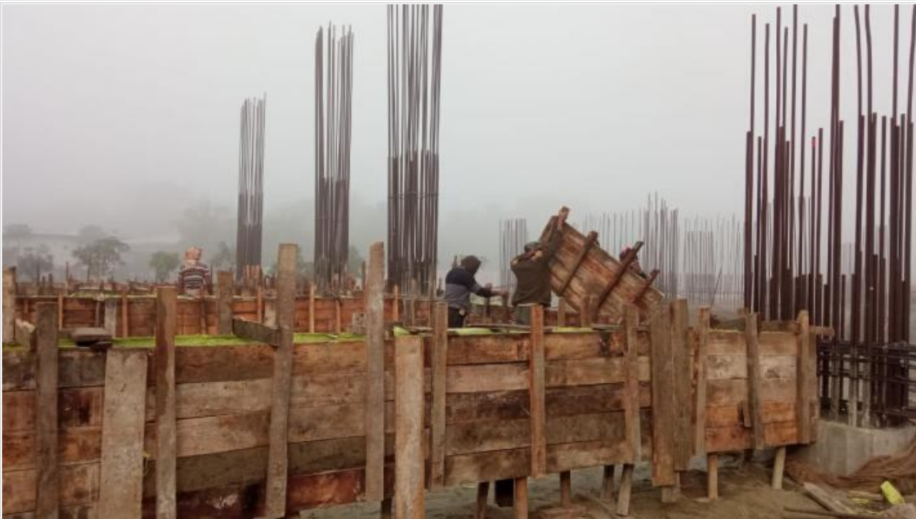
Tower-1-Grade Beam on 04-12-20
