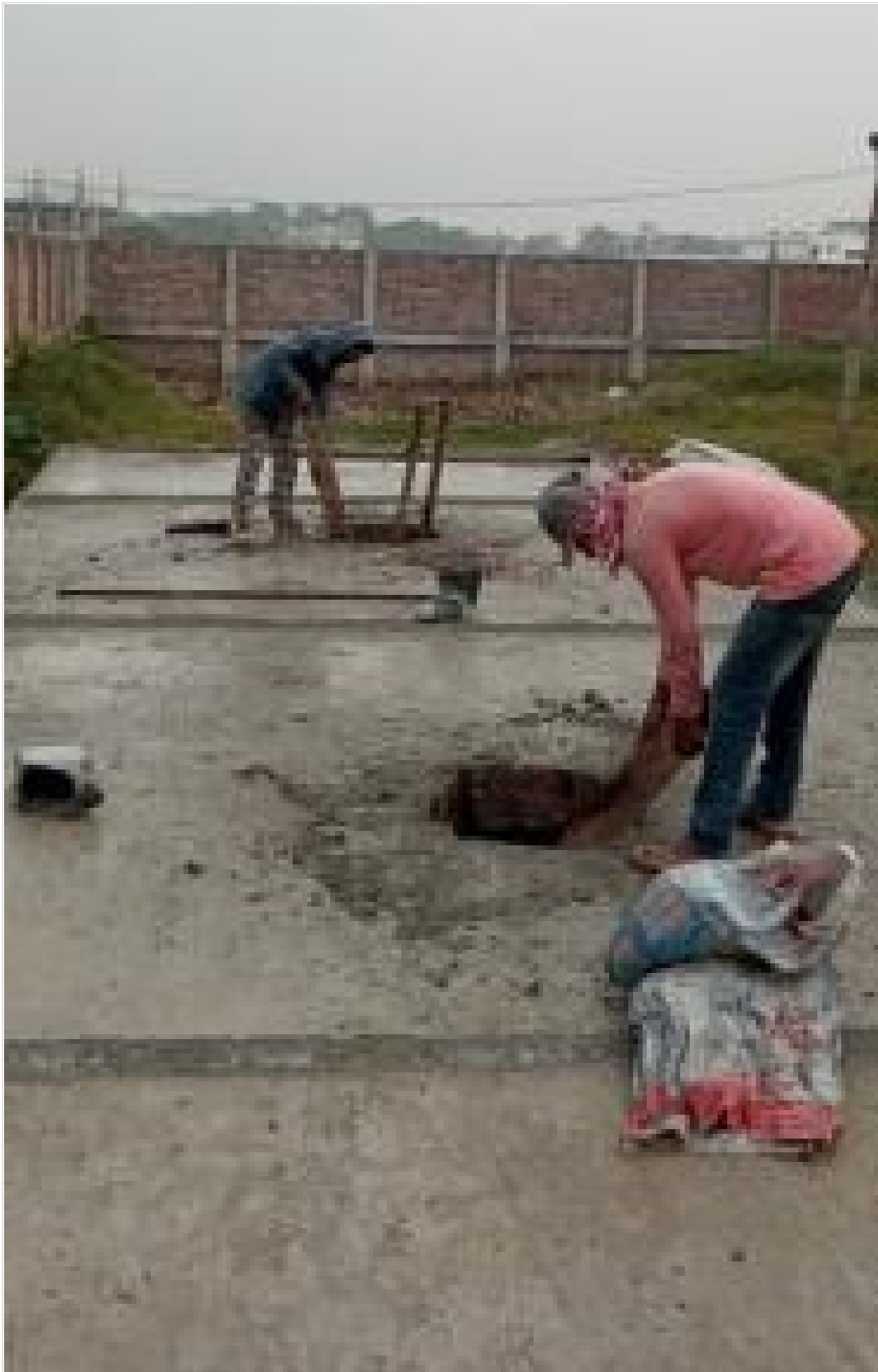
Soak Well Slab Concreted on 27-01-22
