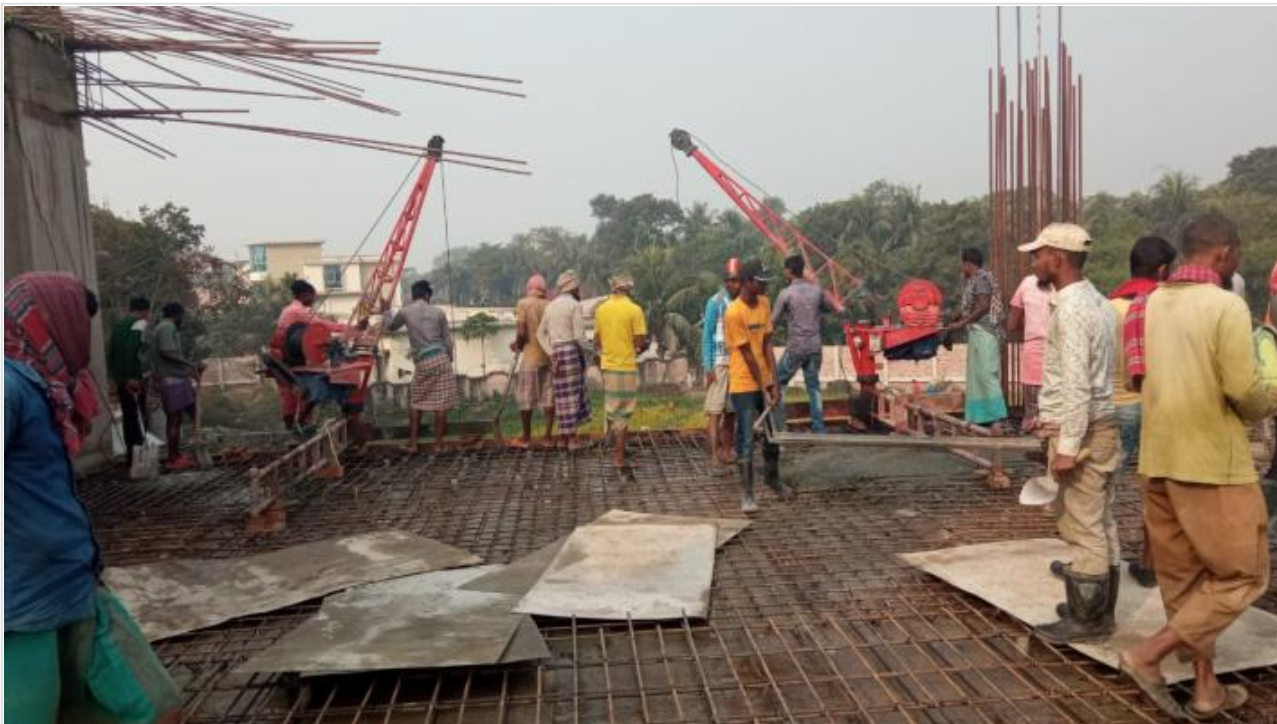
Tower-1-GF Roof Slab Concreting on 16-01-21
