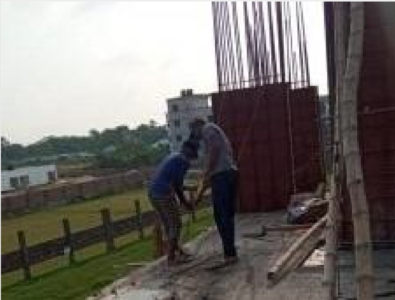
Column Shuttering Work on 30-04-21
