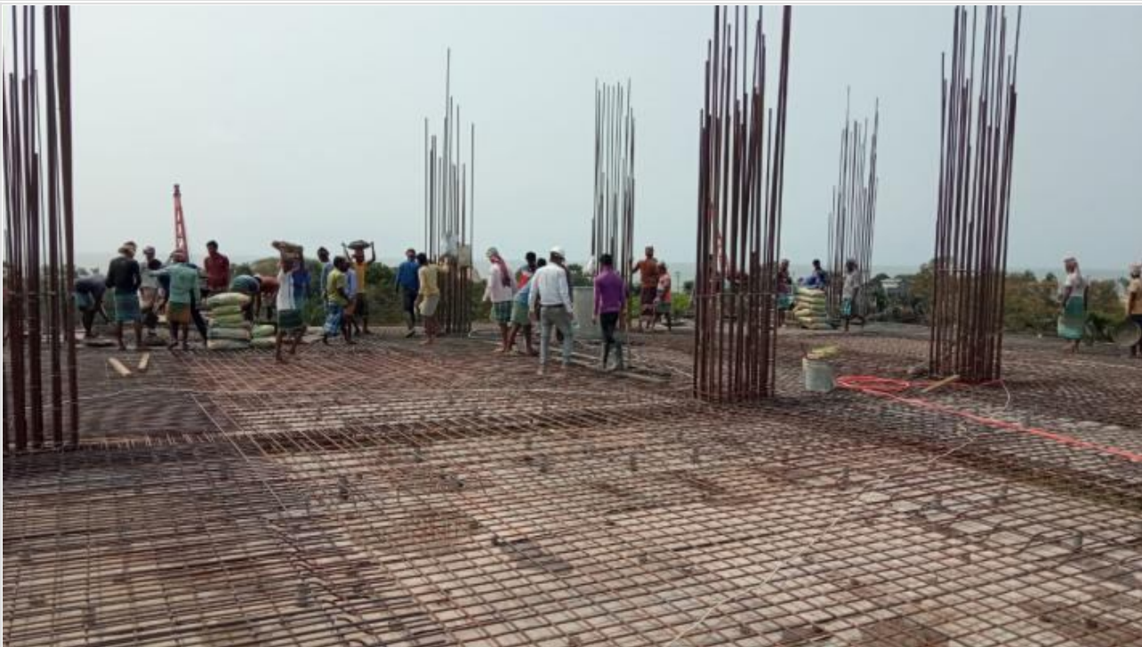
Tower-1-3rd Floor Roof Slab Concreting on 11-03-21
