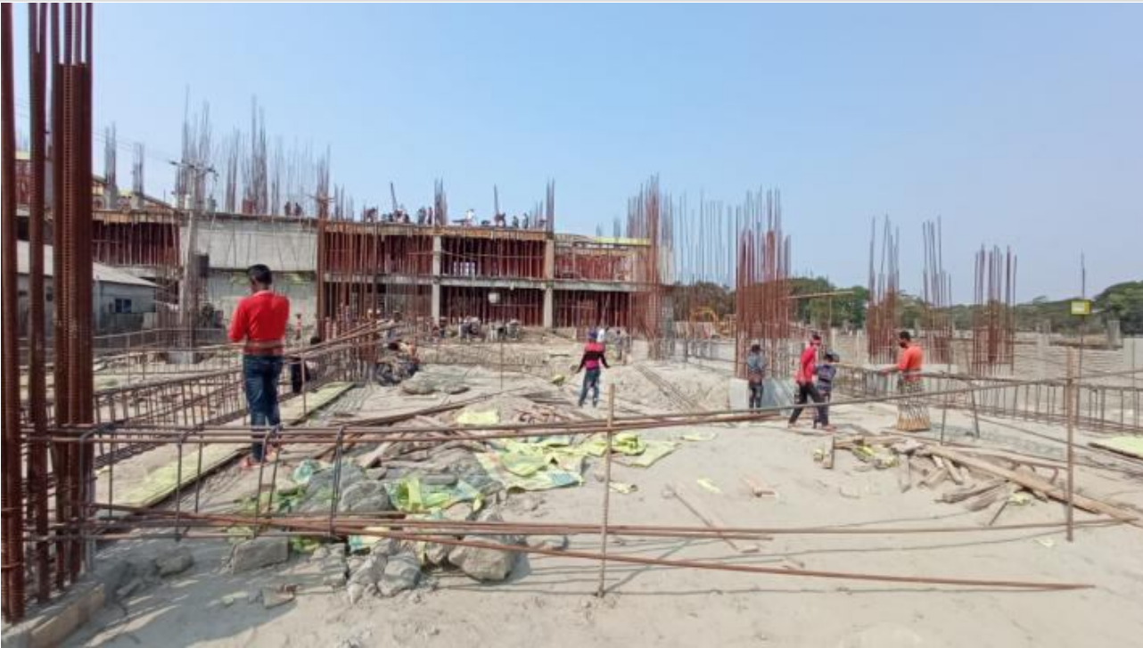
Tower-1-1st Floor Roof Slab Concreting on 07-02-21
