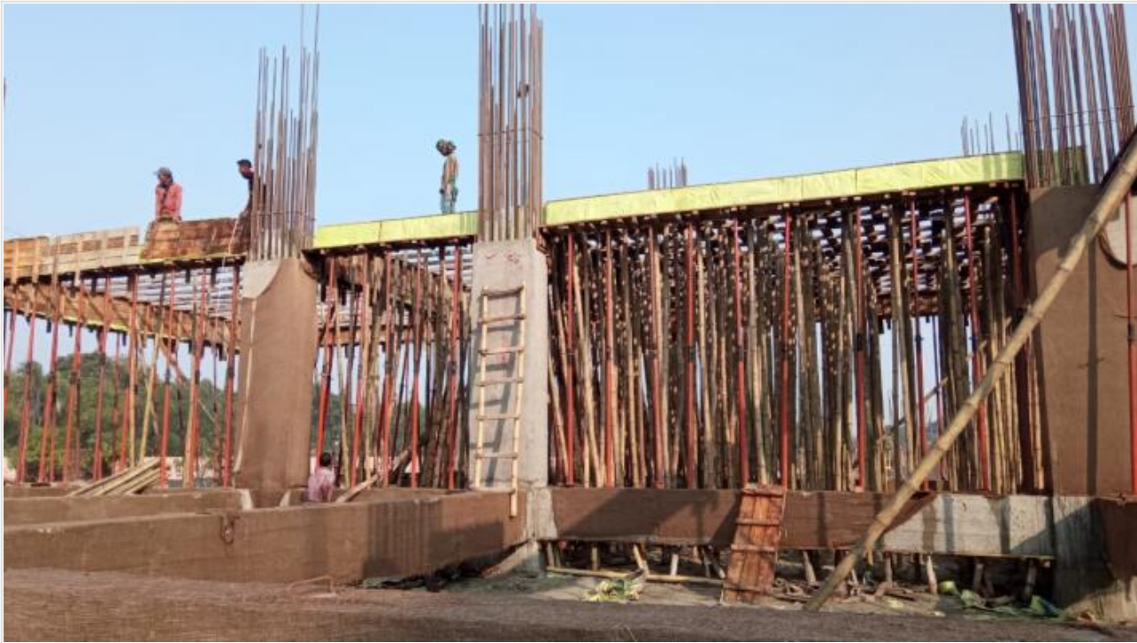
Tower-1-GF Beam Shuttering on 18-12-20
