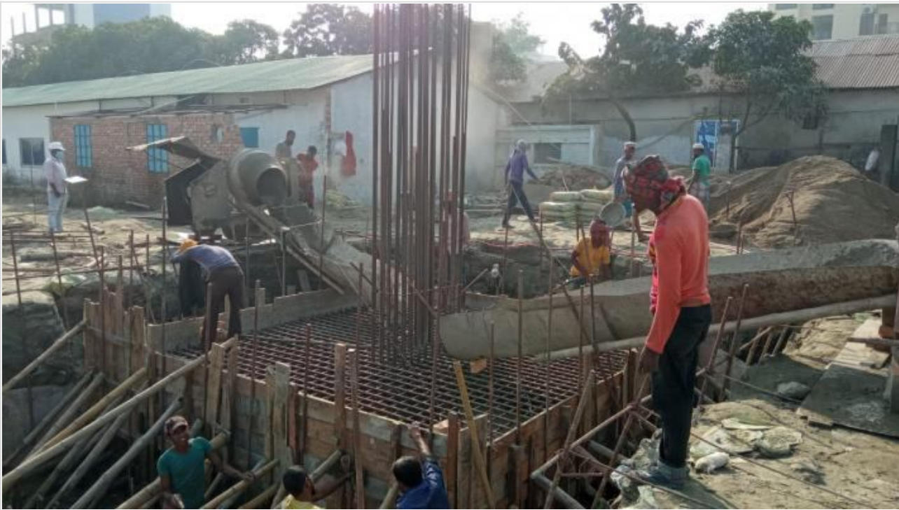
Tower-2-Pile Cap Concreting on 08-01-21
