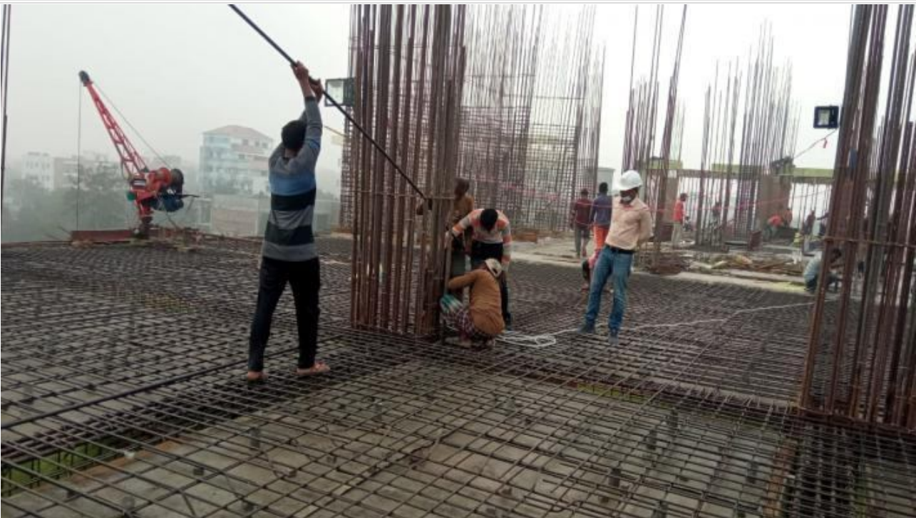
Tower-1-2nd Floor Roof Inspection on 25-02-21
