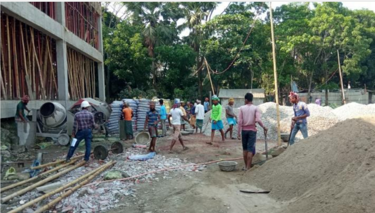
Restaurant GF Doubl Ht Slab-1-4/A-B-Conc on 24-04-21
