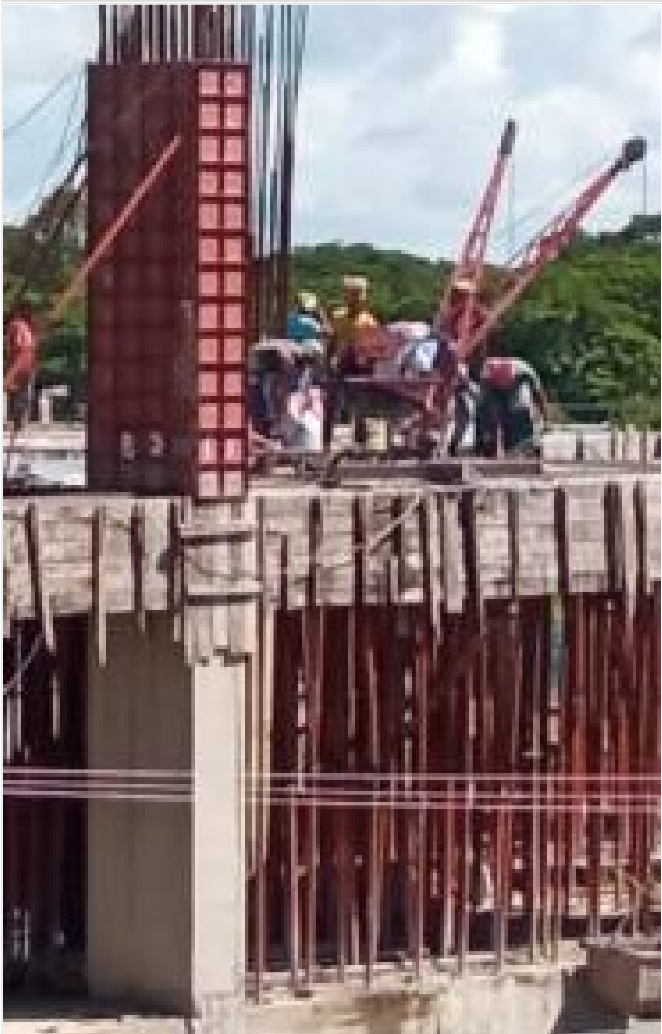
Tower-2-2nd Floor-Column Concreting on 30-09-21
