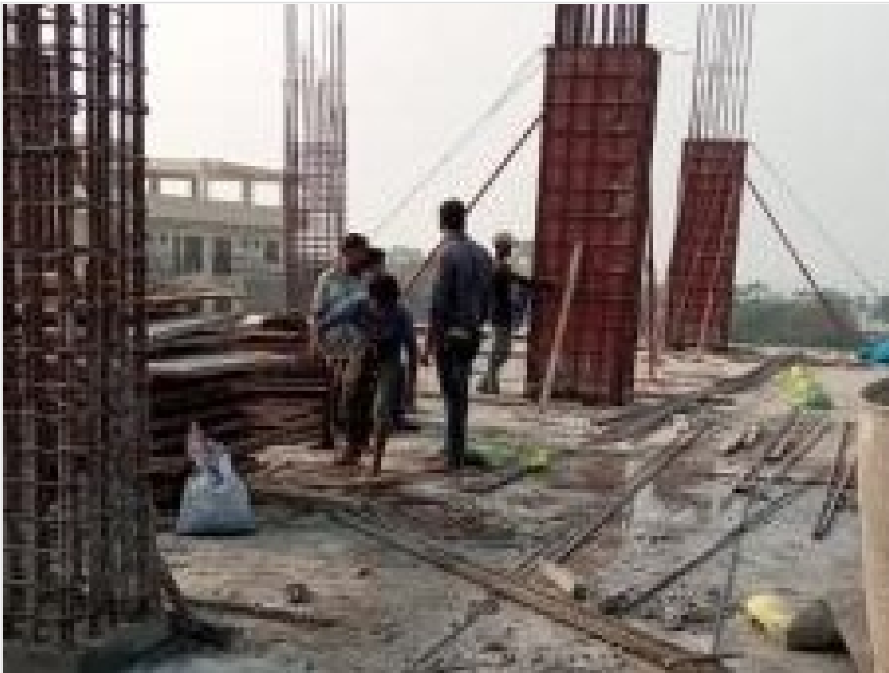
Column Shuttering Work on 25-03-21
