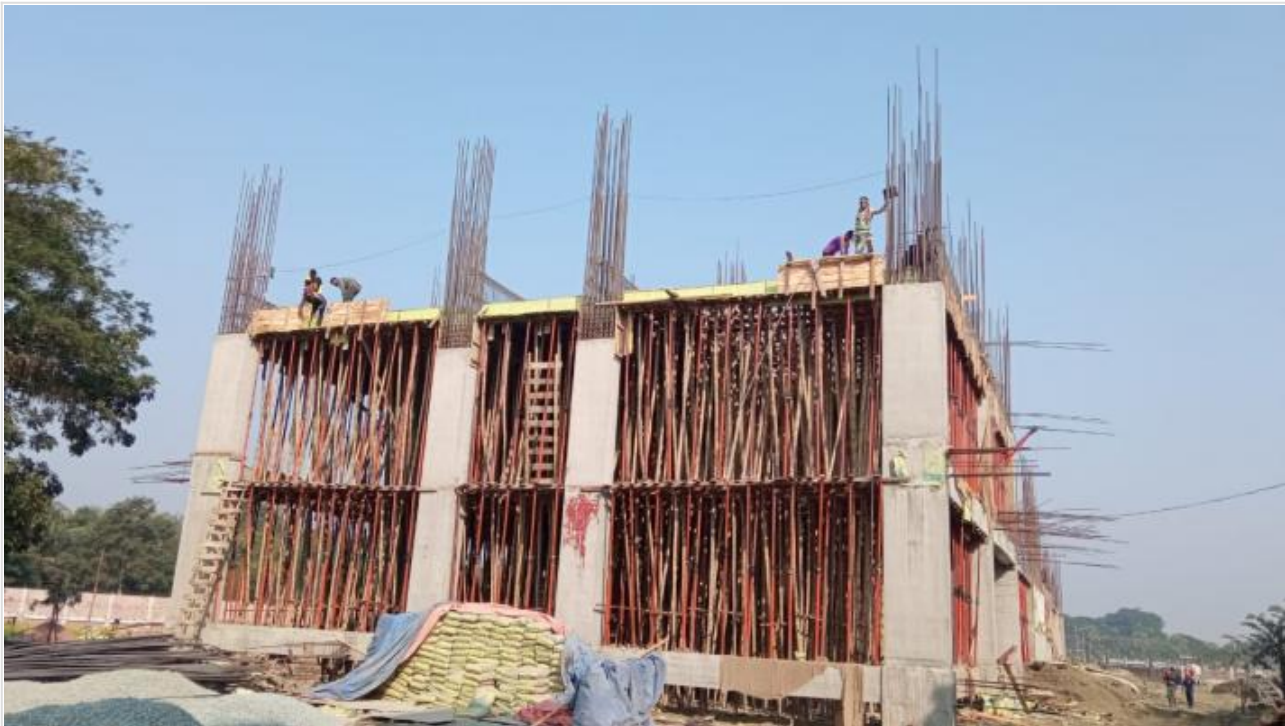
Tower-1-1st Floor Roof Slab Shuttering on 08-01-21
