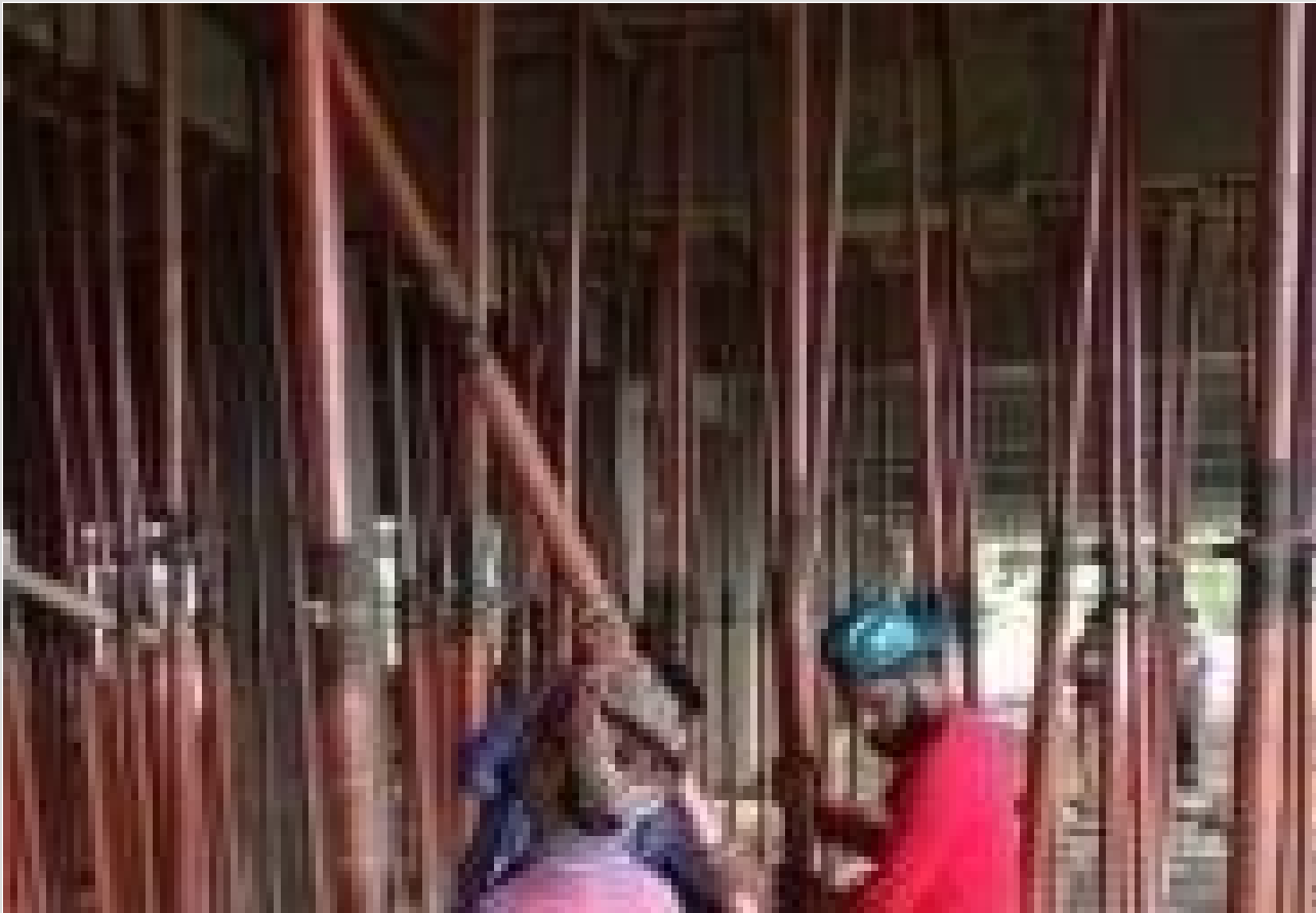
Roof Slab De-shuttering on 24-05-21
