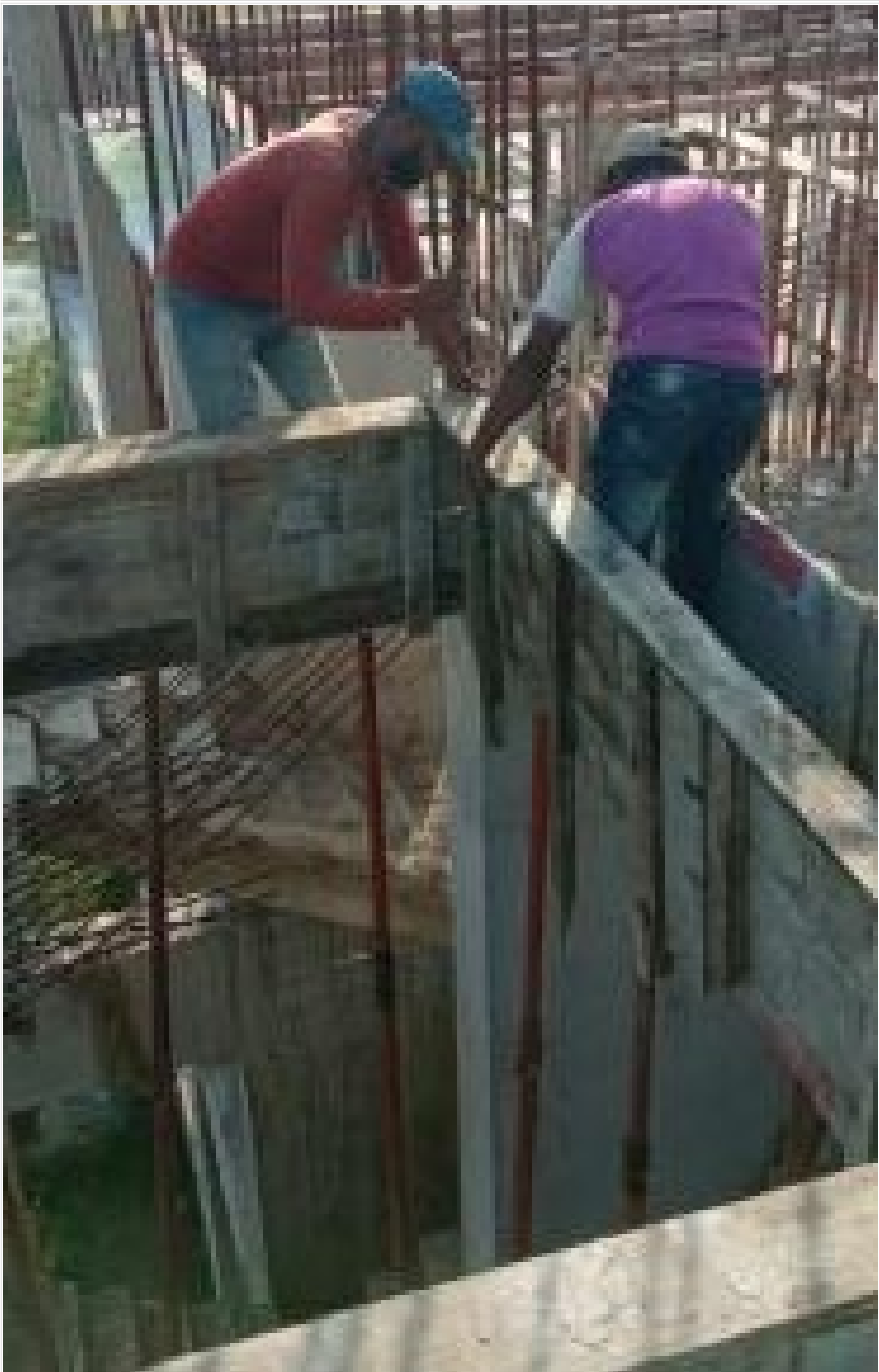
Tower-2-3rd Floor Beam shuttering on 14-11-21
