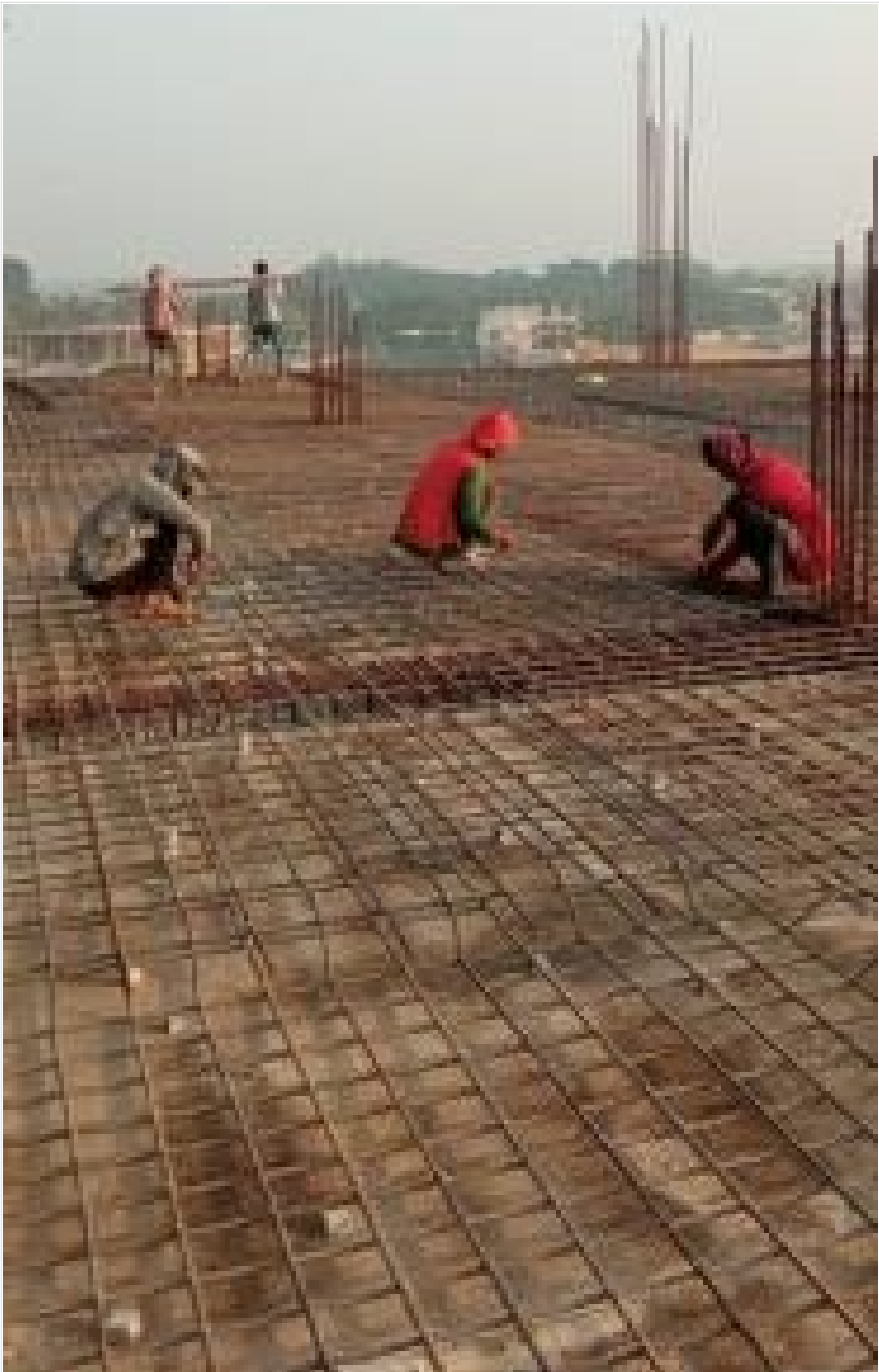
Tower-2-3rd Floor-Re-bar Work on 01-01-22
