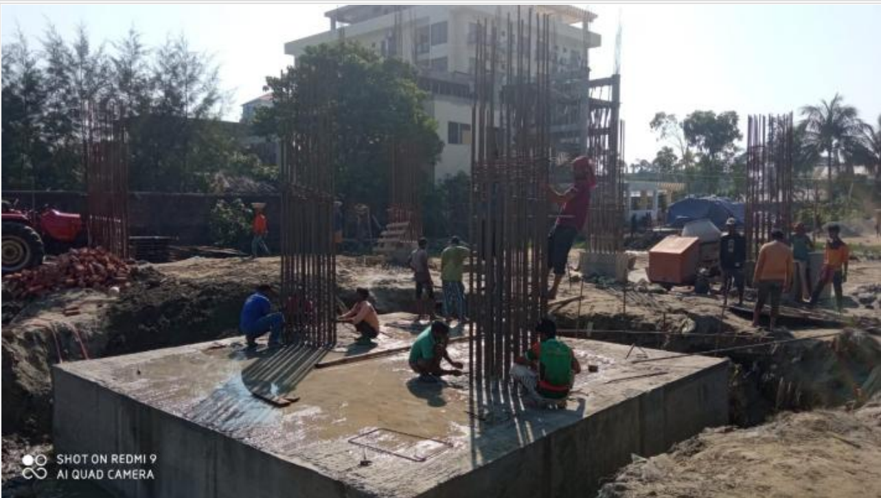
Tower-1 Pile Cap on 30-11-20
