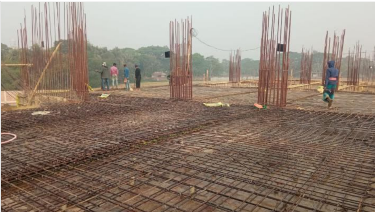
Tower-1-GF Roof Slab-3600sft Concreting on 16-01-21
