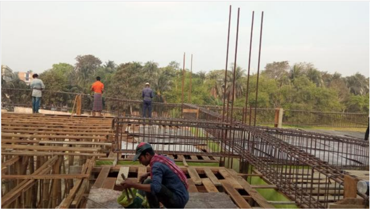
Resturant Area Slab Shuttering on 28-02-21
