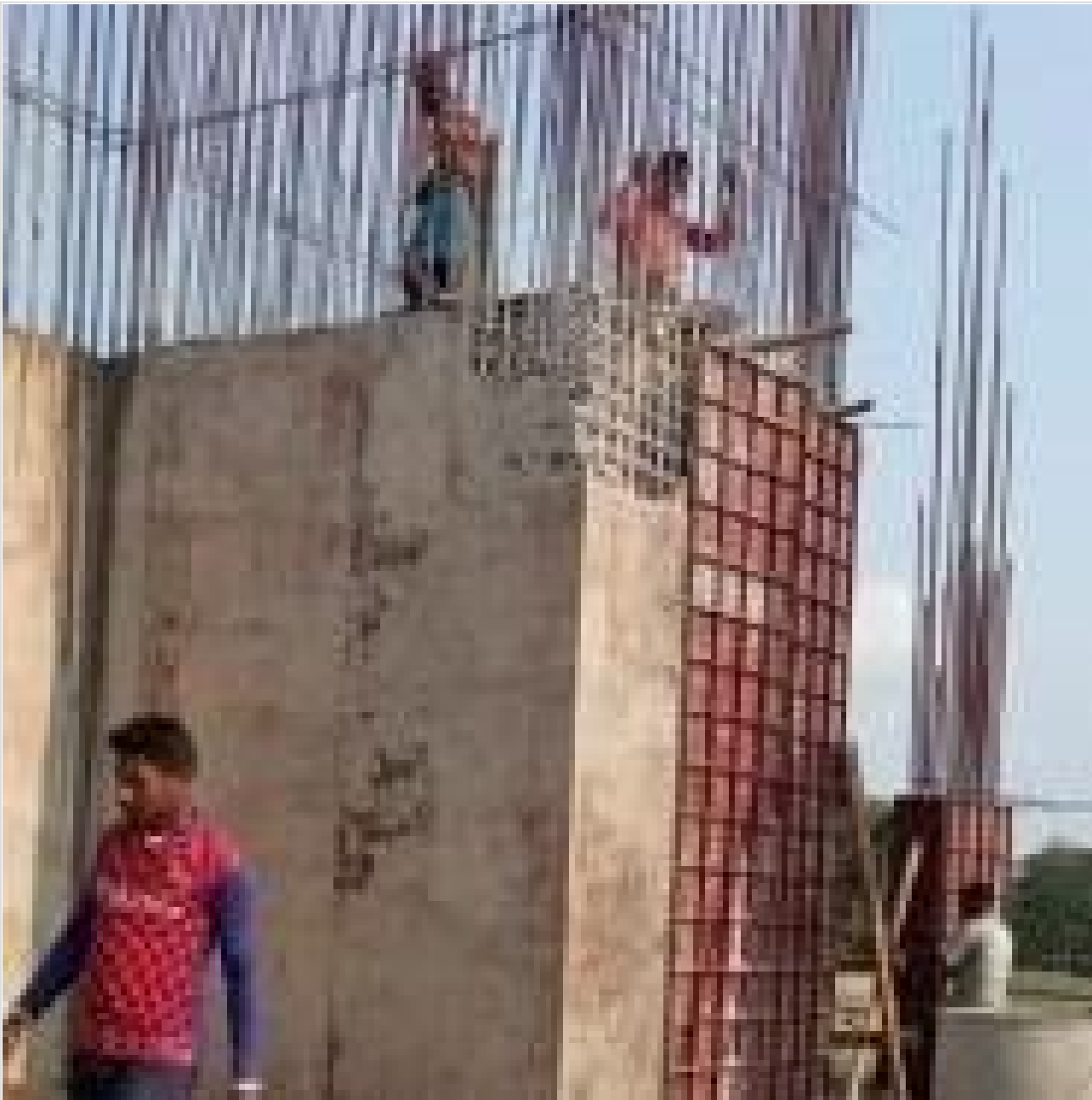
Tower-2-Lift Core Deshuttering on 02-05-21
