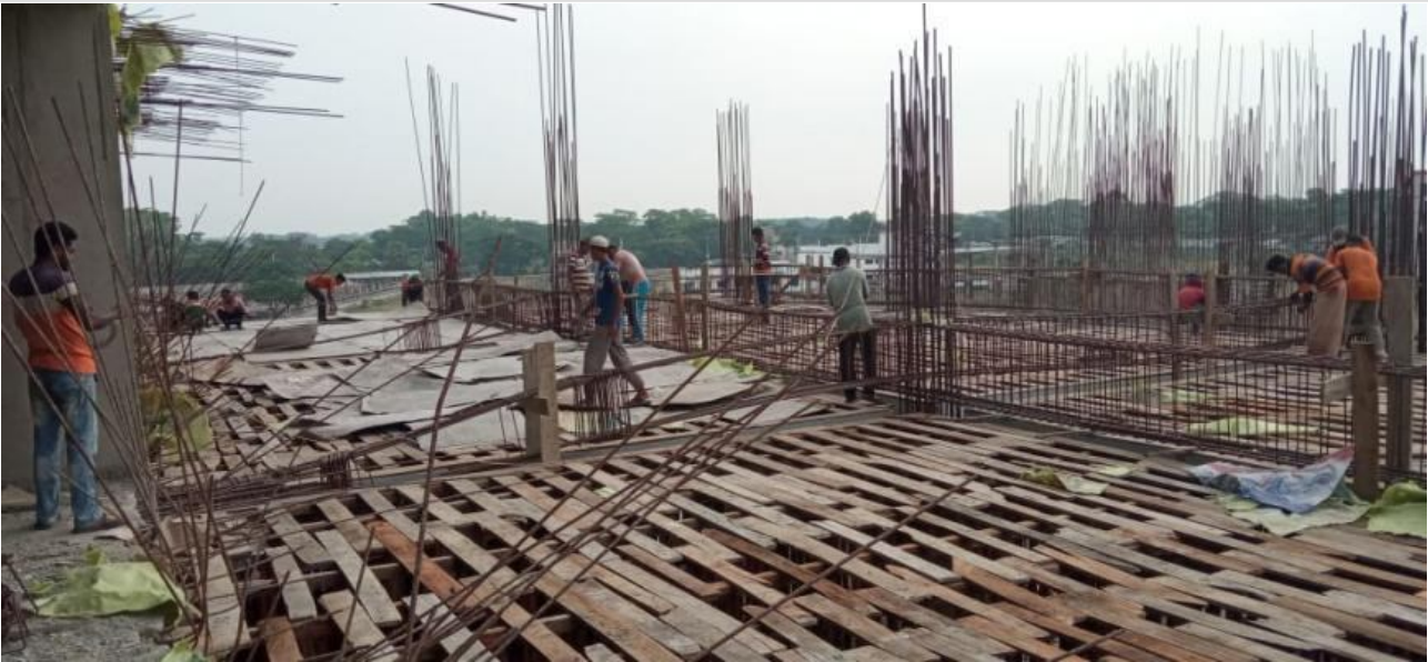
Roof Slab Shuttering on 04-05-21
