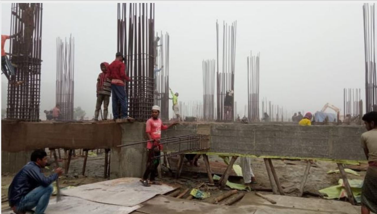
Column Work on 07-12-20
