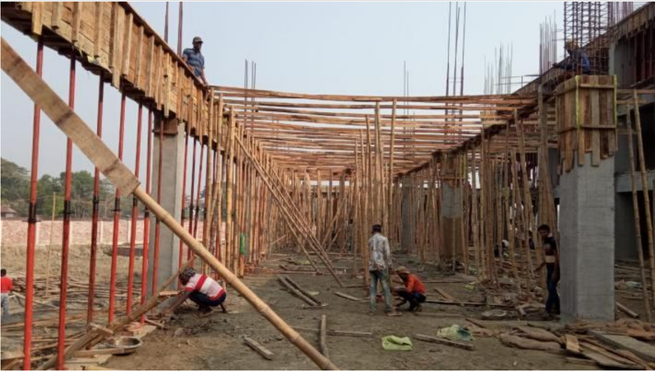
Restaurant Area Slab Shuttering on 23-02-21
