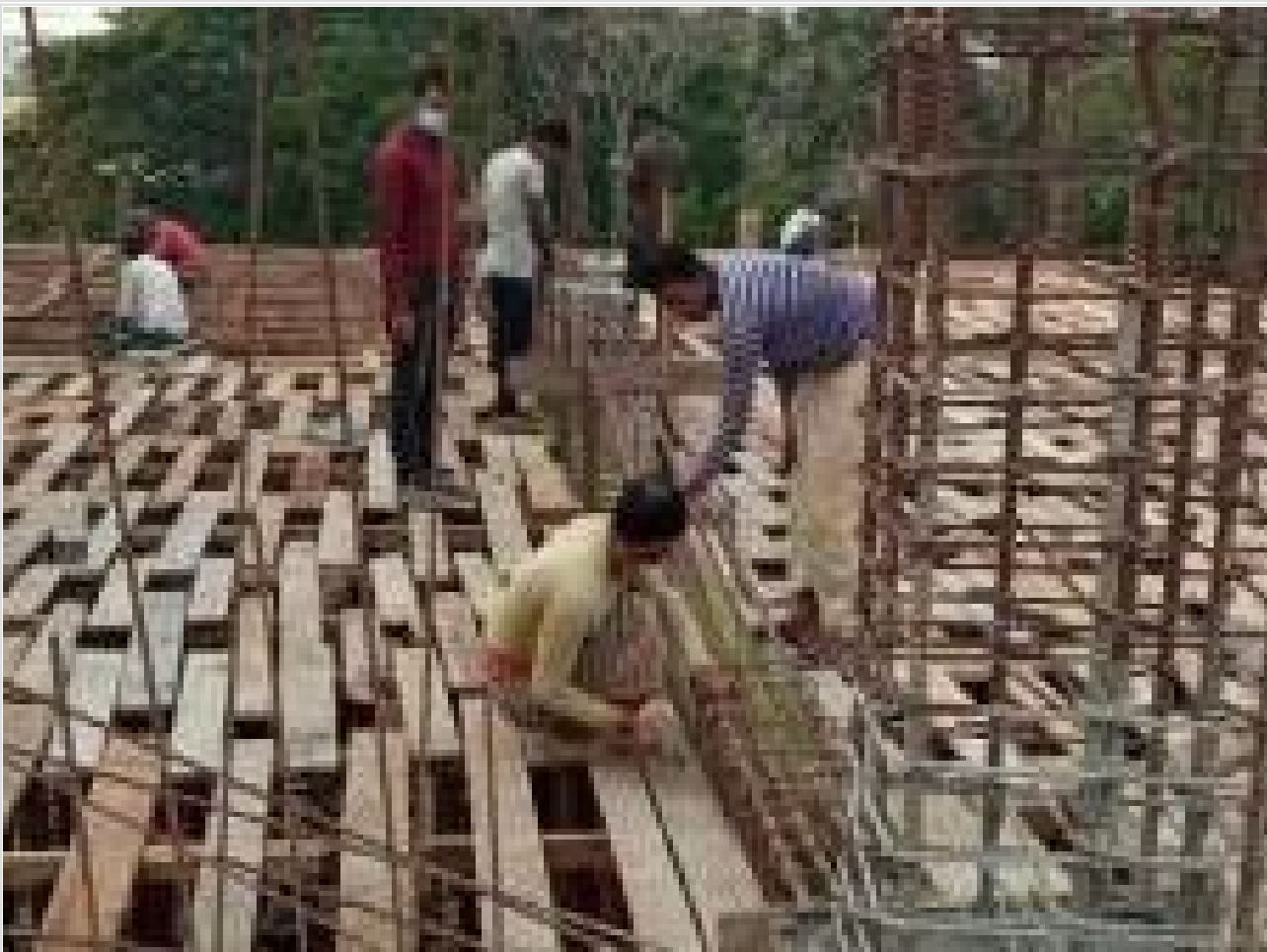
Restaurant CE Double Ht Roof Slab Re bar on 20.03.21
