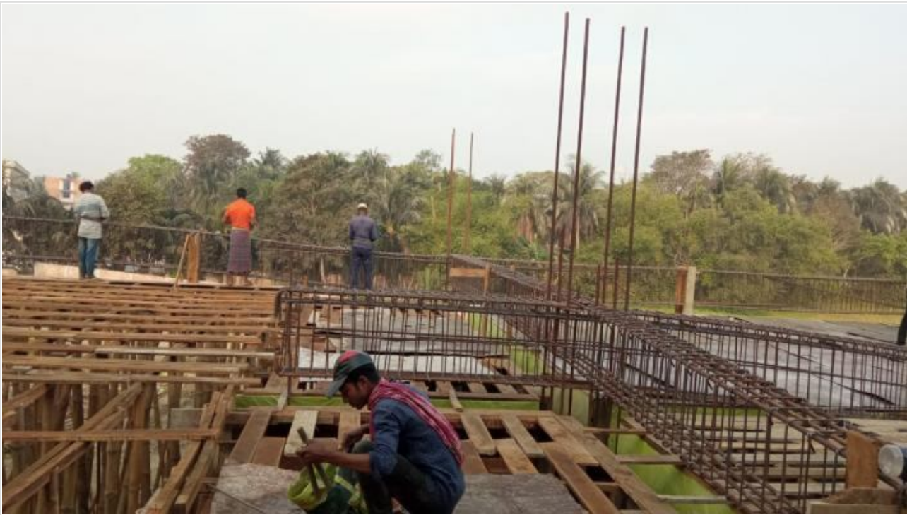
Resturant Area Slab Shuttering on 28-02-21
