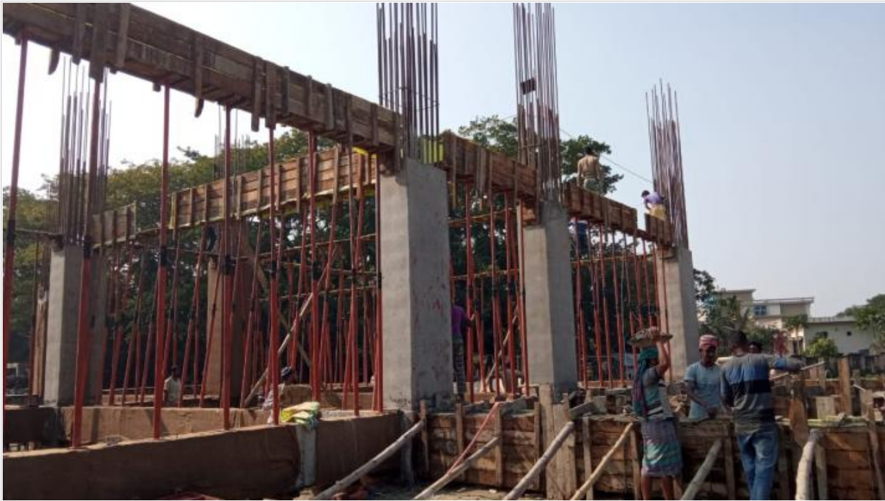
Tower-1-GF Beam Shuttering on 15-12-20
