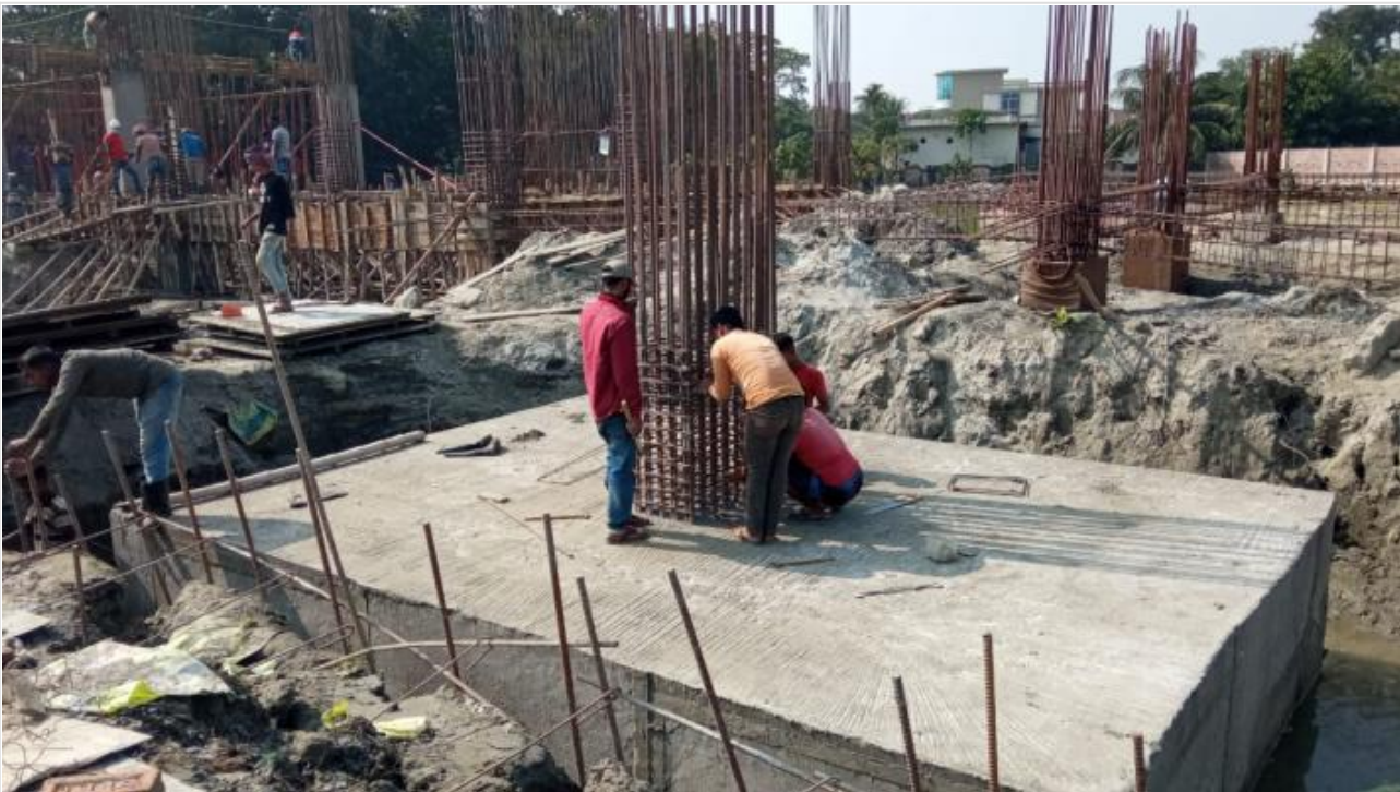
Tower-1-Column Re-bar work on 15-12-20
