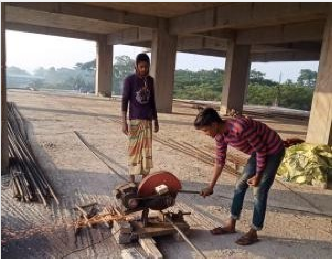
Re-bar Cutting on 08-01-22
