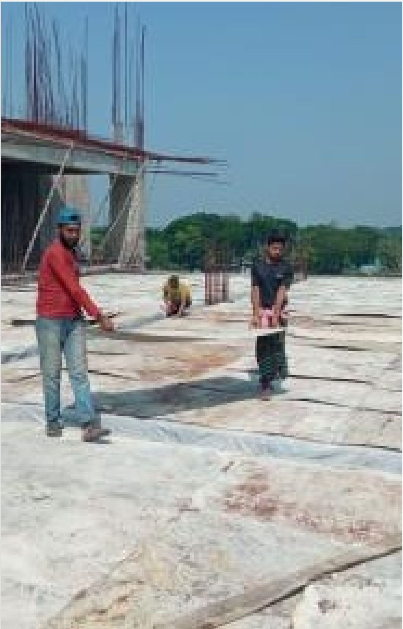
Tower-2-3rd Flr Slab-Plain Sheet laying on 31-10-21
