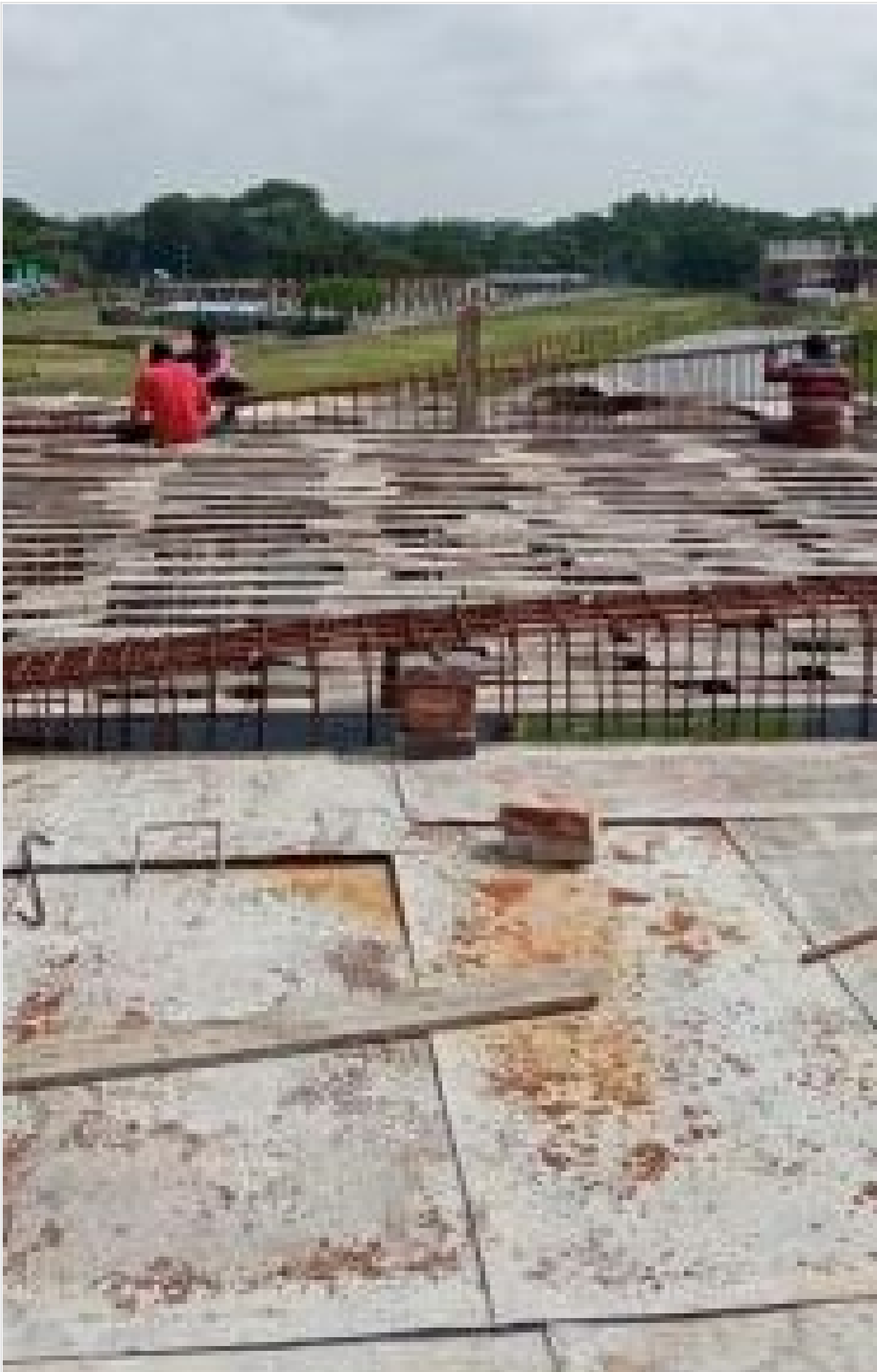
Tower-2-2nd Floor Slab Shuttering on 26-06-21
