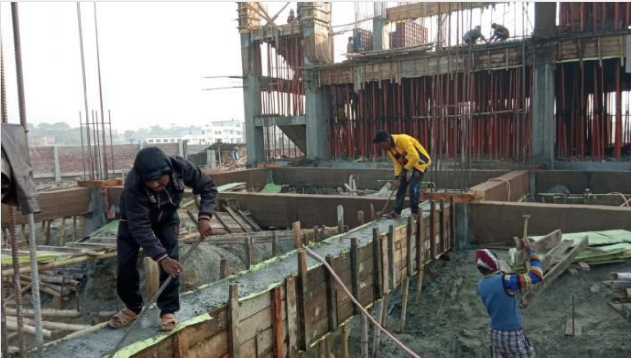
Tower-2-GB Shutter Removing on 05-02-21
