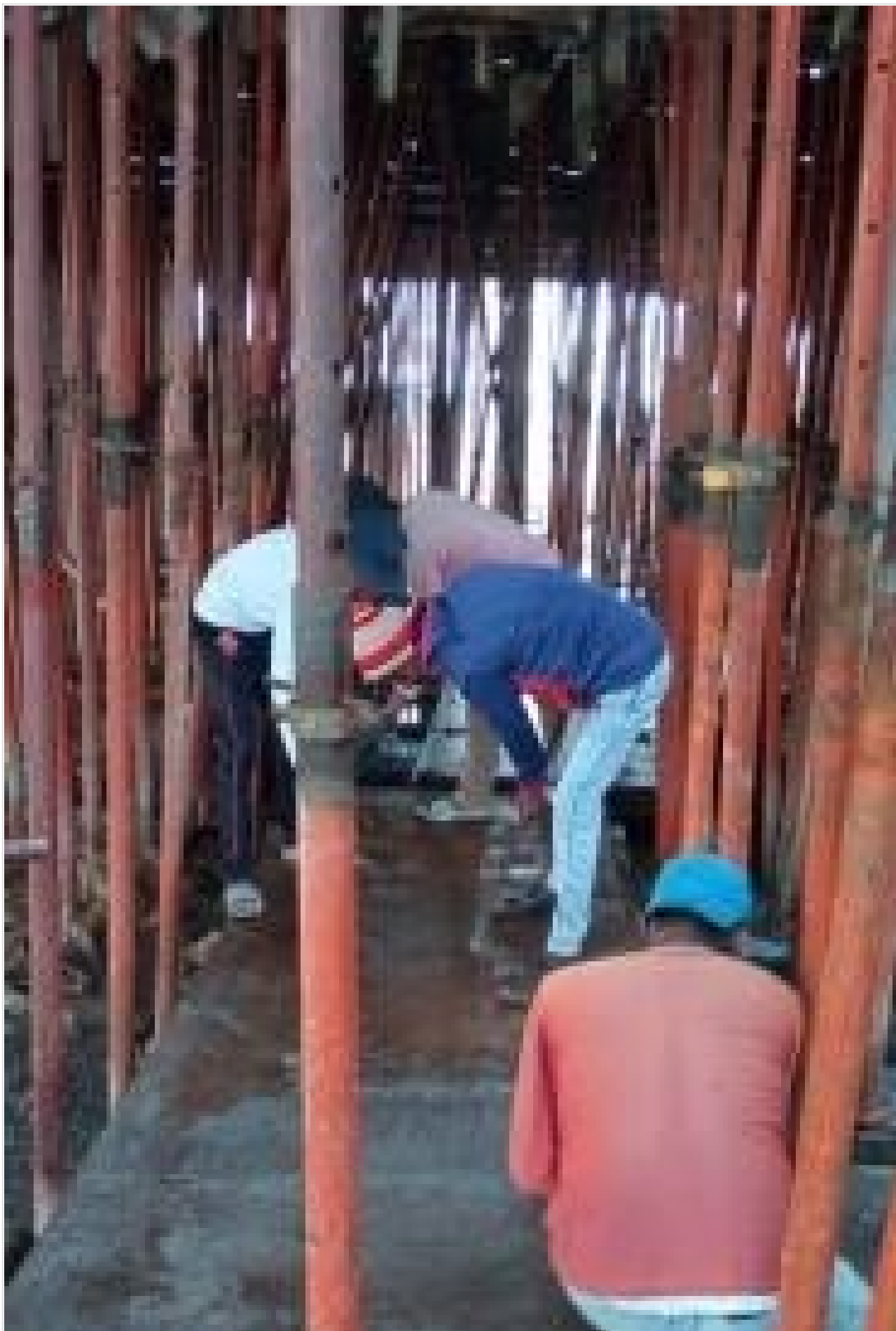
Column/Wall Steel Shutter Cleaning, Oili on 21-02-22
