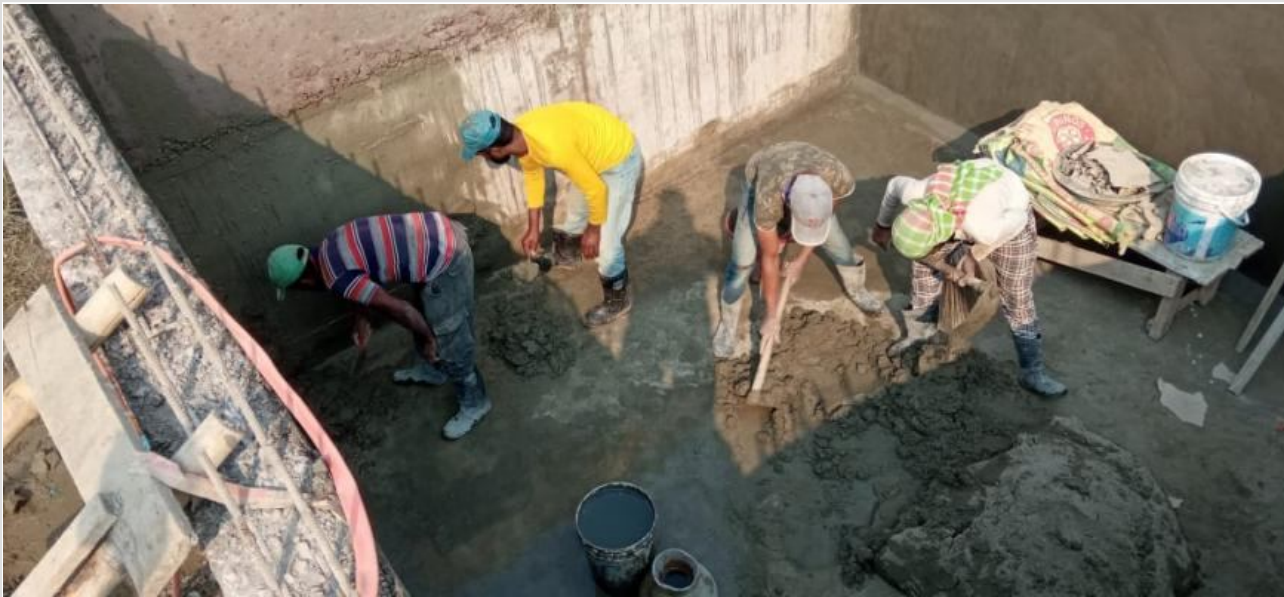
East Septic Tank Plastering on 01-02-22
