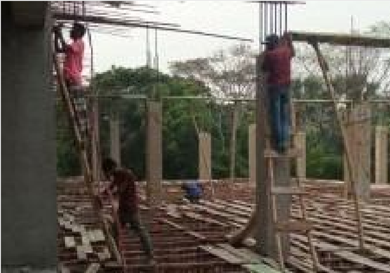
Tower-1-3rd Floor Roof Slab-Beam Shutter on 23-03-21
