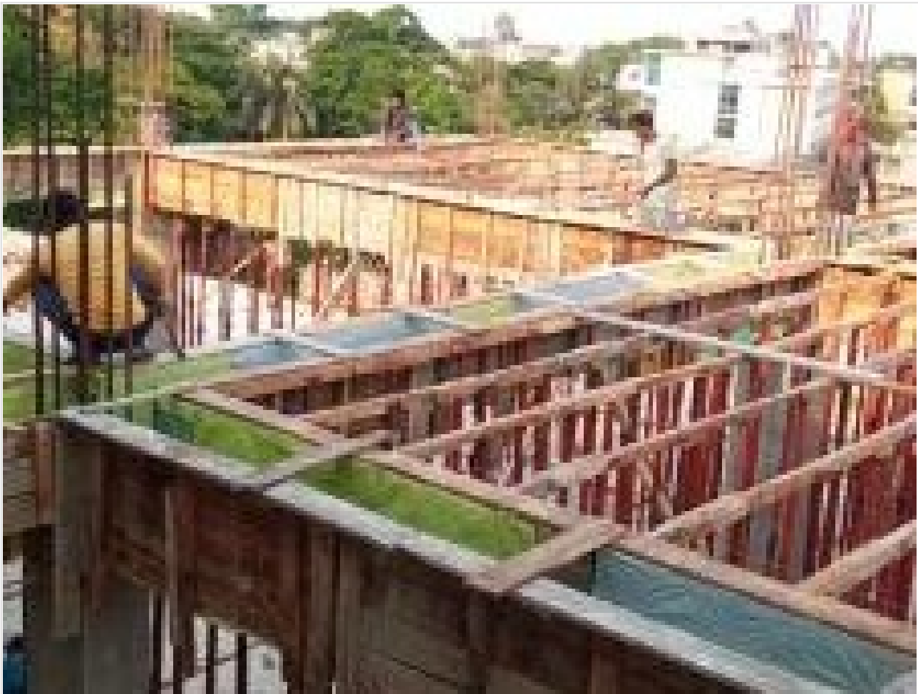
Beam Shuttering on 29-04-21
