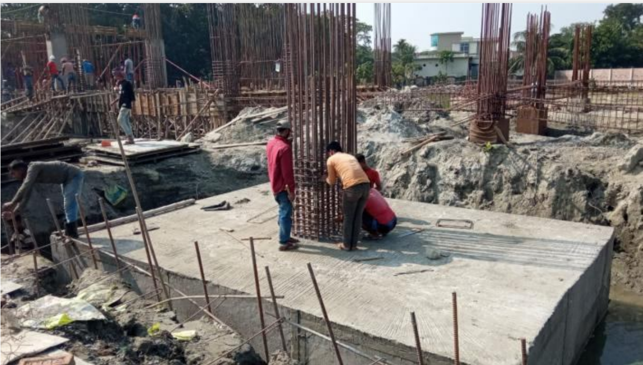
Tower-1-Column Re-bar work on 15-12-20
