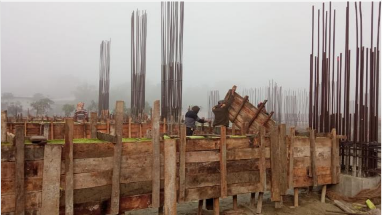
Tower-1-Grade Beam on 04-12-20
