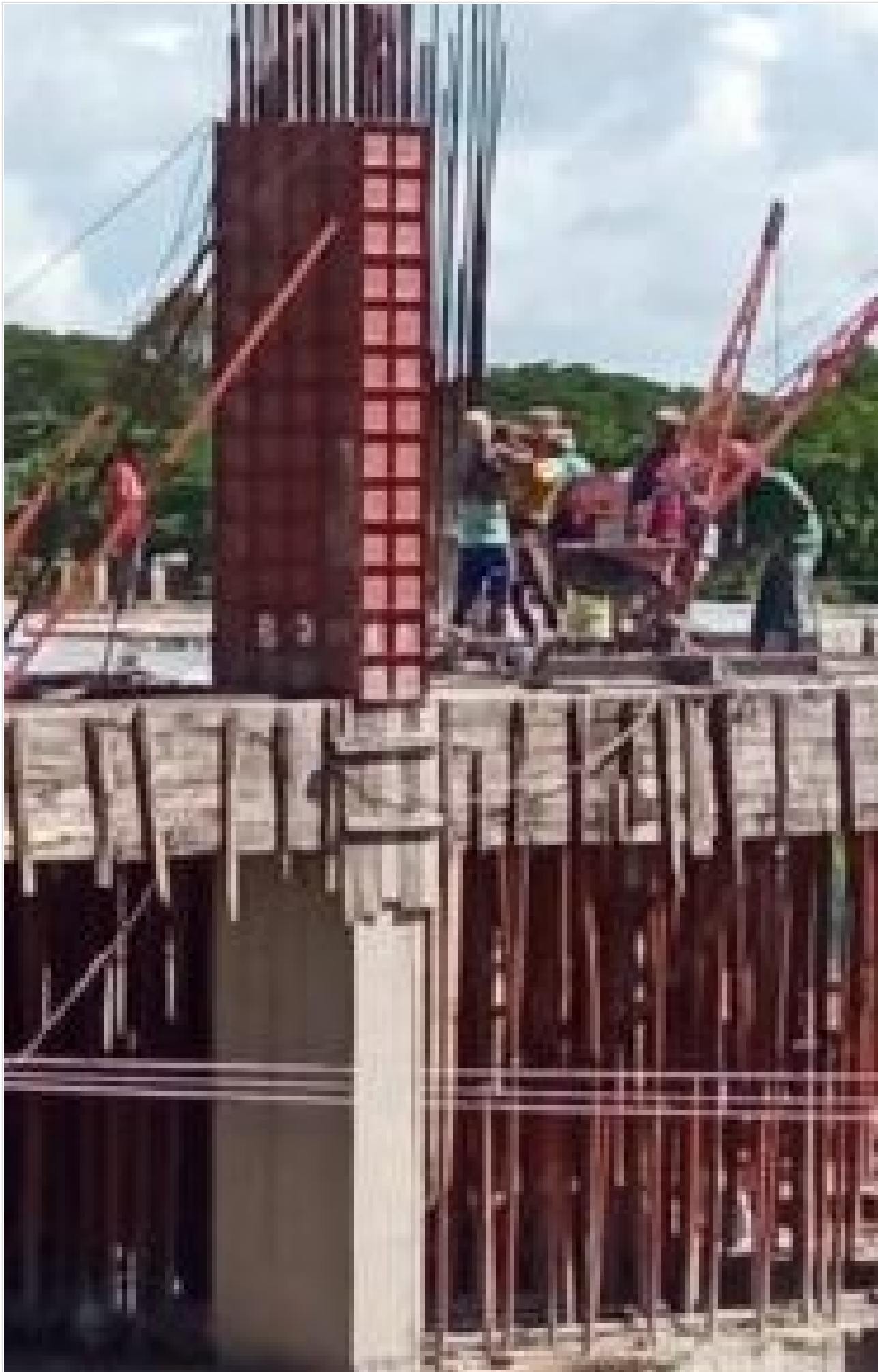
Tower-2-2nd Floor-Column Concreting on 30-09-21
