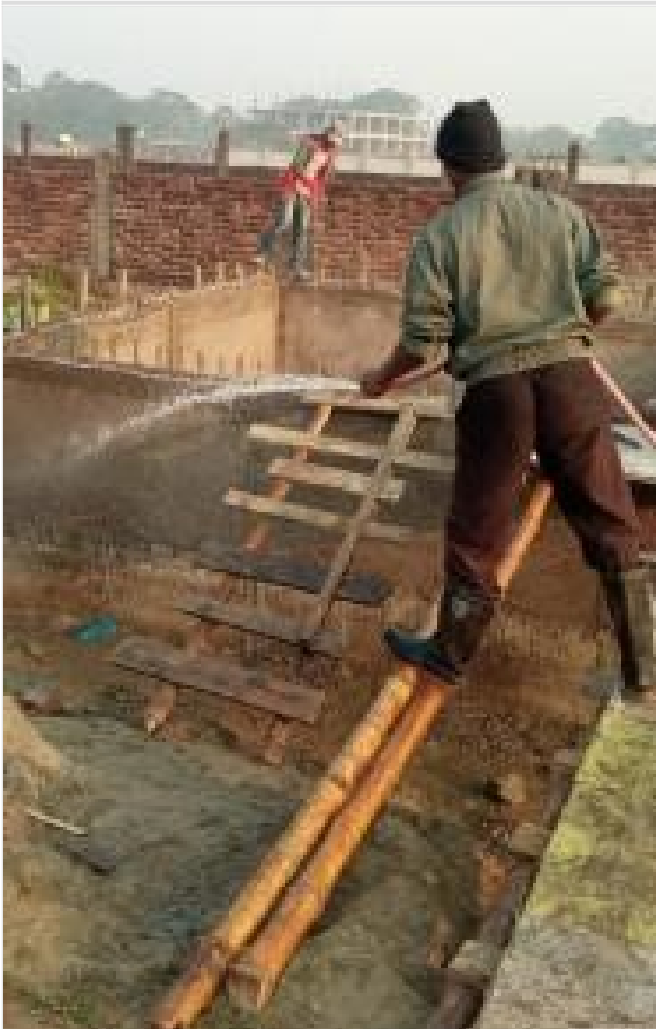
Septic Tank Wall Curing on 31-01-22
