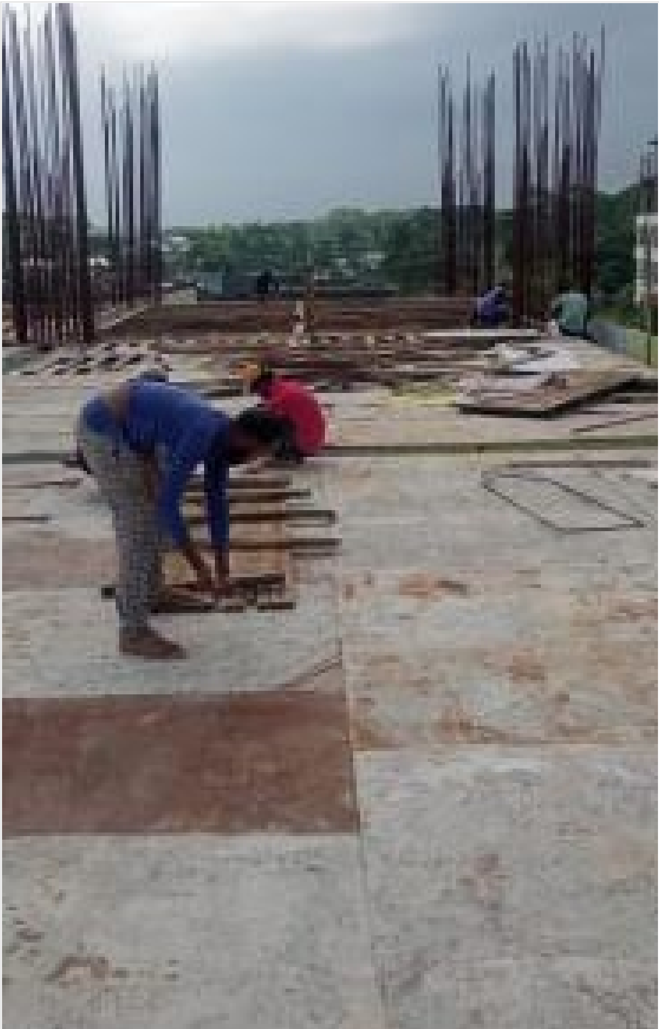
Tower-2-2nd Floor Slab Shuttering on 22-06-21
