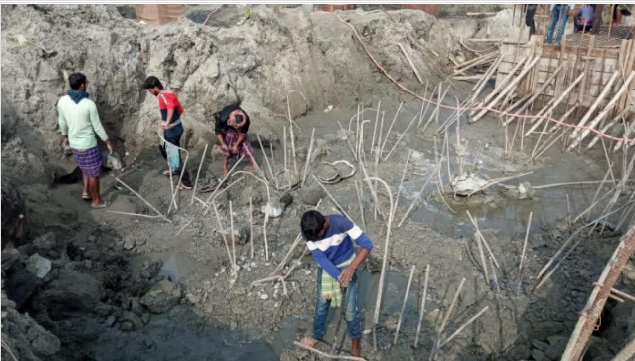
Tower-1-Pile Cap Re-bar Fabrication on 12-12-20
