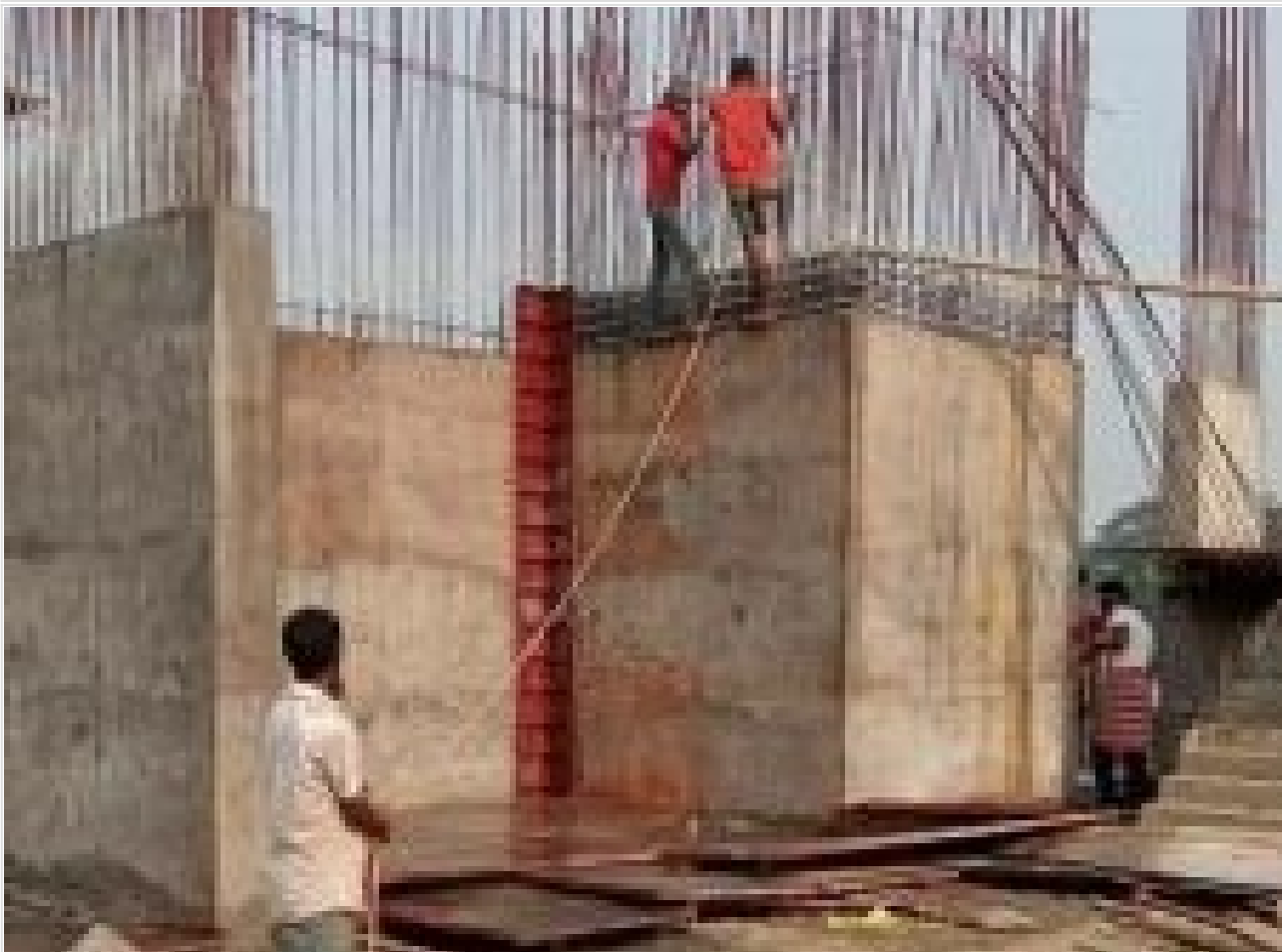
Tower-2: Lift Wall De-shuttering Work on 25-03-21
