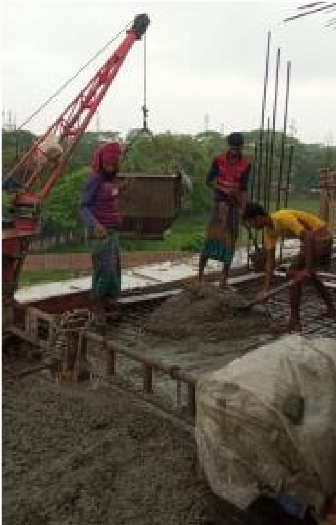
Restaurant-3rd Floor Slab Concreting on 16-06-21
