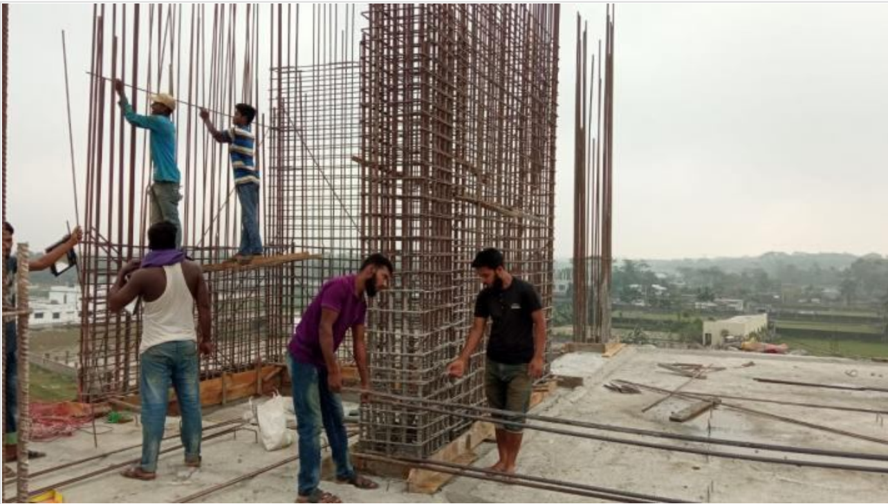
Tower-1-3rd Floor Lift Core Re-bar Work on 02-03-21
