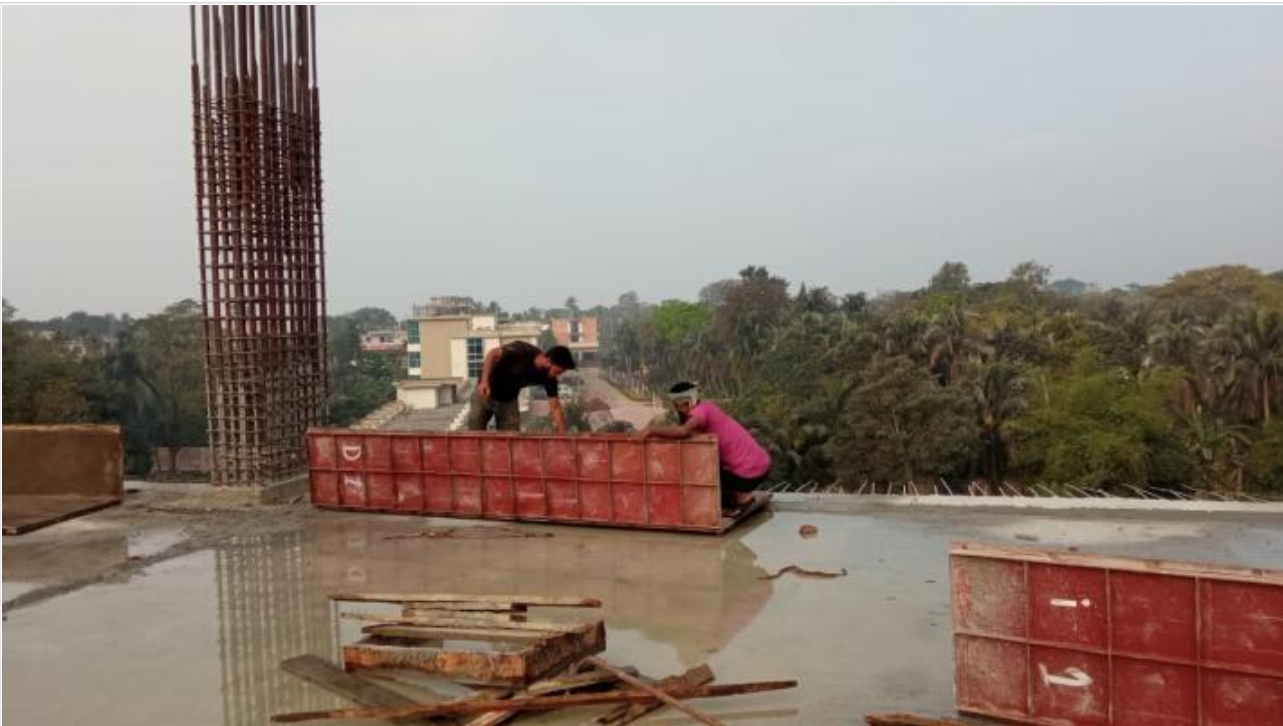
Tower-1-3rd Floor Column Shuttering on 28-02-21
