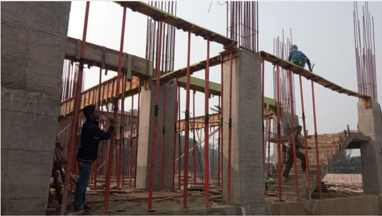
Tower-1-1st Floor Roof Beam Shuttering on 18-01-21
