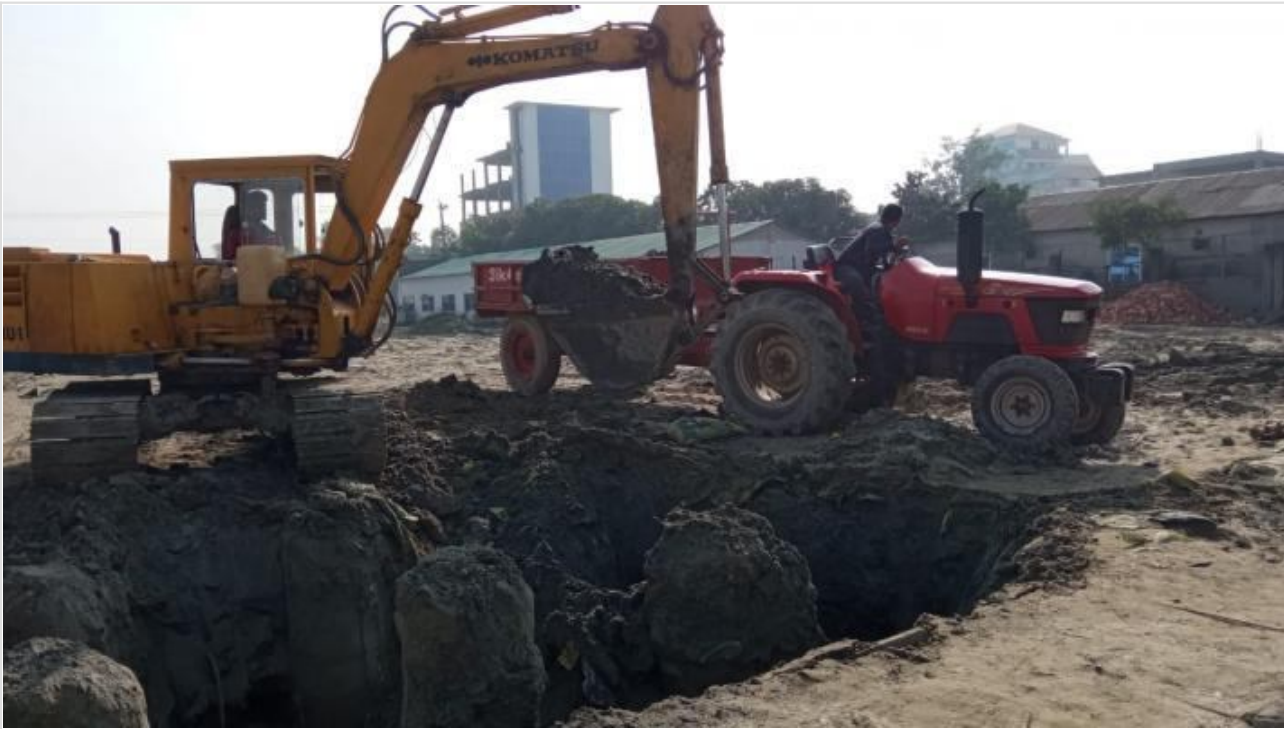
Tower-2-Excavation for Pile Head Breakin on 24-12-20
