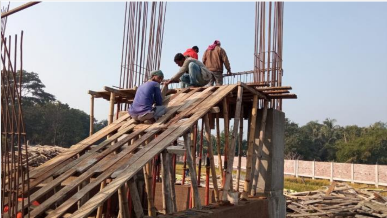
Tower-1-GF Stair Shuttering on 27-12-20
