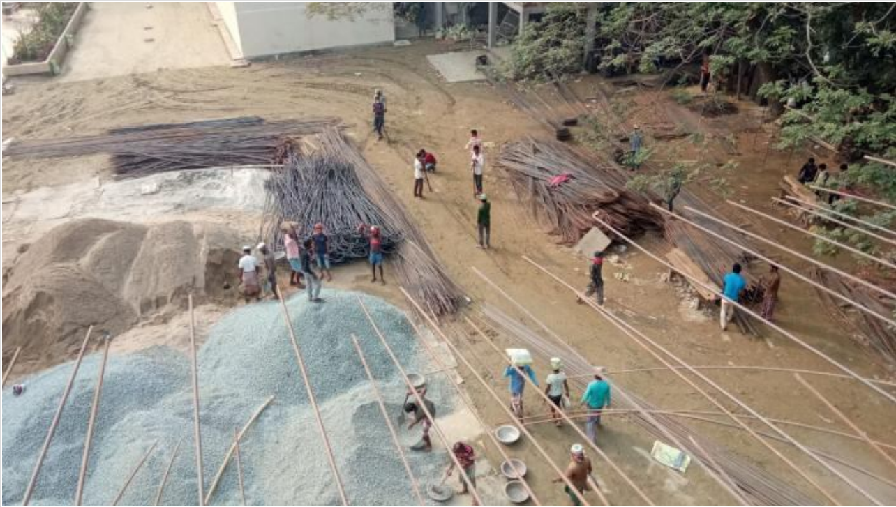
Tower-1-1st Floor Roof Slab Concreting on 11-01-21
