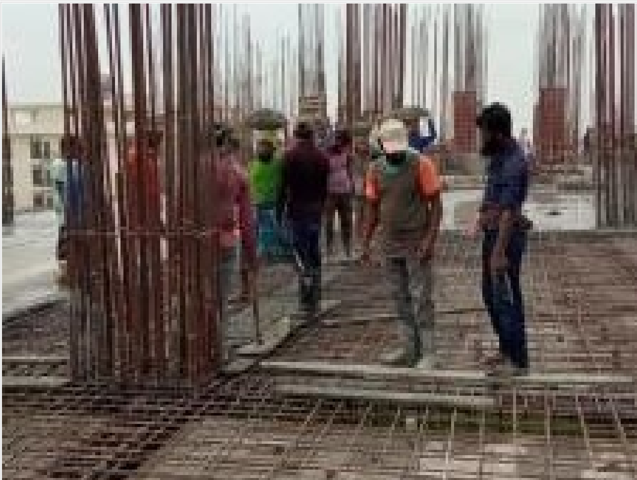
Tower-1-3rd Floor Roof Slab(B-E/6-7)Conc on 31-03-21
