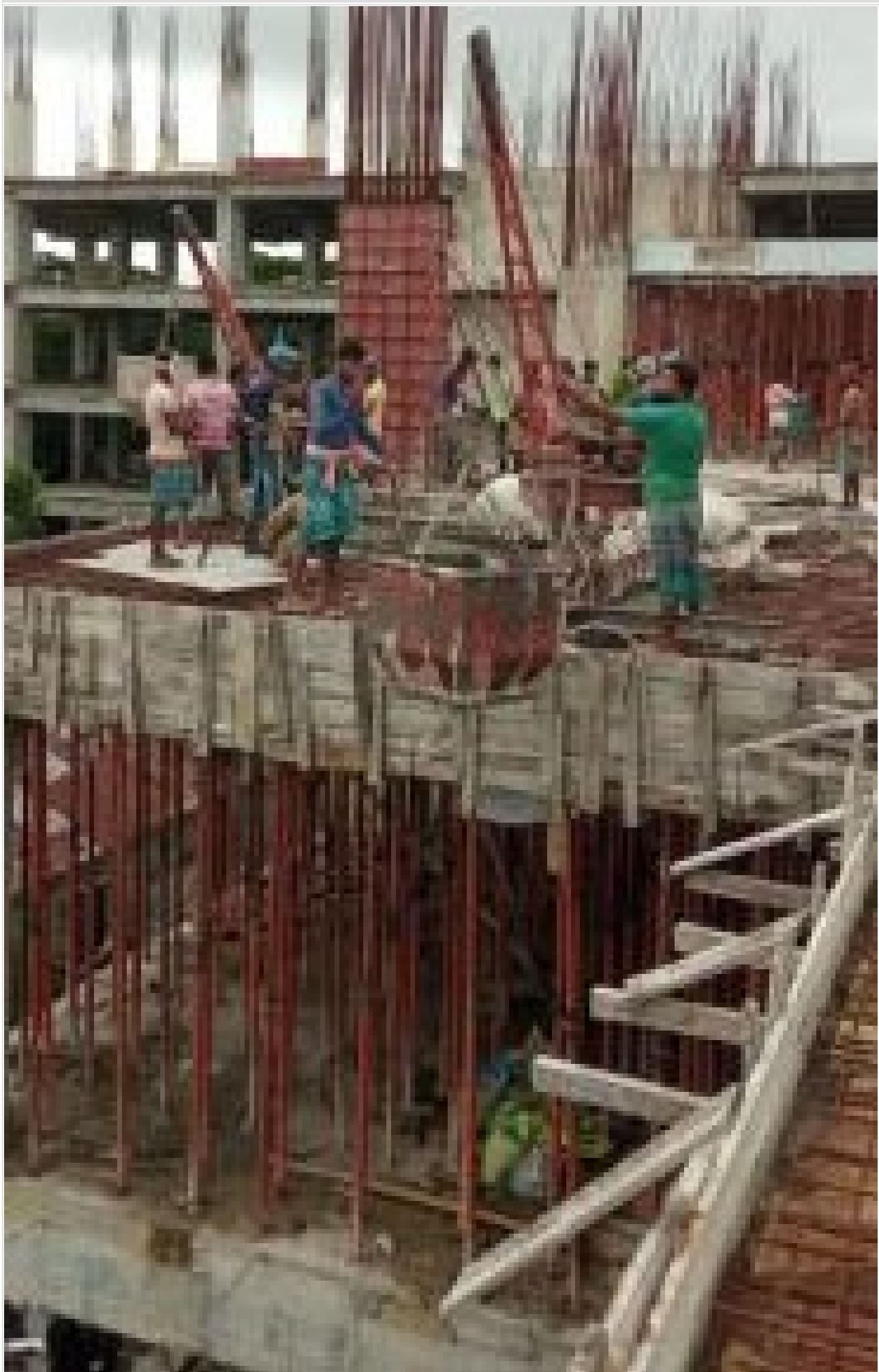
Tower-2:2nd flr double height slab concr on 26-09-21
