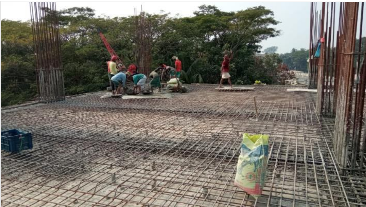
Tower-1-1st Floor Roof Slab 3600 sft Co on 11-01-21
