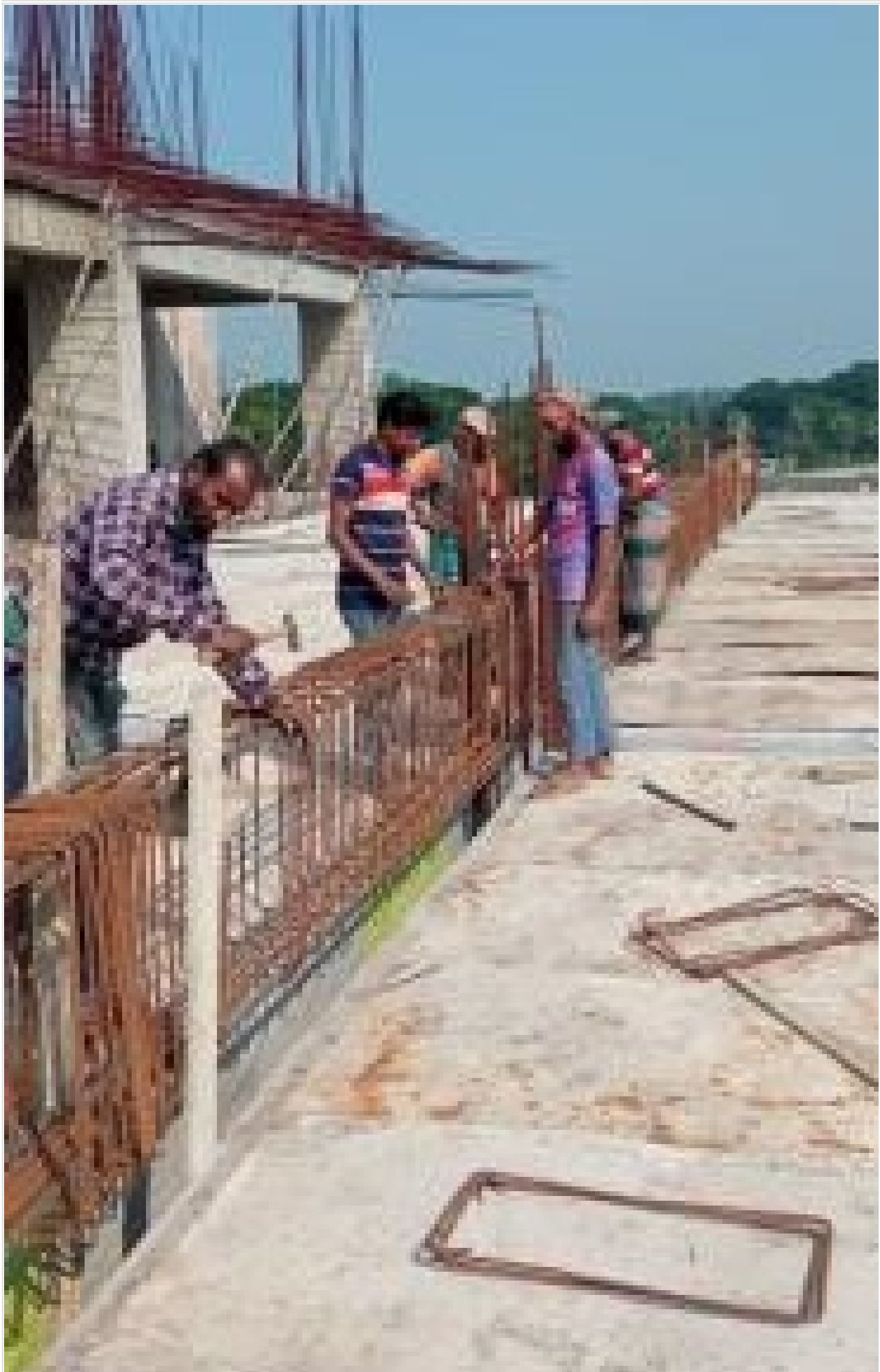
Tower-2-3rd Floor Beam Re-bar work on 01-11-21
