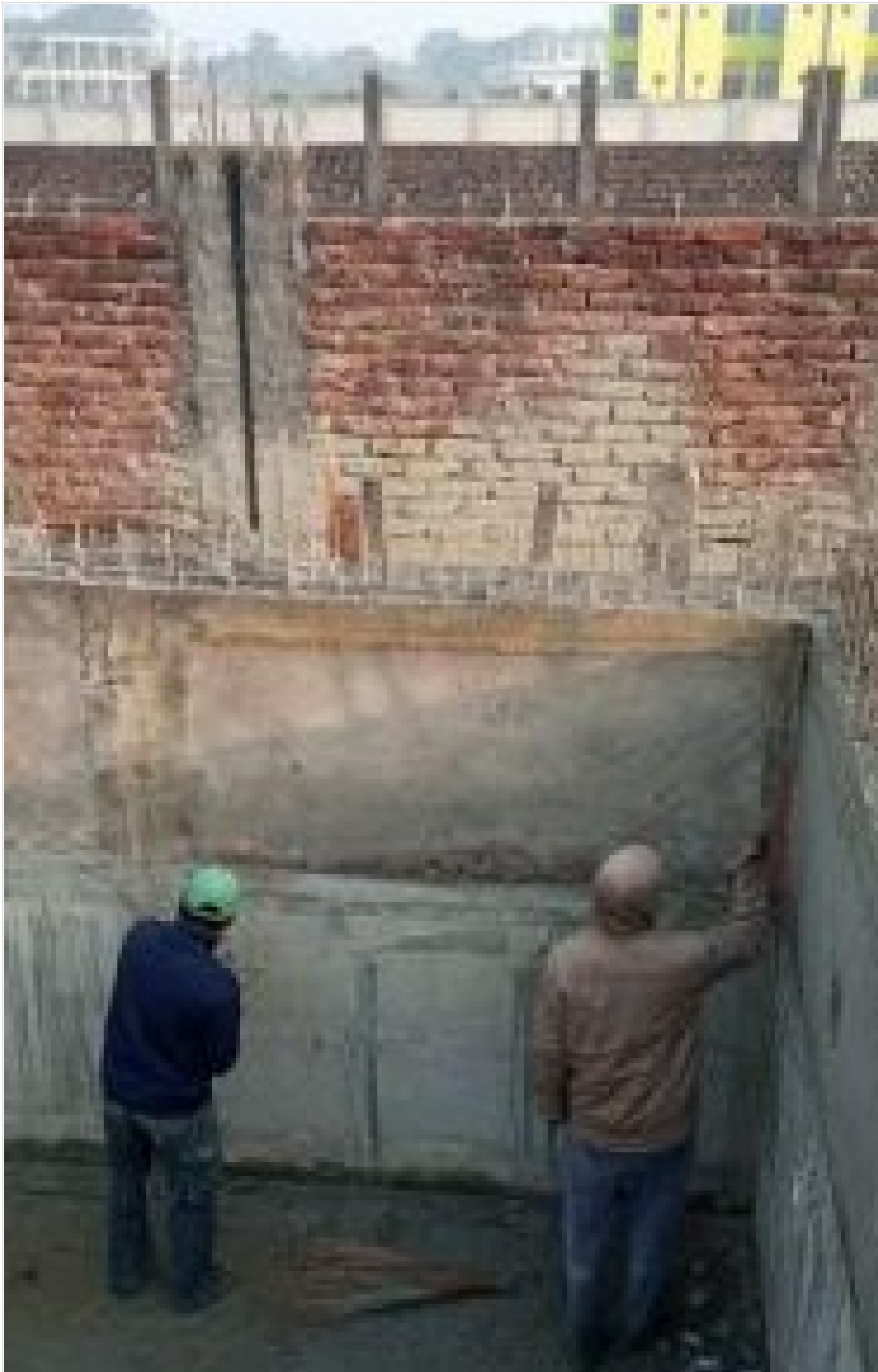
Septic Tank Wall Plastering on 31-01-22
