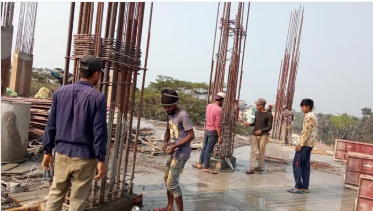
Tower-1-3rd Floor Column Re-bar Work on 23-02-21
