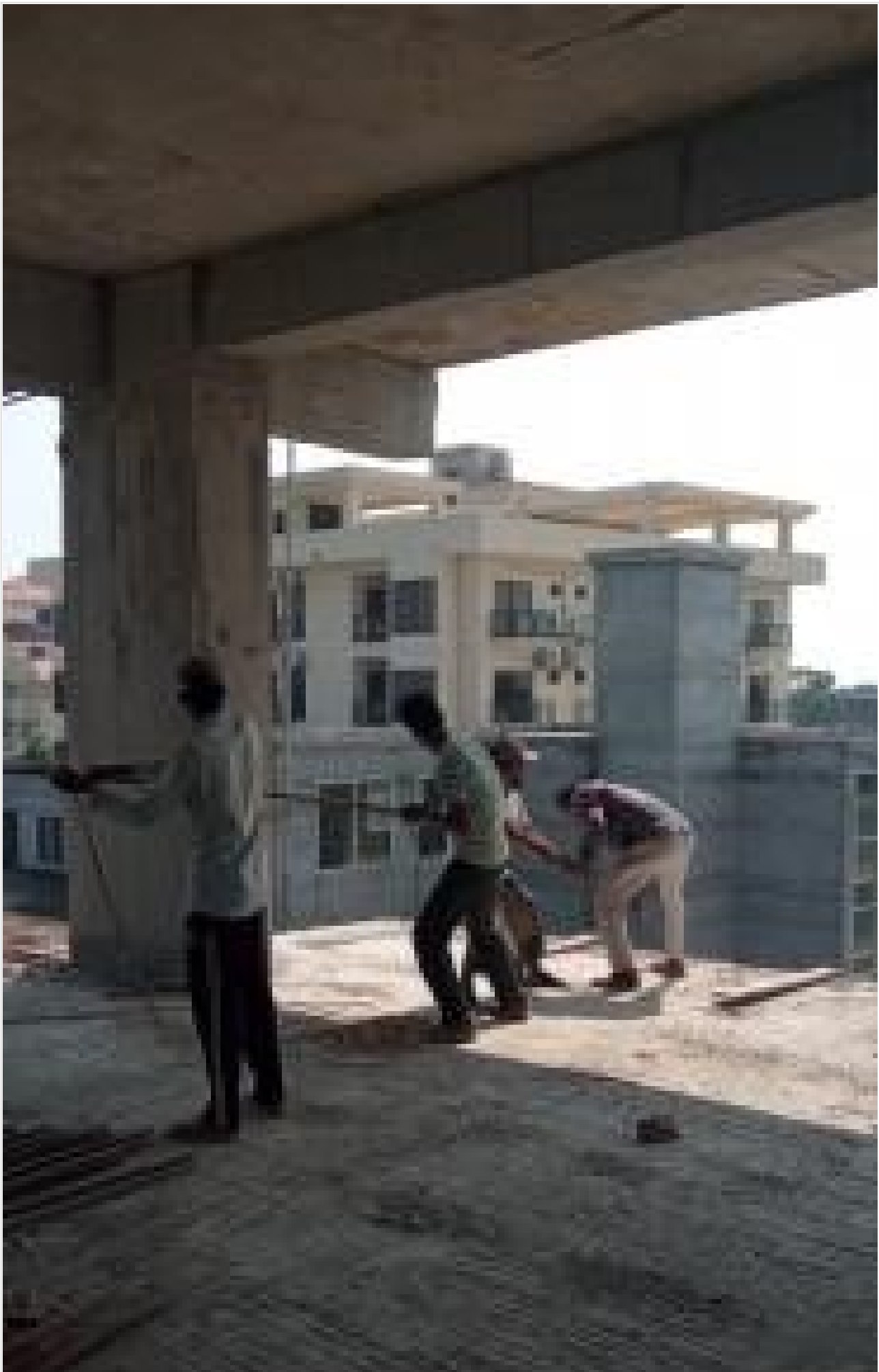
Tower-2-3rd Flor Slab-Rod Lifting on 31-10-21
