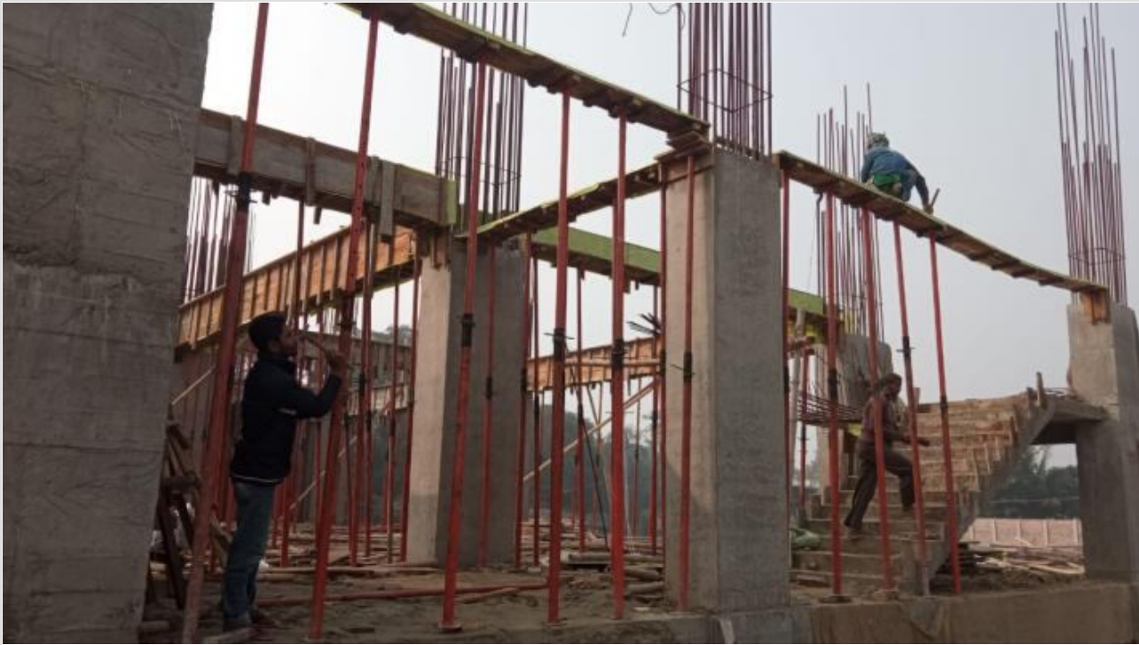
Tower-1-1st Floor Roof Beam Shuttering on 18-01-21
