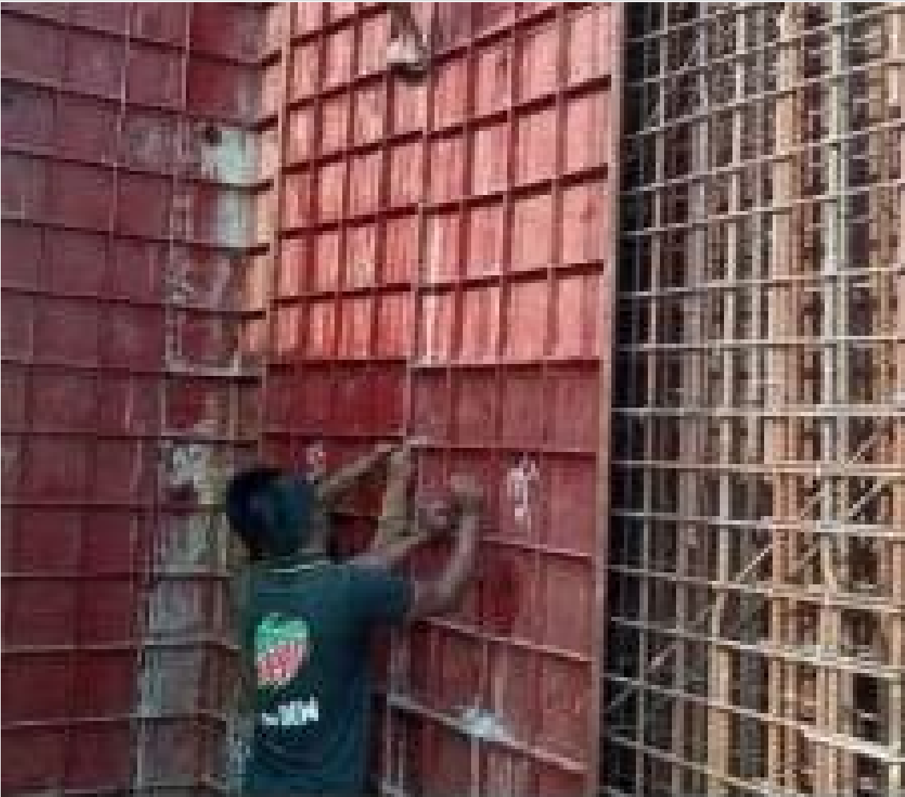
Lift Core Wall Shuttering on 26-04-21
