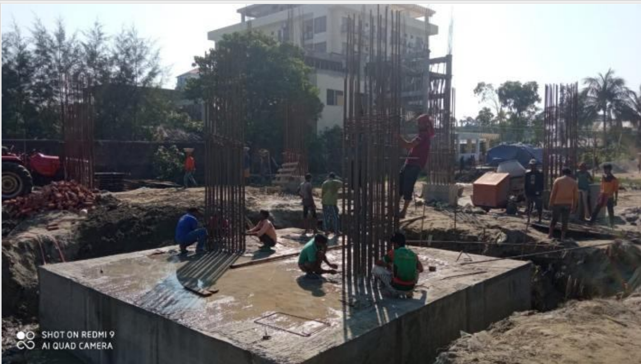
Tower-1 Pile Cap on 30-11-20
