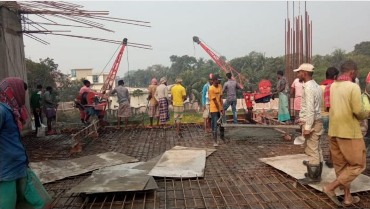
Tower-1-GF Roof Slab Concreting on 16-01-21
